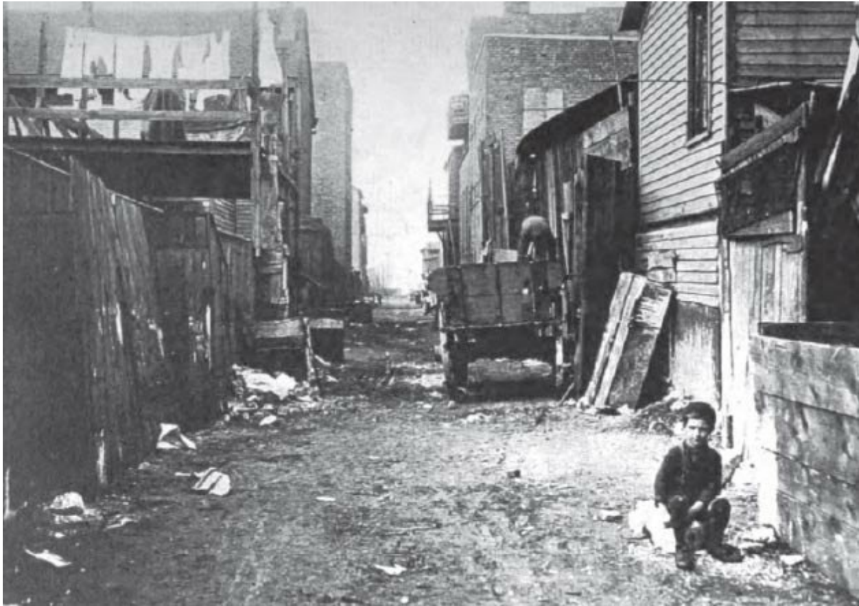
Photo 1.4: The general insanitary conditions which surround the houses on both sides of the alley. The first house on the right is a small dilapidated frame house. Beyond it are three larger tenements. The outbuildings at the left are all dilapidated, and contain privies which are in a foul condition. There are not enough garbage boxes to supply the needs, and the ones provided are so seldom cleaned that the families dump their slops and garbage in the alley. (1901)
