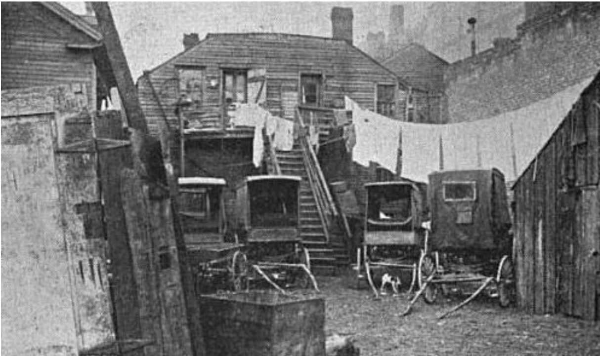
Photo 1.2: Jefferson Street. The shed barn at right contains three horses. The barn next in view contains six horses and two goats. The house in the center of the picture is full of Italian families and presents no redeeming feature. On the left are other tenements full of families. (1911)
