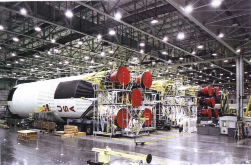
ABOVE The Saturn V first stages, S-1C-10, S-1C-11, and S-1C-9, are in the horizontal assembly area, ready for the installation of the engines (five F-1 engines) at Michoud Assembly Facility (MAF). (NASA)
