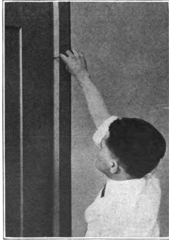
FIG. 448. MARKING DOOR AND FRAME FOR HINGE LOCATION.
