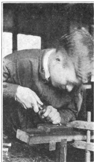
FIG. 346. POSITION FOR HEAVY WORK.
