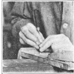
FIG. 369. METHOD OF HOLDING TOOL FOR VERY DELICATE MODELING.
