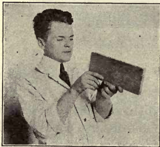
Fig. 49. Sighting for Straightness
