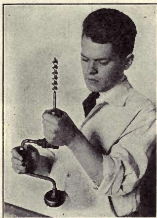
Fig. 65. Inserting a Bit
