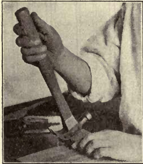
Fig. 102. Withdrawing Nails
