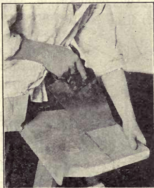
Fig. 30. Position for Final Crosscutting
