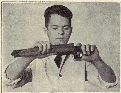
Fig. 23. Setting Marking Gage
