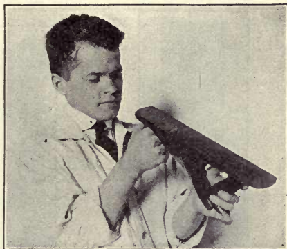
Fig. 42. Sighting a Plane-iron
