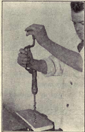
Fig. 70. Vertical Boring; Second Position
