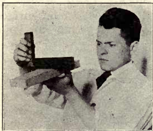
Fig. 56. First Test for Surface Trueness
