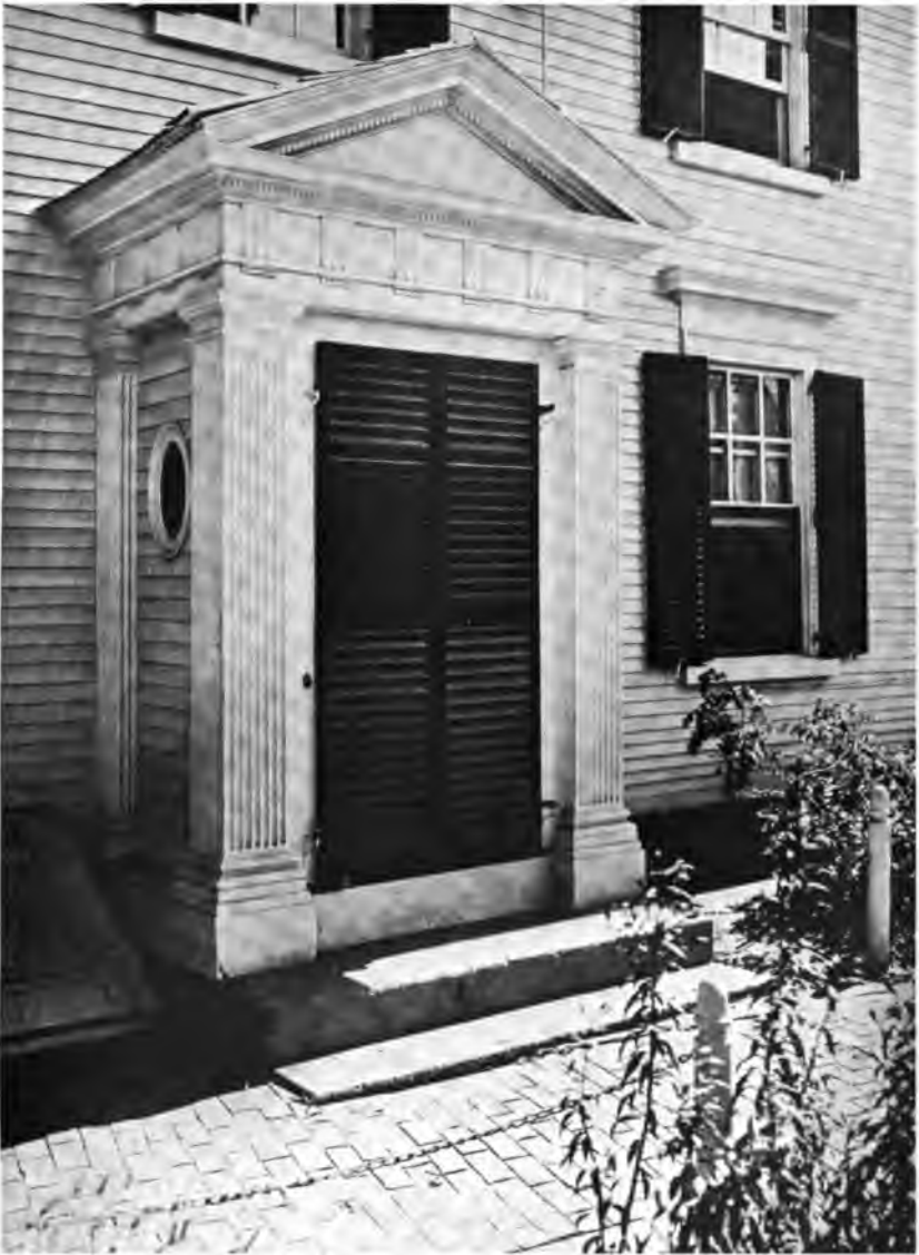
PLATE XCII.—Enclosed Side Porch, Pierce-Johonnot-Nichols House.
