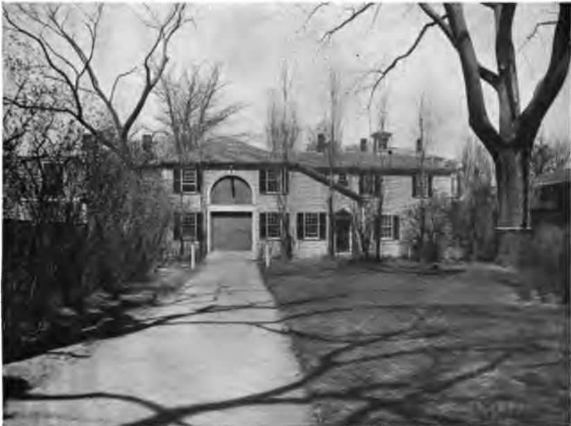
PLATE XVIII.—Cornice, Eaves, and Balustraded Roof, Peabody-Silsbee House; Peabody-Silsbee Barn.
