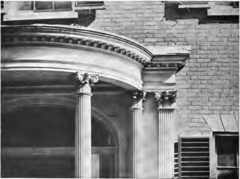
PLATE XXV.—Tucker-Rice House, erected in 1800; Detail of Porch.
