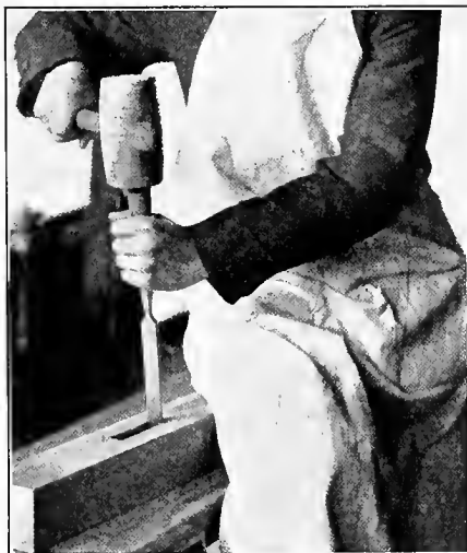
FIG. 149. — METHOD OF GRASPING THE CHISEL FOR MORTISING LARGE WORK.
