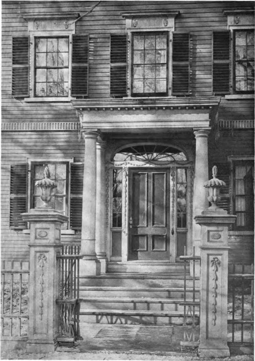
PLATE LXXVIII.—Cook-Oliver Entrance, showing Window Heads.
