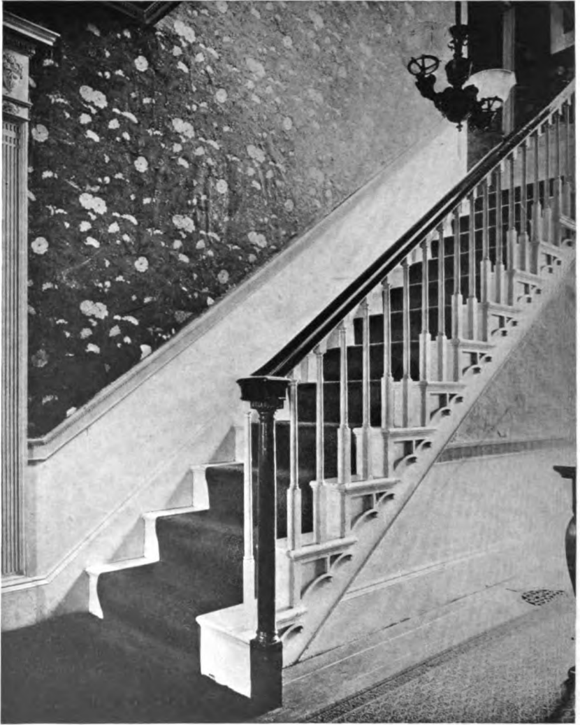
PLATE LXXIX.—Stairway, Cook-Oliver House.
