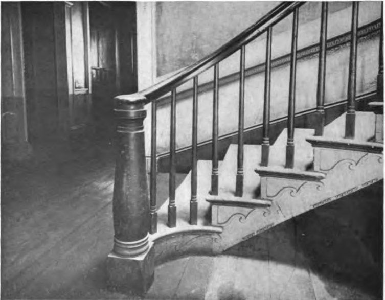
PLATE XLVII.—Stairway at Second Floor Level, Derby-Crowninshield-Rogers House; Detail of Newel and Stair Ends.
