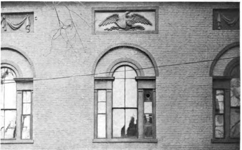
PLATE CXXIII.—Hamilton Hall, erected in 1805; Detail of the Second Floor Windows and Sculptured Panels.
