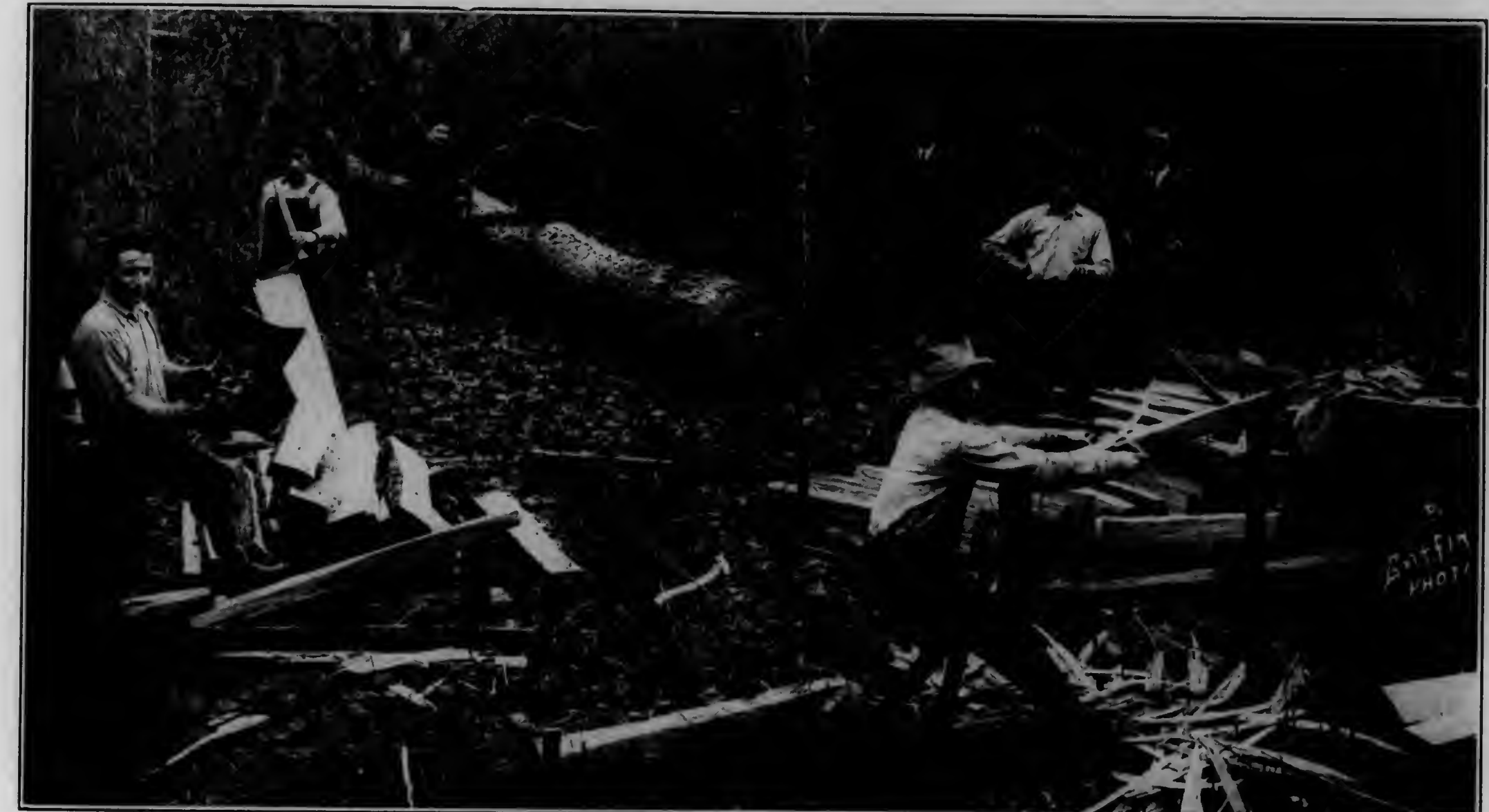
STAVE CAMP IN NORTHERN LOUISIANA Photograph showing the several processes through which the white oak passes in its process of becoming a "French claret" stave. Photo taken for the Foxley Stave and Lumber Company, of New Orleans, F. J. Foxley, President.
