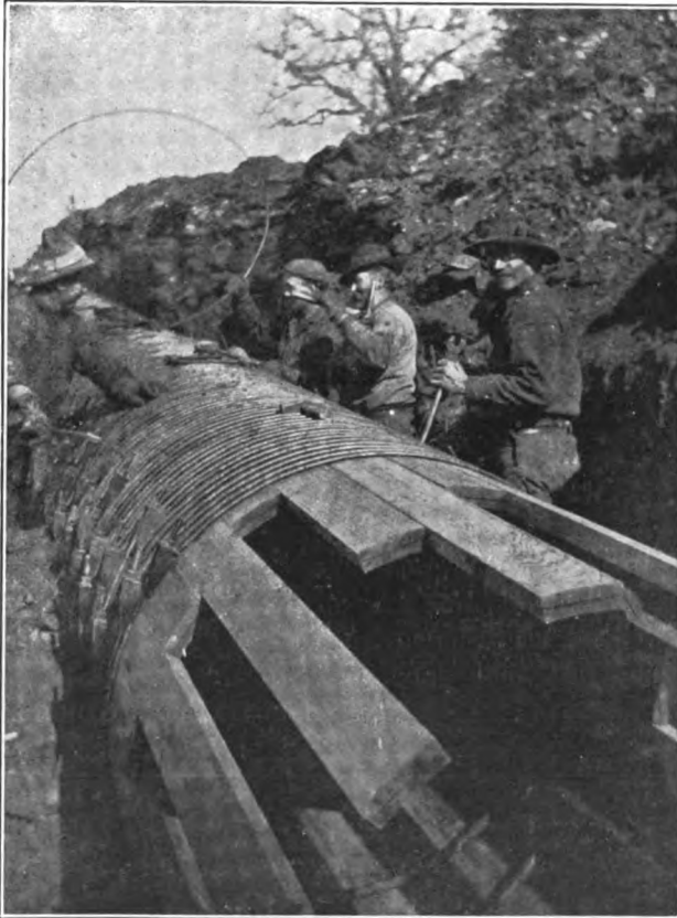
Fig. 8. Finishing Wooden Pipe.
