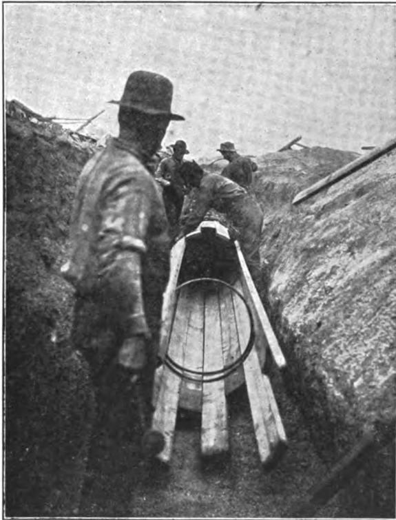
Fig. 6. Laying Wooden Pipe.
