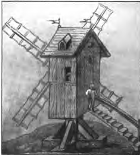
Post Mill as Bolted to the Ground : Sixteenth Century.
