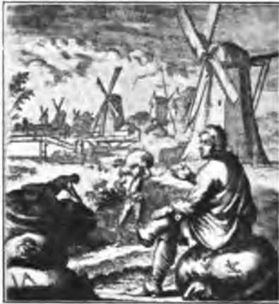
German Post and Tower mills : Seventeenth Century.
