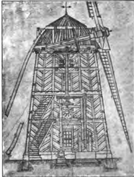
Modern Tower : Cap and Beam.
