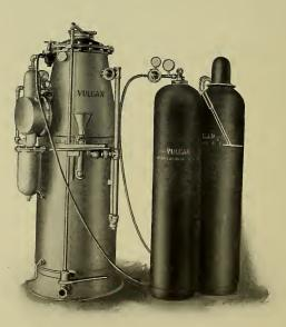
Showing a complete oxy-acetylene plant made in various sizes, all ready for work.
