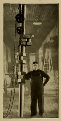
SAME CRANK SHAFT WELDED. Good as new and working every day.
