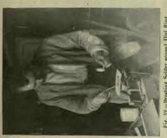
Fig. 39.-Brushing Solder around Dial Ring
