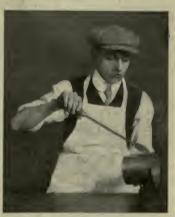
Fig. 22.—Soldering Can Externally
