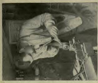
Fig. 36.-Soldering Lug to Lamp Bottom
