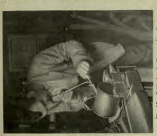
Fig. 35.—Soldering Lading-can handle
