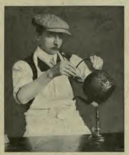
Fig. 41.—Re-soldering Kettle Spout
