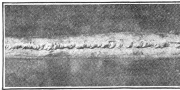
Fig. 45. Appearance of Poor Weld in Light Sheet Steel
