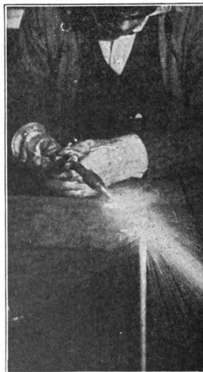
Fig. 81. Beveling End of Heavy Square Shaft for Welding
