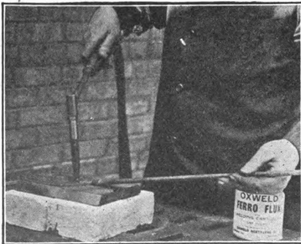
Fig. 75. Dirt May Be Scraped off by Means of the Welding Rod
