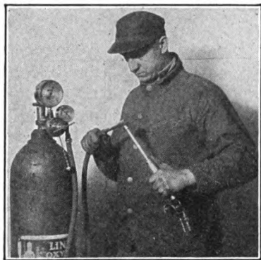
Fig. 16. Cleaning Blowpipe by Means of Oxygen under Pressure
