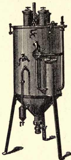
Figure 22.—Generator for Using the Carbide in Compressed Cakes
