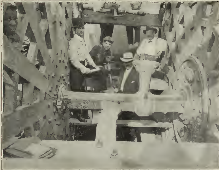
Finished Weld on Stern Wheel Shaft of S. S. "Betsy Ann" Before Removing Metal Left in Gate and Riser.
