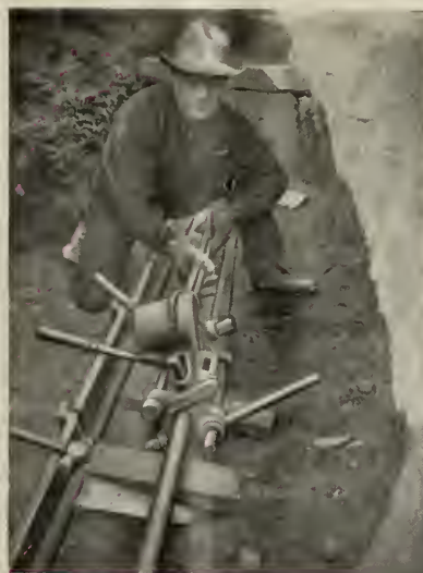
FIG. 4.—WELDING 1¼-INCH PIPE.
