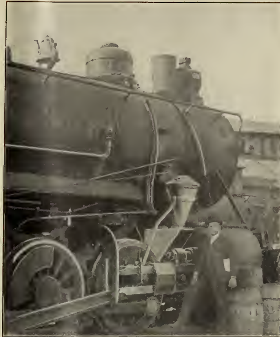
FRAME READY FOR WELDING.
