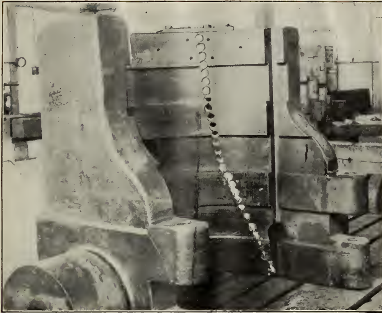
Fracture in Gun Cradle, Drilled Out Preliminary to Welding with Thermit Steel.
