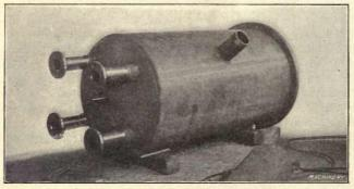
Fig. 1. Head, Flange and Branches welded in a 42-inch Tank with the Metallic Arc
