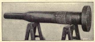
Fig. 2. A Built-up Fit on an Armature Shaft done with the Metallic Arc
