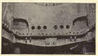
Fig. 3. Fractured Mud-ring of Locomotive Firebox prepared for making the Welds
