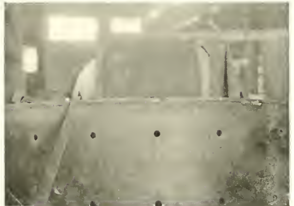
Fig. 70. Welding end on cylindrical tank.
