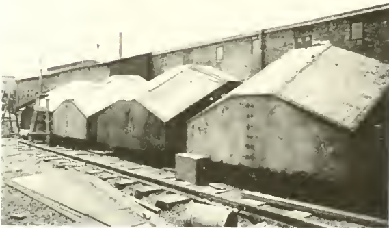
Fig. 3A. Fresh water tanks for welded ship. Lincoln Arc Welder. Speed of welding on these tanks is about 20 feet per hour.
