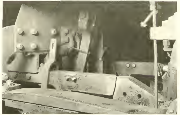
Fig. 53. Engine frame prepared for welding.
