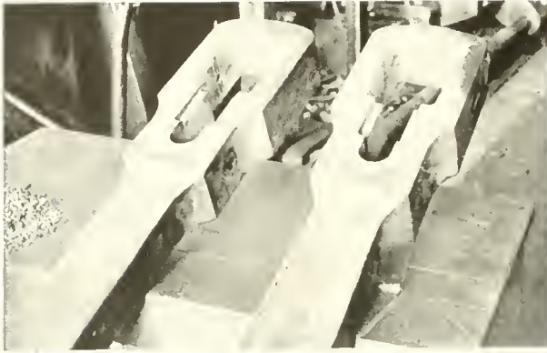
Fig. 31. Engine sub-roads repaired by electric arc welding. The ends of these rods were badly worn and new metal was built in by the use of the arc. One of these has been machined, the other shows only the rough weld, but so neatly was the work done that it is difficult to tell which is which.
