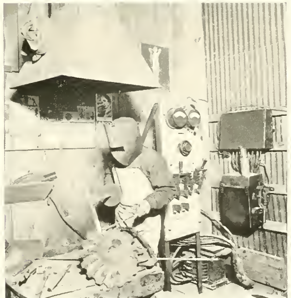
Fig. 25. Filling in a blow hole in a steel casting by the Carbon Electrode process
