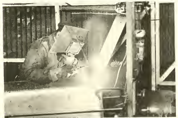
Fig. 11. Metal Electrode Welding. The electrode in this case is a metal wire of small diameter and this wire gradually melts itself away, furnishing metal for the weld.
