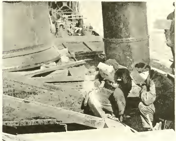
Fig. 57. Welding a Hatch Cover on a steel case.
