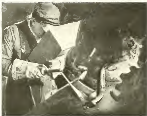
Fig. 86. Repairing drop forgings by the metal electrode process (shown a Lincoln Arc Welder).
