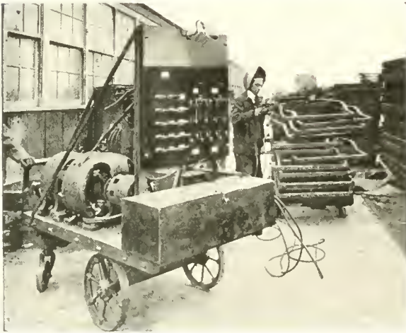
Fig. 5. Arc Welding can be applied anywhere that electric current is available and a cable can be carried. This is the most convenient method of welding.
