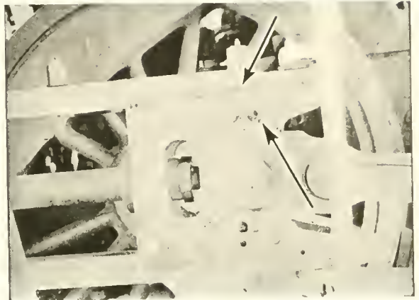
Fig. 46. Worn Engine Cross head repaired by welding on piece of boiler plate at the top and welding crack as shown.
