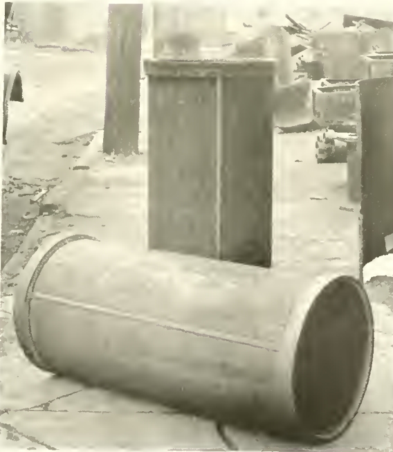
Fig. 104G. Typical welding job on 3/8 inch plate, and rings made of 5/8 inch stock. Using 200 ampere welder, 1/4-inch electrode welding 14 feet of seam per hour.
