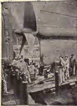
Fig. 191.—Repair of stern-post of steamer.
