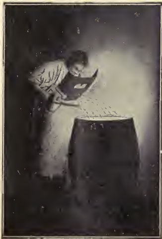
Fig. 7.—Welding by the voltaic arc.
