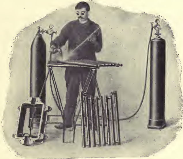
Fig. 39.—Welding with dissolved acetylene.
