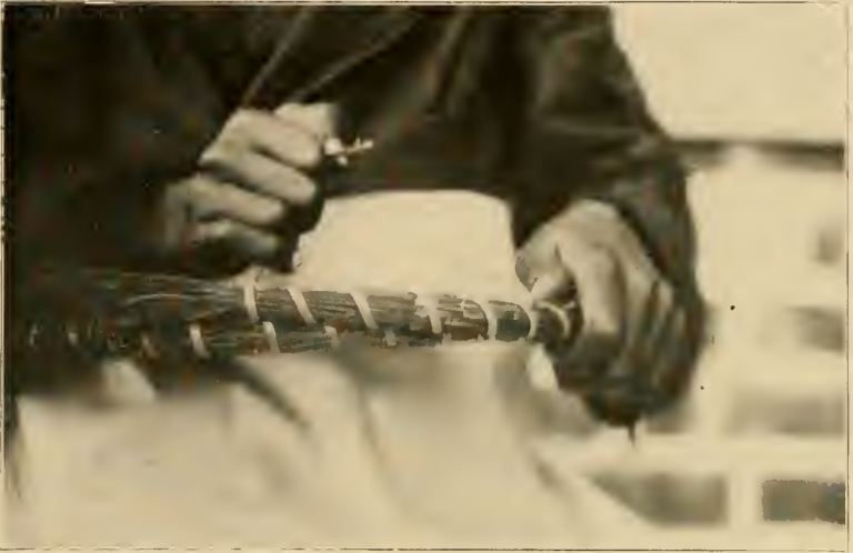
FIG. 23. STARTING TO BUILD UP THE SIDE OF THE BASKET.
