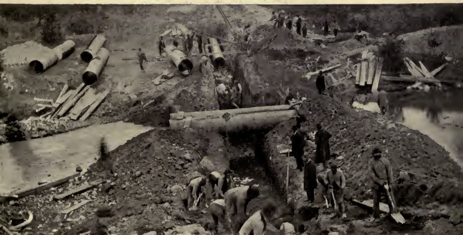
Laying Water-mains of 40- and 38-inch Steel Enamelled Pipe.
