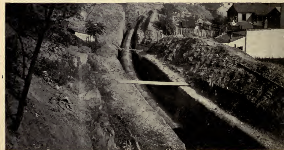
Laying Water-mains of 40- and 60-inch Steel Enamelled Pipe.
