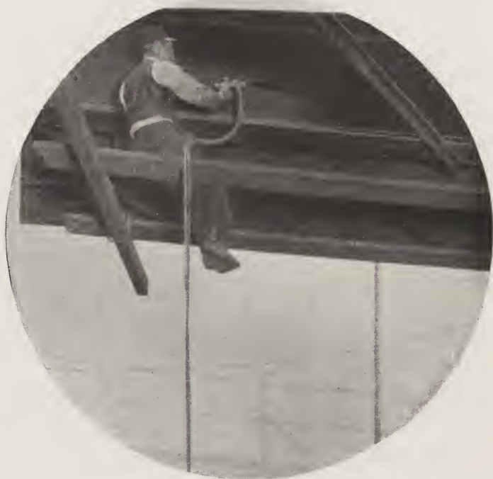
FIG. 48 Steel Girders of Elevated Railway Spray Paint Tests at Washington.
