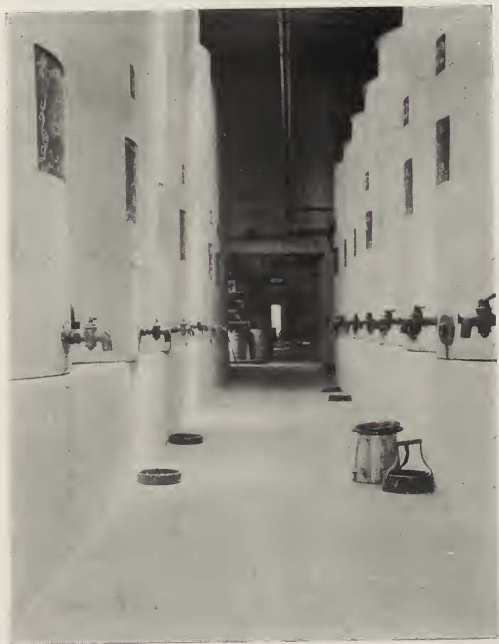
FIG. 54.—Varnish Storage. Louisville Varnish Co.
