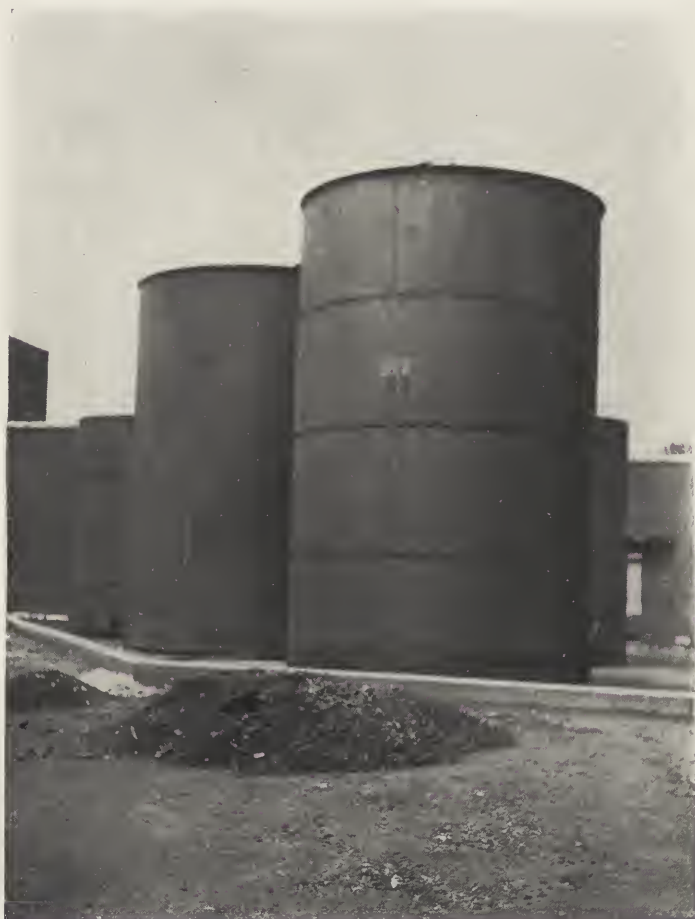
FIG. 53.—Turpentine Tanks. Louisville Varnish Co.
