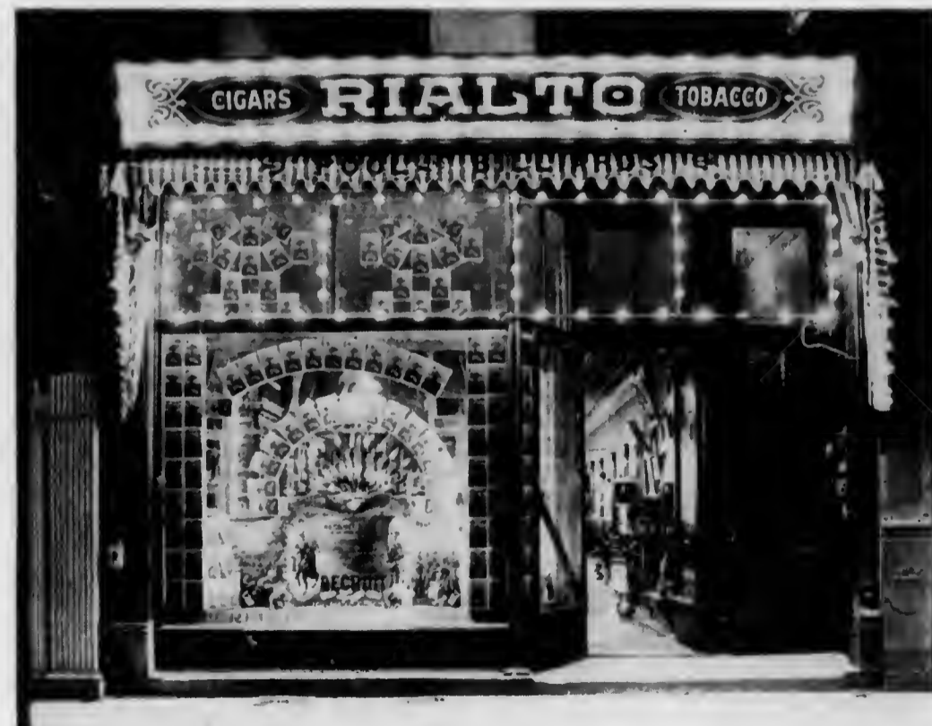
Fig. 1. Exterior View of Rialto Cigar Store Showing Outline and Sign Lighting
