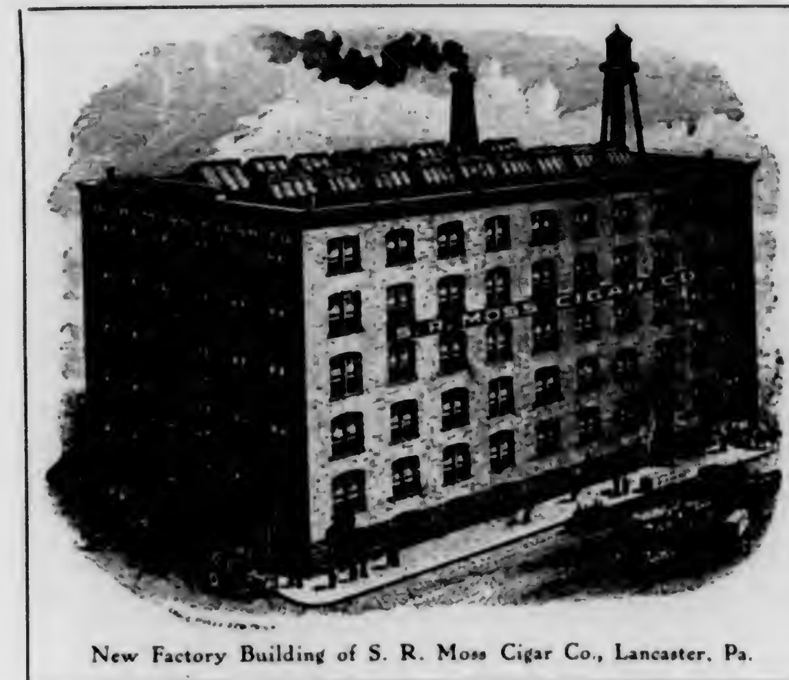
New Factory Building of S. R. Moss Cigar Co., Lancaster, Pa.
