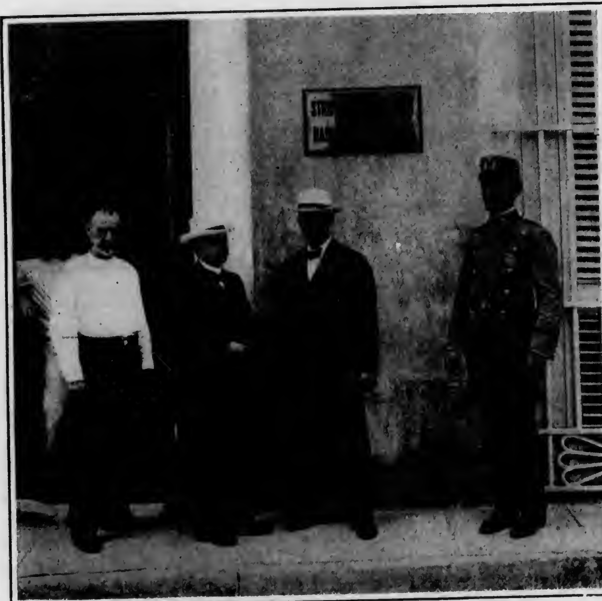
Exterior View, Stripping Department
