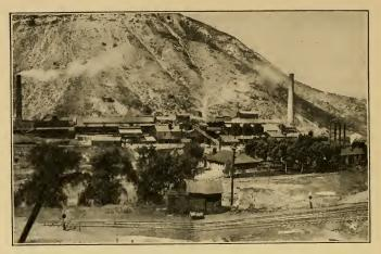
ONE OF THE GREAT SMELTERS Where the ore, after mining, is separated from the rock, and freed from impurities.
