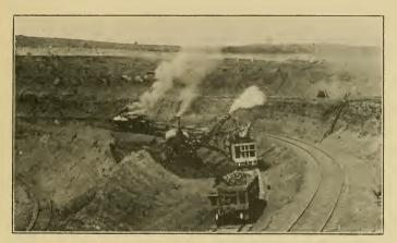
STEAM SHOVELS LOADING ORE In one of the mines in the Mesaba range. Note that tracks are laid on several levels.
