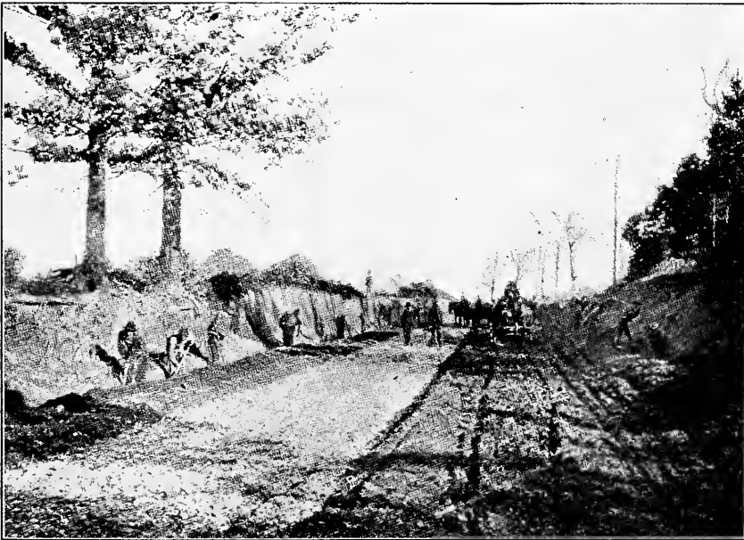
PREPARING THE ROADBED.
