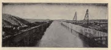
1. A section of the canal cut through solid rock.
