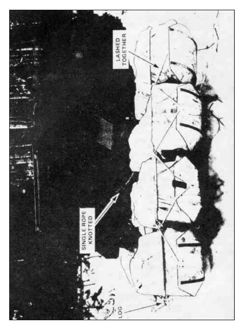
Figure 2-11 The Whippletree Method of Lashing Toboggans Together
