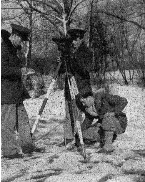
FIG. 29.—Obtaining horizontal control with transit and tape.
