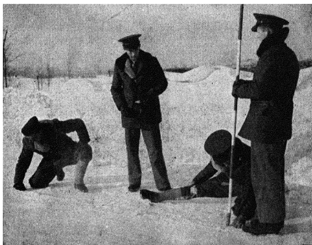
FIG. 17. —Taping under arctic conditions.
