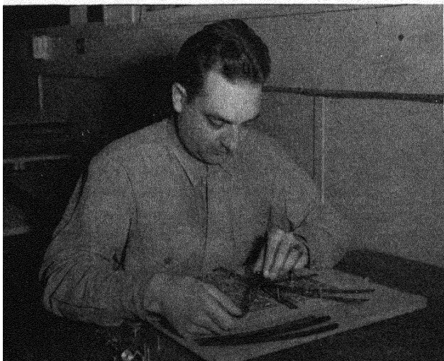
FIG. 172.—Placing radial arms over the pin guide shafts.
