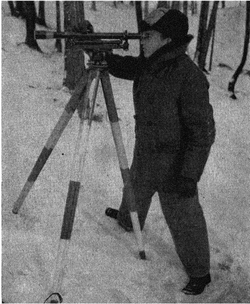
FIG. 38.—Differential leveling with Wye level.
