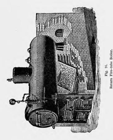
from there pass to the front through a number of tubes or flues. If the tubes are of greater diameter than six inches, they are usually spoken of as flues. The number of tubes varies with the diameter of the shell of the boiler and the diameter of the tubes.
