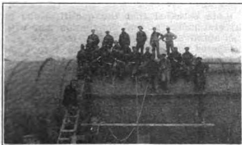
A GROUP OF MEN WORKING ON PIPE LINE AT PRESTON, IDAHO.
