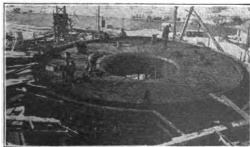
WORK FOR PIPE LINE AT PRESTON, IDAHO.
