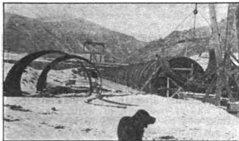
PIPE LINE AT PRESTON, IDAHO.
