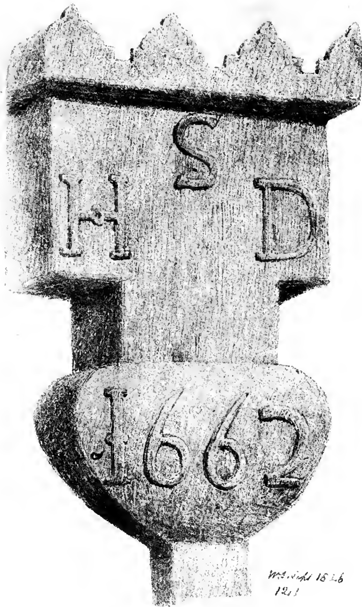
V RAINWATER PIPE-HEAD, STANWICK, YORKSHIRE
