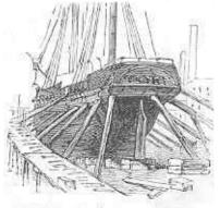
Then the water is let out by means of sluices in the gates, or it is pumped out, and the ship left dry. When the tide returns, the gates and sluices are all shut, and its entrance into the dock prevented, until such time as the ship is repaired, when water is let slowly in. As the vessel floats, the
