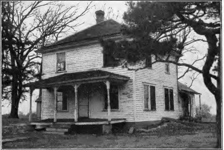
Figure 6. A typical example of the need for housing improvement. For one remodeling solution, see Figure 86.
