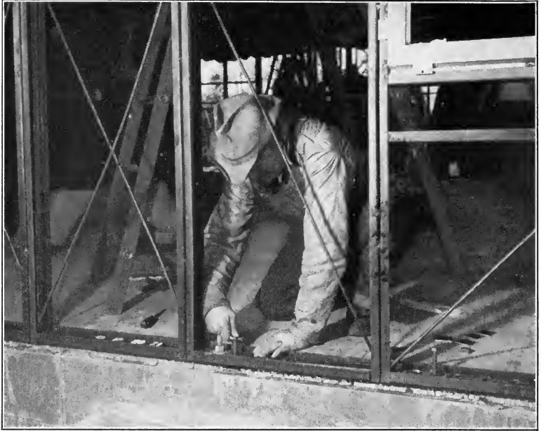
Figure 140. Use of metal in house framework.
