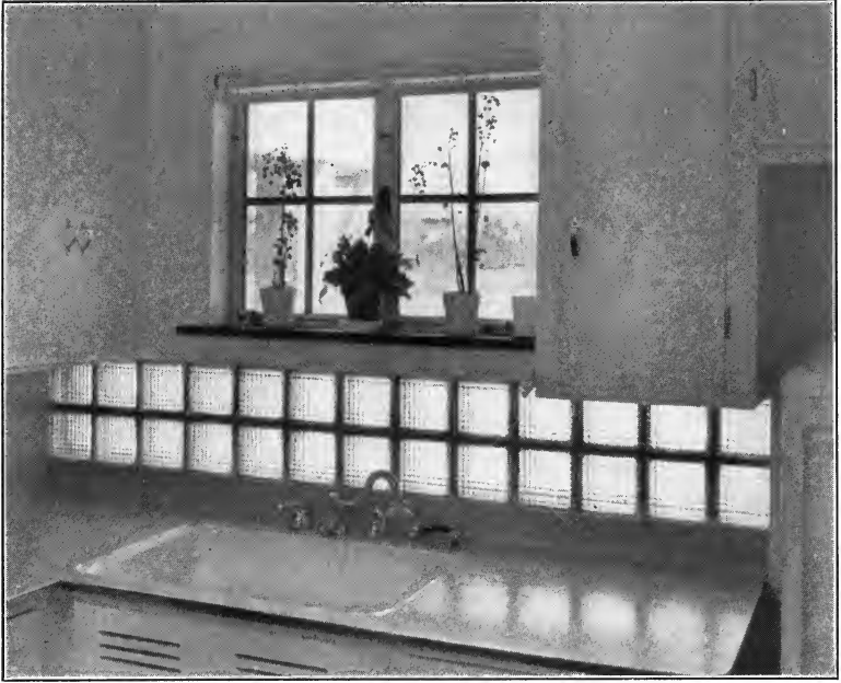
Figure 147. Effective use of glass block panel for both light and decoration.
