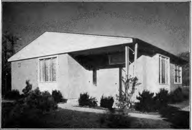
Figure 126. Prefabricated design, largely metal construction, both in framework and covering.
