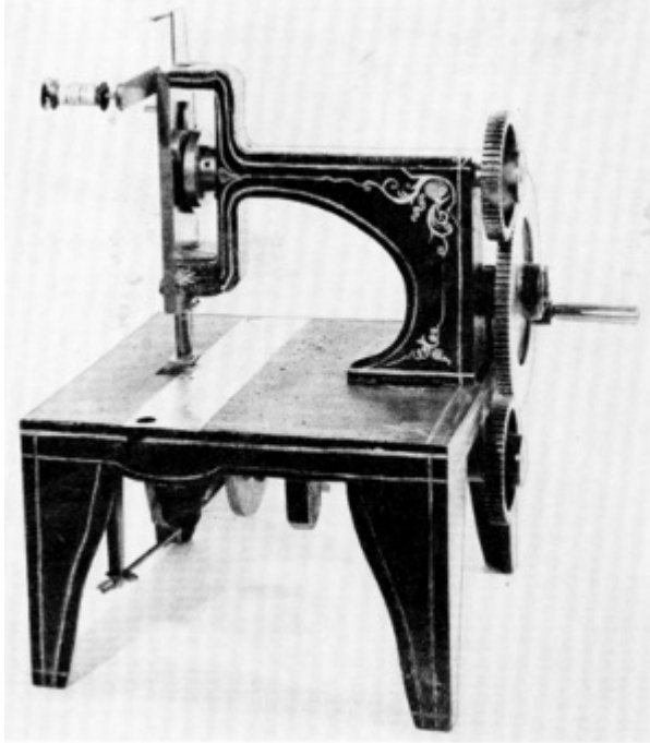
Figure 28.—Singer's patent model, 1851; a commercial machine was used, bearing the serial number 22. (Smithsonian photo 45572-D.)
