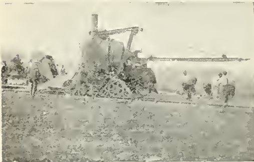
SMITH SIMPLEX PAVING MIXER, SIZE 21-E ON CONCRETE ROAD JOB.
