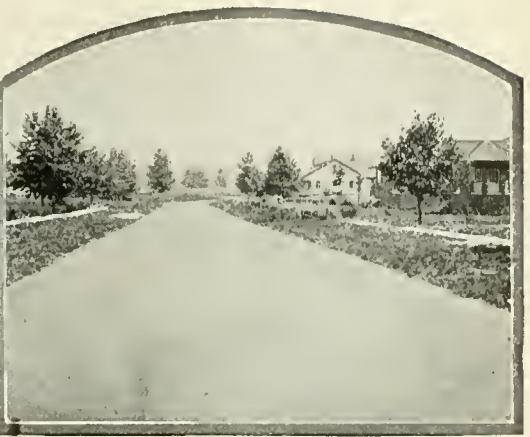
Picture of same section after being constructed with "Tarvia-X." Note excellent condition of road today
