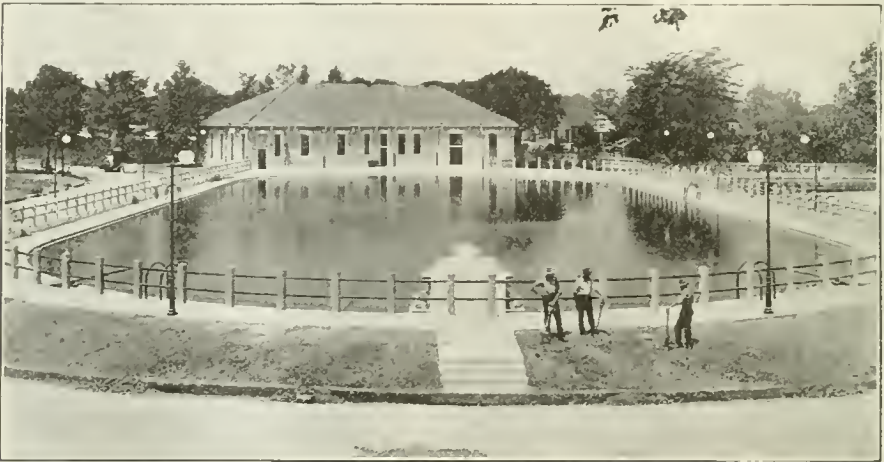
VIEW OF THE FINISHED CONCRETE SWIMMING POOL, LOUISVILLE WATER CO.
