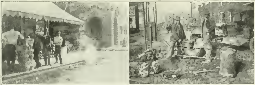
FIG. 1.—PUTRID VAPORS FROM SEWER MADE NEARBY STORES ALMOST UNINHABITABLE. FIG. 2.—WATER STANDS AT LEVEL OF DOTTED LINE IN THESE TRAPS, THUS PREVENTING ESCAPE OF VAPORS OR GASES.
