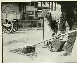
A seal-coat of 1/2 gallon of "Tarvia-KP" to the square yard is spread over the patch.
