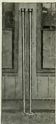
2-inch Service Pipe cast bell down in 9-foot lengths
