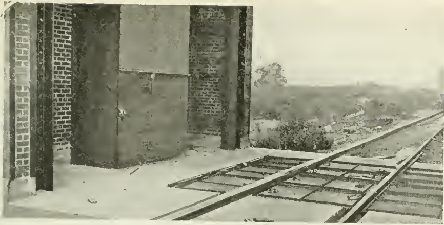
TRACK HOPPER AND CASING FOR VERTICAL RUN.
