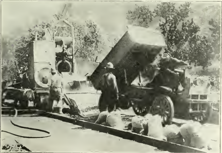
AUTOCAR TRUCK USED BY O'BRIEN BROS. (MARTINEZ, CALIF.) ON CONSTRUCTION OF PAVEMENT CONSISTING OF TWO 8-FT. CONCRETE STRIPS SEPARATED BY 4 FT. OF MACADAM.
