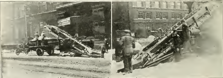
NEW BARBER-GREENE SNOW LOADER WORKING ON CHICAGO STREETS.
