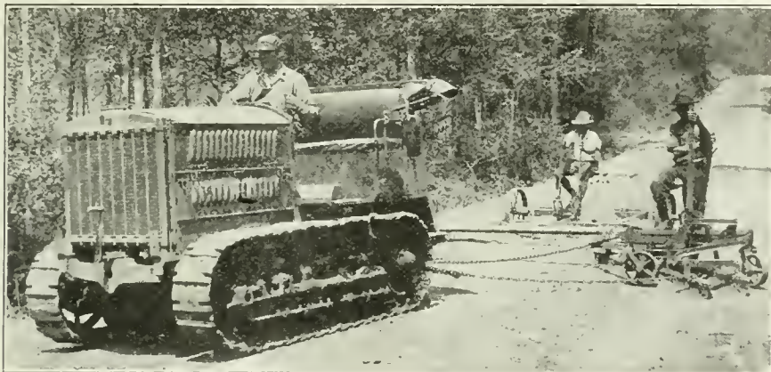
FIG. 7. "CATERPILLAR" TRACTOR PULLING ROAD MAINTAINER IN SUMPTER COUNTY, GEORGIA.
