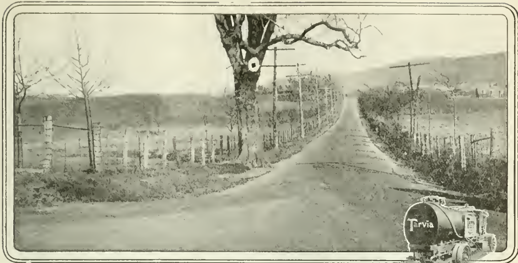
Hopwood to Brownfield Road, Fayette Co., Pa., built with "Tarvia-X" penetration method in 1917
