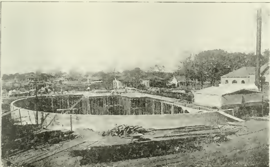
CONSTRUCTING ROOF FOR REINFORCED CONCRETE RESERVOIR AT ARKANSAS CITY, KANS.
