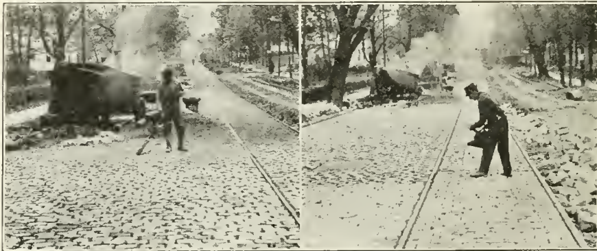
VIEWS OF ASPHALT-FILLED GRANITE BLOCK PAVEMENT CONSTRUCTION IN CINCINNATI, OHIO.
