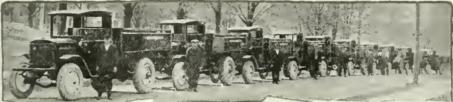
Fleet of special Kissel Road-Builders' trucks employed by Ogara Construction Company on Hartland (Wisc.) road contract.
