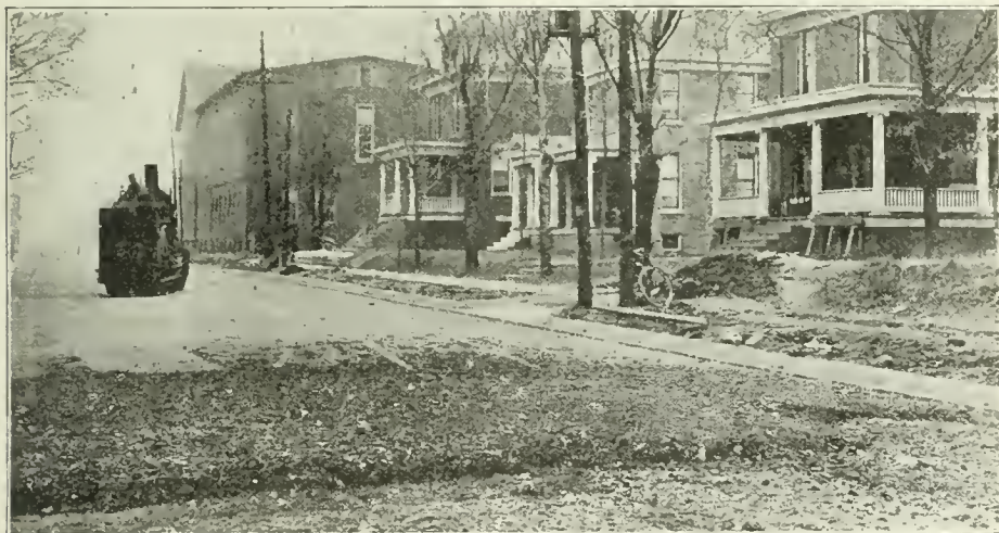
LAYING 5-INCH ASPHALTIC CONCRETE BASE AT OWENSBORO, KY.
