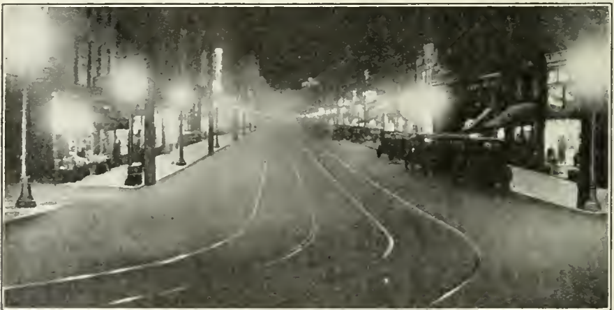
NIGHT SCENE IN NEW CASTLE, PA., SHOWING THE EFFECT OF IMPROVED WHITE-WAY LIGHTING. NOTE THAT MOST OF THE ILLUMINATION IS DOWNWARD SO THAT THE GREATEST EFFICIENCY IS OBTAINED.
