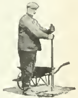
The mixture is well tamped and covered with screenings.
