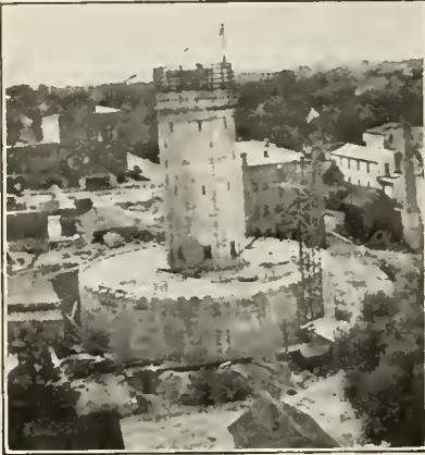
FIG. 2. RESERVOIR COMPLETED, TOWER UNDER CONSTRUCTION, ALBERT LEA, MINN.
