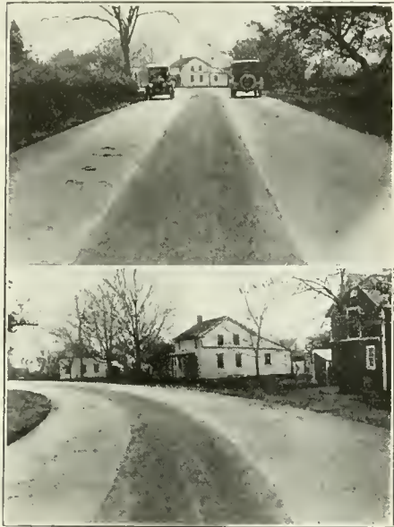
VIEWS OF MACADAM - CONCRETE DUAL TYPE OF HIGHWAY ON MAIN TRAVELED ROAD BETWEEN ALBANY AND NEW YORK, N. Y.
