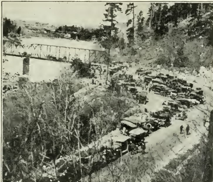
COLUMBIA RIVER HIGHWAY, PORTLAND, OREGON Warrenite-Bitulithic Surfacing over Old Macadam Sandy Road. Approach to the Columbia River Highway at Sandy River Bridge.
