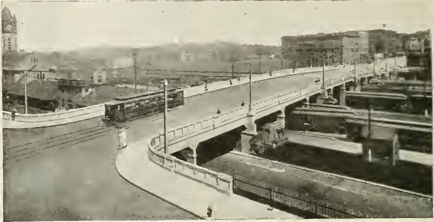
VIEW OF NEW GAY STREET VIADUCT AT KNOXVILLE, TENN.
