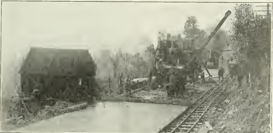
CONSTRUCTING AN 18-FT. CONCRETE ROADWAY WITH AN INDUSTRIAL RAILWAY FOR HAULING MATERIALS TO MIXER, McMULLEN (MD.) HIGHWAY.
