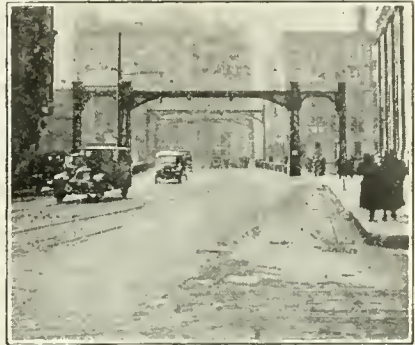
ONEIDA STREET, MILWAUKEE, WIS. LOOKING WEST TO ONEIDA STREET BRIDGE.
