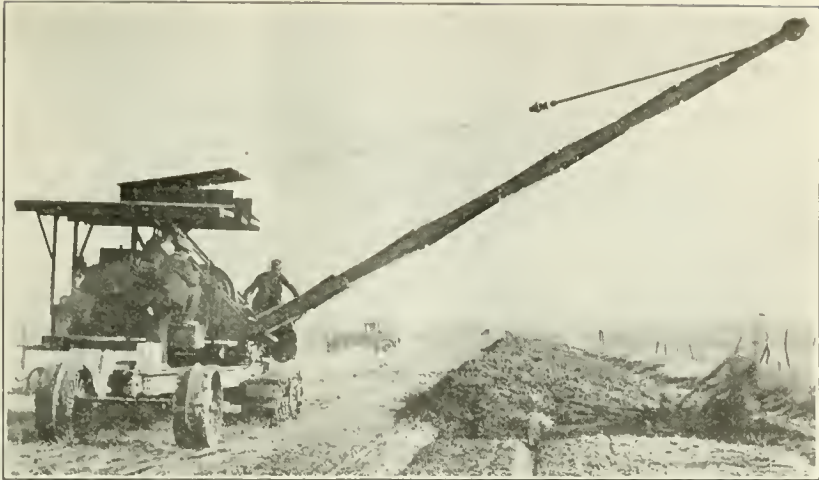
P & H Excavator-Crane Excavating Road Ditch and Grading Road
