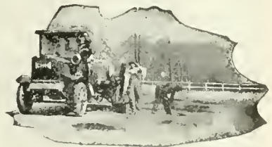
Road patrol maintenance crew patching improved road with "Tarvia-KP"
