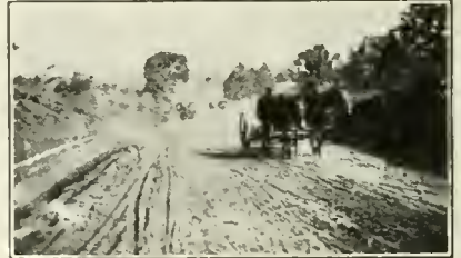
BEGINNING THE CUT.
