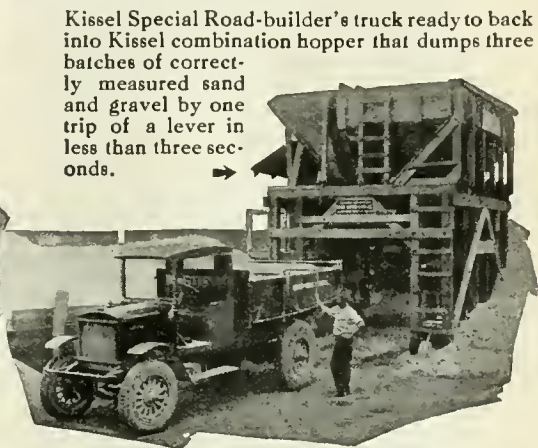
←Kissel Special Road-builder's truck. Hydraulic dump body of three batches of one yard each—designed, geared and powered for the flexibility, proper speed and dependable service necessary to meet contractors' requirements.
