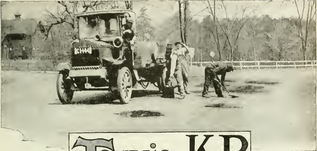
Patrol maintenance crew patching with "Tarvia-KP."
