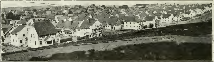
A REBUILT AREA IN HALIFAX, NOVA SCOTIA, SHOWING HOUSES OF CONCRETE BLOCK, STUCCO AND FRAME CONSTRUCTION. THIS IS THE NEW COLONY OF WORKMEN'S HOMES.
