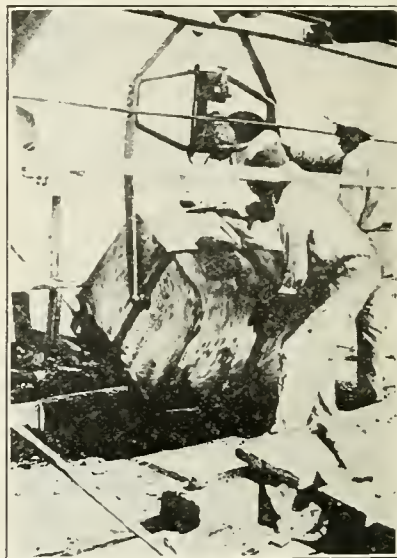
DUMPING ASPHALT FROM SKIP BUCKETS DIRECTLY INTO HOLD OF STEAMER AT BRIGHTON, TRINIDAD.
