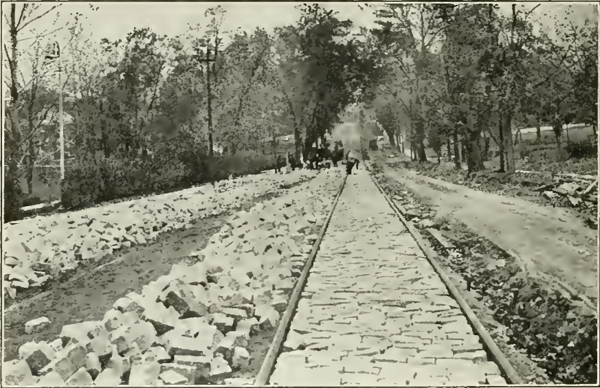
GRANITE BLOCK PAVEMENT CONSTRUCTION IN CINCINNATI, OHIO.
