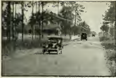
Fort Fisher Highway, New Hanover County, N. C. Treated with "Tarvia-B" 1915-17-18-19-21, and "Tarvia-A" in 1916.
