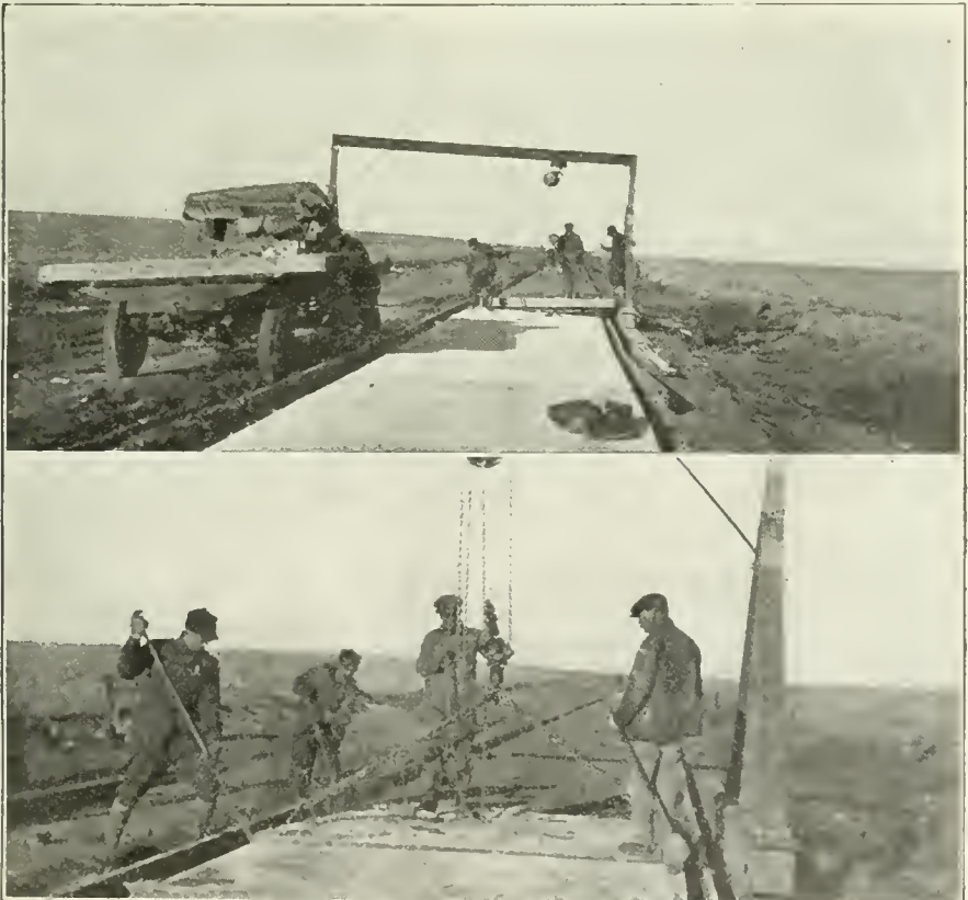
LAYING PRE-CAST CONCRETE SLAB PAVEMENT ON CASPER-SALT CREEK, WYOMING, HIGHWAY.
