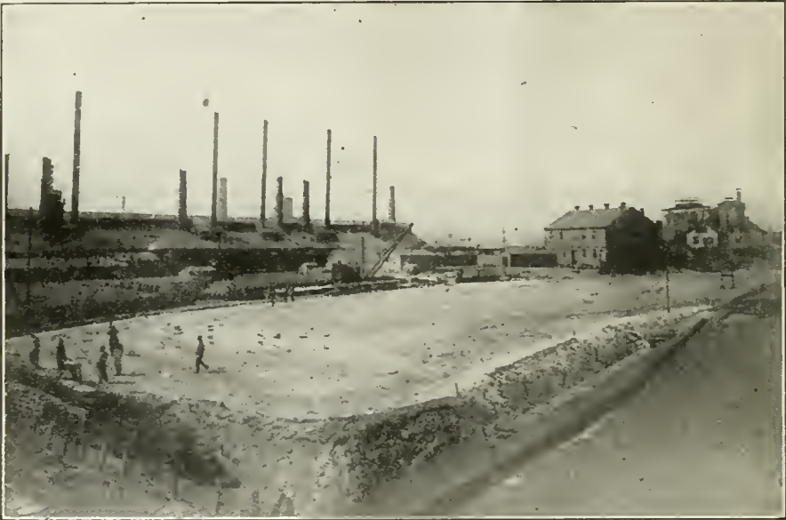
MINIATURE ASPHALT LAKE AT THE REFINERY AT MAURER, N. J. INTO THIS BASIN CRUDE ASPHALT IS DUMPED WHEN UNLOADED FROM STEAMERS, AND LEFT UNTIL NEEDED. THEN IT IS DUG OUT AND REFINED.
