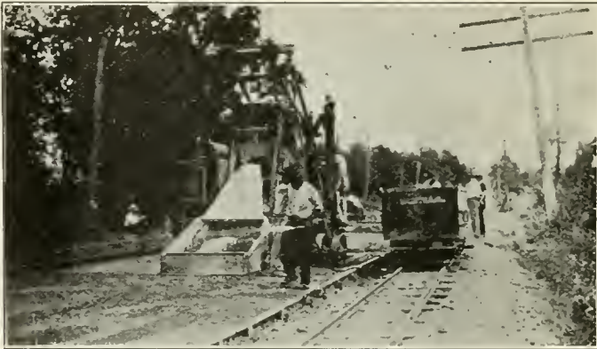
FIG. 7—SPRINKLING THE SUBGRADE AHEAD OF MIXER.
