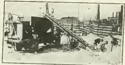
LOADING AGGREGATE HOPPERS MOUNTED ON MOTOR TRUCK WITH PORTABLE SCOOP CONVEYOR.
