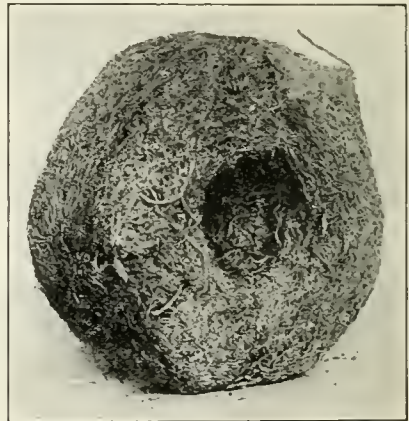
GROWTH REMOVED FROM \frac{3}{4} -IN. WATER METER AT LAREDO, TEXAS.
