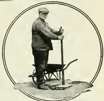
The mixture is well tamped and covered with screenings.
