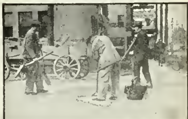
Screenings are scattered over the seal-coat and the patch is again tamped.
