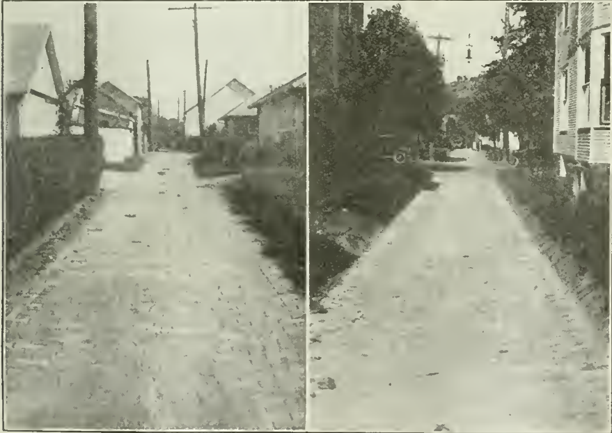
VIEWS OF ALLEYS IN LANCASTER, OHIO, PAVED WITH BRICK TAKEN FROM A STREET PAVEMENT 33 YEARS OLD.
