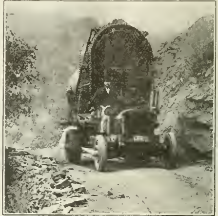
FEDERAL 5-TON TRUCK HAULING BOILER UP THE SIERRAS IN 1 DAY, A JOB FORMERLY REQUIRING 28 MULES AND 3 DAYS.
