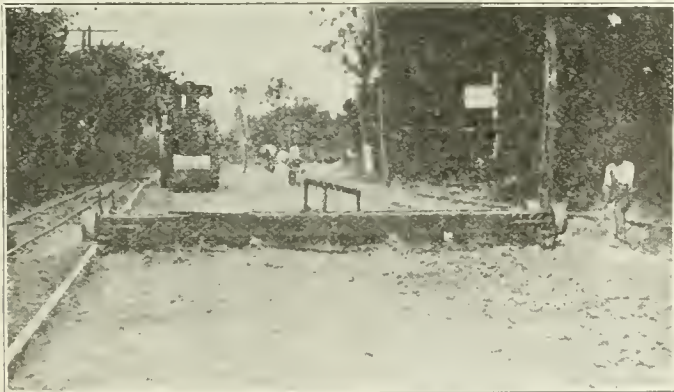
FIG. 9—LAKEWOOD SUBGRADER USED TO SHAPE SUBGRADE AHEAD OF MIXER.
