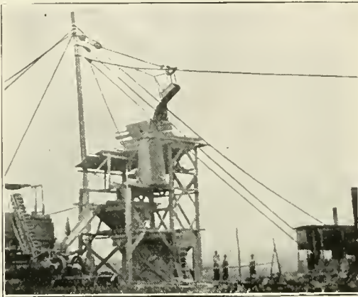
Small Sauerman Cableway operated by 70 h p. Double-Drum Steam Hoist. This outfit furnishes all the gravel needed for a Michigan Township's road work.
