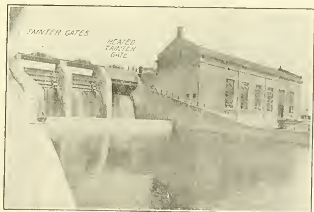
FIG 8. "FIVE CHANNELS" HYDRO-ELECTRIC PLANT OF THE CONSUMERS' POWER COMPANY, AU SABLE RIVER IN MICHIGAN, SHOWING 24 x 13-FT. TAINTER GATES.
