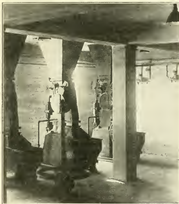
MACHINES FOR DRY-FEEDING SULPHATE OF ALUMINA, TWIN FALLS, IDAHO, WATER PURIFICATION PLANT.
