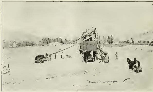
GRAVEL PIT SHOWING SCREENING PLANT OVER LOADING BINS.
