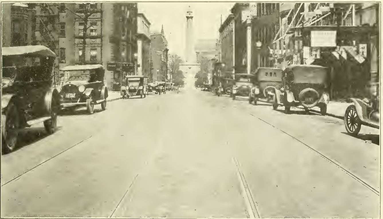
VIEW OF CHARLES STREET NORTH OF MULBERRY STREET, BALTIMORE, MD. Paved with Sheet Asphalt on Sides on 6 in. Concrete Base. Vitrified Block in Tracks with Wood Block Liners between Asphalt and Rails. Completed in 1915.
