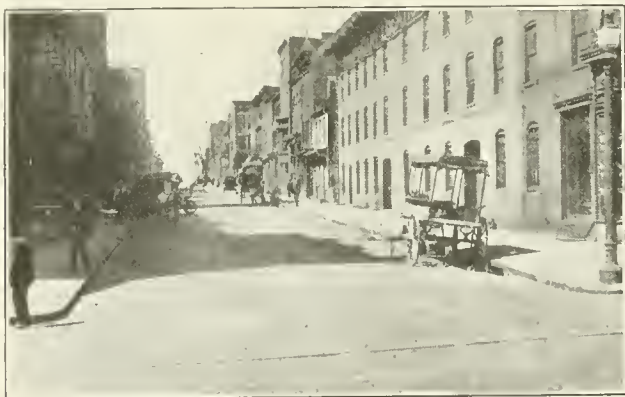
VIEW OF MULBERRY STREET WEST OF HOWARD STREET, BALTIMORE, MD. Paved with Sheet Asphalt on 6 in. Concrete Base with Brick Gutters. Completed in 1914.
