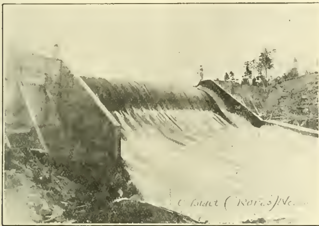
FIG. 6. UNDERHUNG COUNTERWEIGHT AUTOMATIC GATE AT OSFALDET (RORØS) NORWAY.
