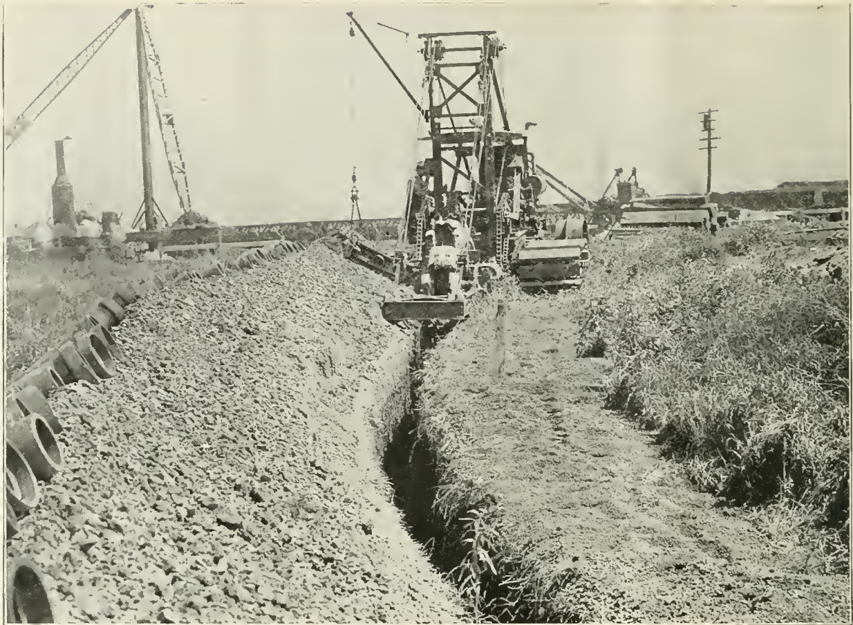
Wheel Type P & H Excavator Cutting a Curved Trench.
