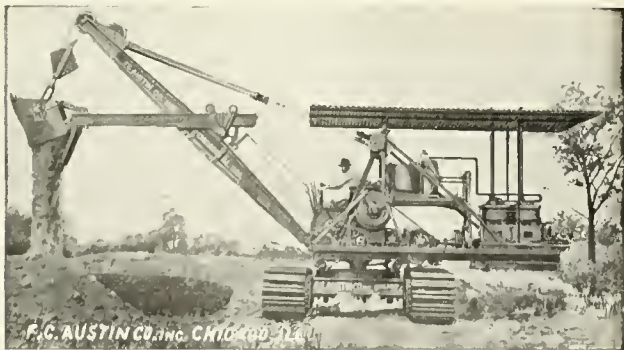
SHOWING HOW SHOVEL DIPPER IS ATTACHED ON AUSTIN COMBINATION DRAGLINE MACHINE.
