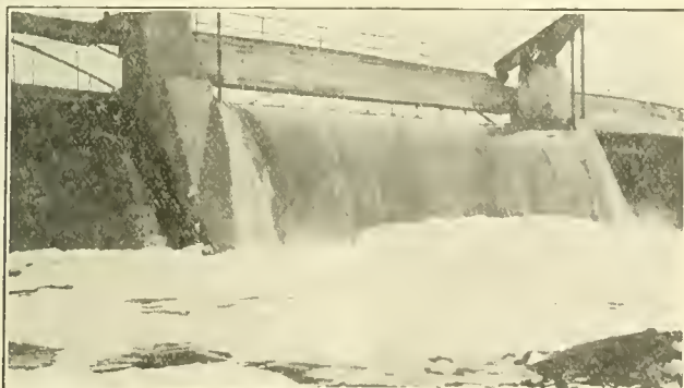
FIG. 7. OVERHEAD COUNTERWEIGHT AUTOMATIC GATE AT NASHUA, IOWA. SIZE 46 x 7 FEET. INSTALLED BY FARGO ENGINEERING CO.
