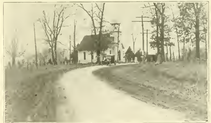
MONOLITHIC BRICK PAVEMENT 9 FT. WIDE, 5 IN. SLAB, STOCKLAND TWP., IROQUOIS COUNTY, ILL.
