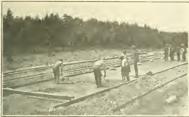
FIG. 1. USE OF TEMPLATES IN OBTAINING CORRECT SUBGRADE AND IN REDUCING WORK OF FINE GRADING.
