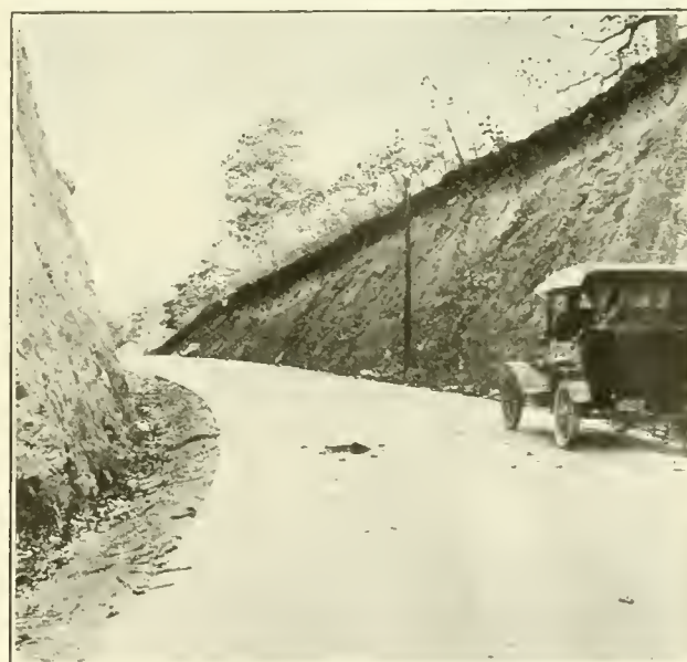
FIG. 2. ASHEVILLE-WILMINGTON-CHARLOTTE HIGHWAY AT MILE HOLE GAP, NORTH CAROLINA. This is also an Asphaltic Concrete Highway over old Macadam.
