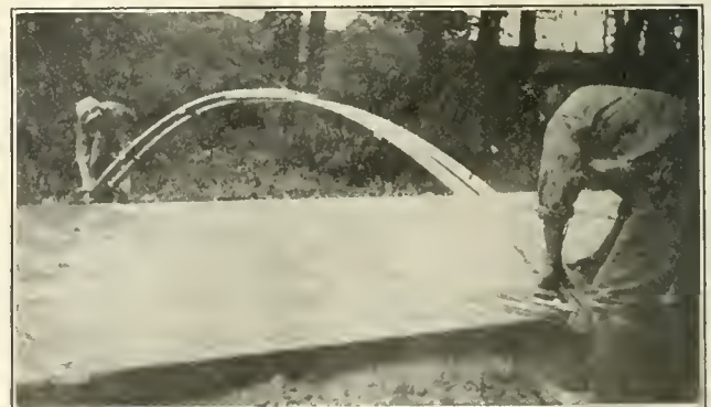
FIG. 9. LATEST METHOD OF BELT FINISHING A CONCRETE ROAD.
