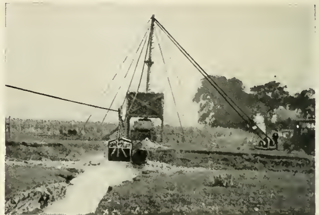
Small Sauerman Cableway operated by Double-Drum Belt Hoist driven by 20 h p. traction engine. This outfit used by Illinois Township.
