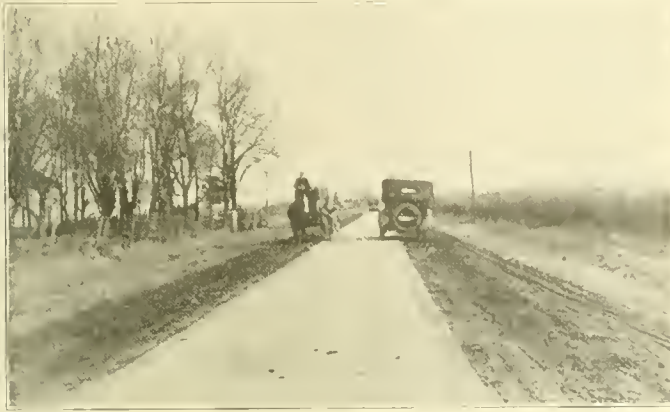
FOUR INCHES OF BRICK ON A ONE INCH CONCRETE BASE.
