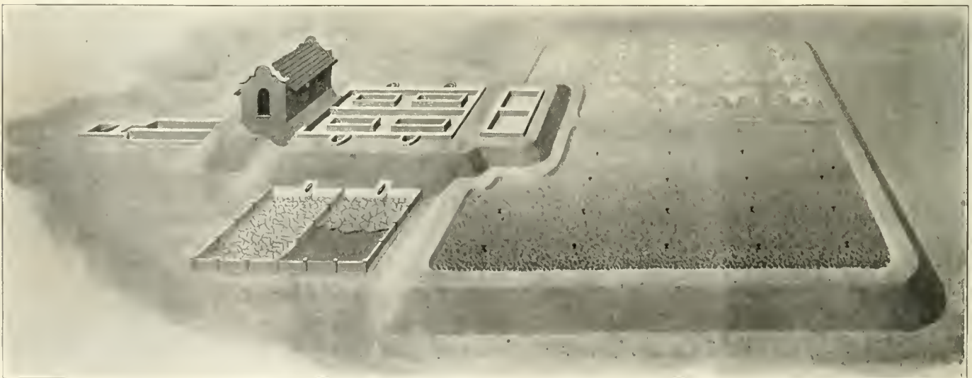
FIG. 1—GENERAL VIEW OF A TYPICAL SEWAGE DISPOSAL WORKS SHOWING, FROM LEFT TO RIGHT, BAR SCREEN, GRIT CHAMBERS, PUMPING STATION, IMHOFF TANKS, DOSING TANKS AND TRICKLING FILTERS, WITH TWO SLUDGE BEDS IN FOREGROUND.
