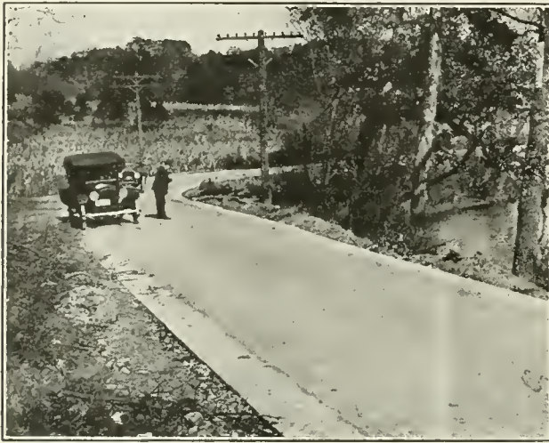
FIG. 3. CENTRAL HIGHWAY BETWEEN ASHEVILLE AND MOORHEAD CITY, NORTH CAROLINA. Built of Texaco Asphaltic Concrete over old Macadam.
