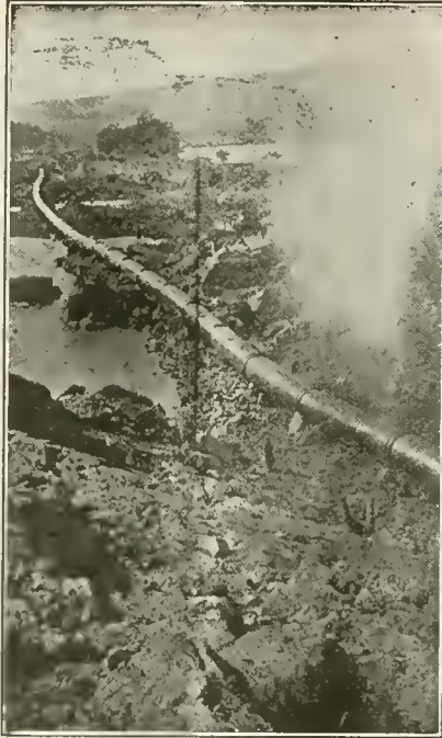
24-inch line looking south from Dam, through Medicine Canyon.
