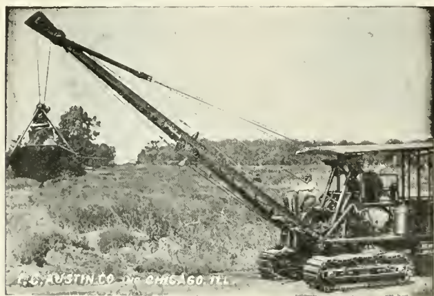
AUSTIN COMBINATION DRAGLINE MACHINE HANDLING ONE-HALF YARD CLAMSHELL BUCKET.
