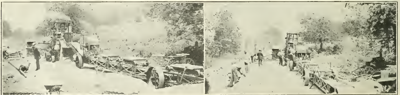
FIGS. 6 AND 7. TWO VIEWS OF THE KOEHRING MIXER LOADER IN OPERATION.
