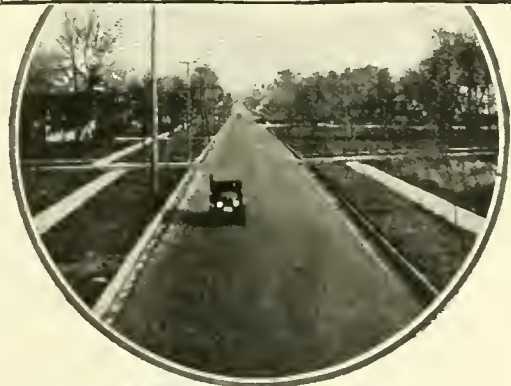
Above Washington Blvd., looking east from "Soo" R. R. viaduct, River Forest, Ill. Waterbound macadam treated with "Tarvia-B" in 1914 and 1916. "Tarvia-A" in 1918 and 1919.
