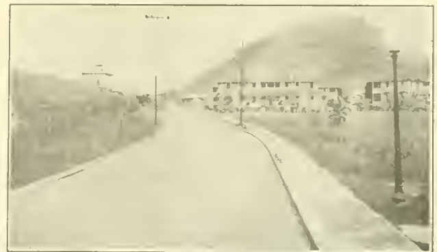
FIG. 1. SHEET ASPHALT WEARING SURFACE LAID ON A CONCRETE BASE ON THE HIGHWAY THROUGH PEDRO MIGUEL, PANAMA CANAL ZONE.
