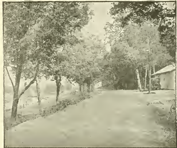
Three different sections of Marquette-Negaunee Road, Marquette County, Mich. These roads were waterbound macadam treated with "Tarvia-B" in 1917 and 1918. This is the main line of travel between the busy mining cities of Ishpeming and Negaunee, Mich. A traffic census revealed the passage over this road of 1980 vehicles per hour, the majority of which were automobiles.
