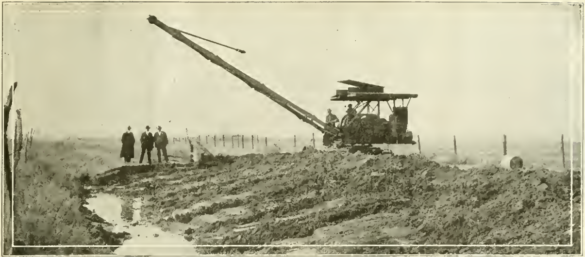
P & H Excavator-Crane Excavating a Ditch and Grading a Road.
