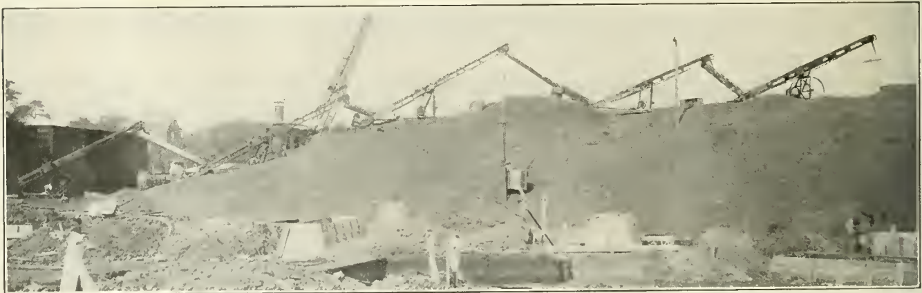
FIG. 1. UNLOADING COAL A DISTANCE OF 150 FT. WITH FIVE SCOOP CONVEYORS.
