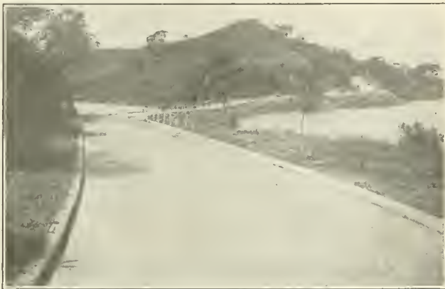
FIG. 2. A SECTION OF THE ANCON-PEDRO MIGUEL HIGHWAY; CONCRETE BASE, SHEET ASPHALT WEARING SURFACE.
