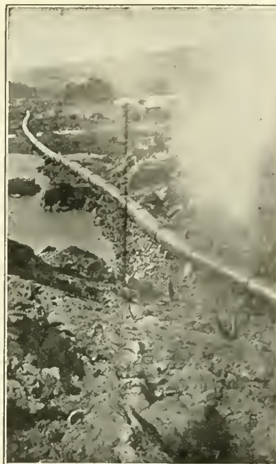
24-inch line looking south from Dam, through Medicine Caayoo.
