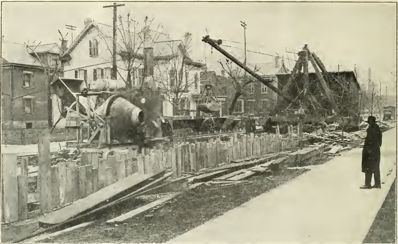
FIG. 6. EQUIPMENT USED ON CONSTRUCTION OF BUCKEYE STREET SEWER, HAMILTON, OHIO.
