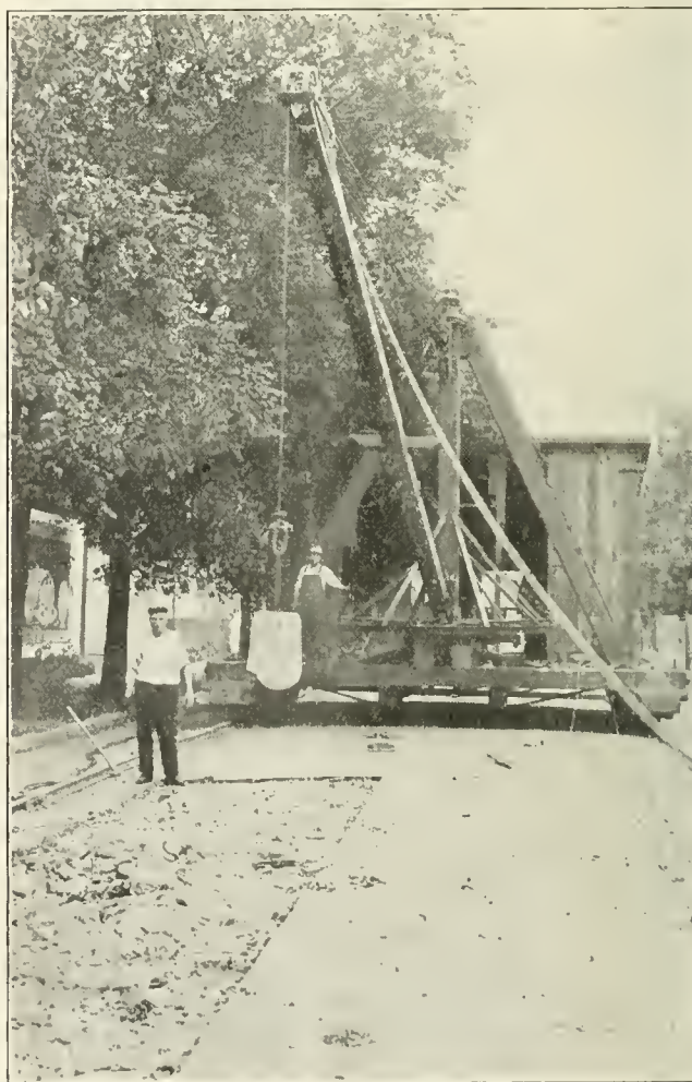
FIG. 1. BREAKING CONCRETE PAVEMENT BASE, ON SEWER CONSTRUCTION, HAMILTON, OHIO.
