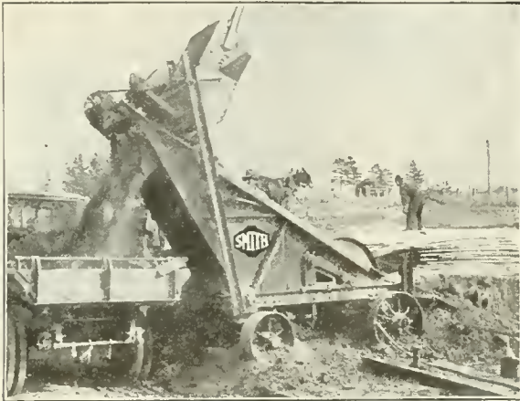
THE SMITH EXCAVATOR AND LOADER IN OPERATION.
