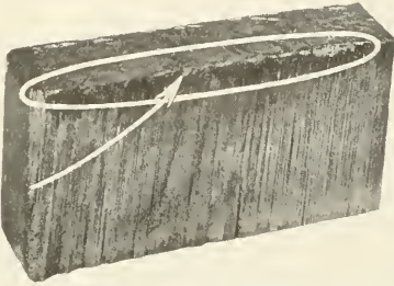
FIG. 2. THIS BLOCK WAS TREATED WITH KREOLITE OIL, UNDER TRAFFIC THREE YEARS, TAKEN UP AND FACE IMMERSED IN WATER 24 HOURS.
