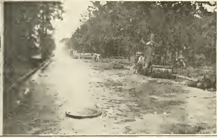
FIG. 5. THE SURFACE OF A ROLLER FINISHED CONCRETE BASE. FIG. 6. OPERATING A ROLLER ON A CONCRETE FOUNDATION TO BE COVERED WITH AN ASPHALT PAVEMENT.
