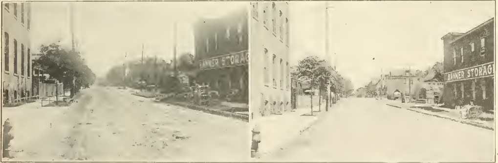
WALNUT STREET LOOKING EAST FROM 31ST STREET, MILWAUKEE WIS., BEFORE AND AFTER RESURFACING OLD MACADAM WITH TARVIA X.
