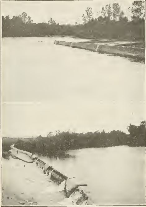
FIG. 3. DOWN STREAM VIEW SHOWING JUNCTION OF TAIL RACE WATER WITH THE MAIN CURRENT. Note the swells and wave action on opposite shore due to high velocity in main channel.
