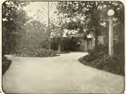
A driveway on the Lake Forest, Ill., estate of Mrs. C. H. McCormick. "Tarvia-X" two-course penetration and surfaced with "Tarvia-A."
