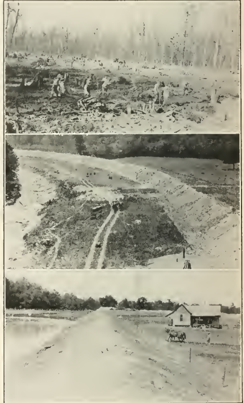
VIEWS OF OPERATIONS IN THE INTER-RIVER DRAINAGE DISTRICT, BUTLER COUNTY, MO.
