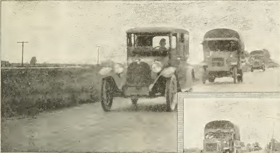
Ridout Road, Toledo, Ohio. All during 1918 this road was traversed by Army trucks being driven to the Atlantic seaboard. Macadam road resurfaced with "Tarvia-X" in 1918 and treated with "Tarvia-B" in 1916 and 1918.
