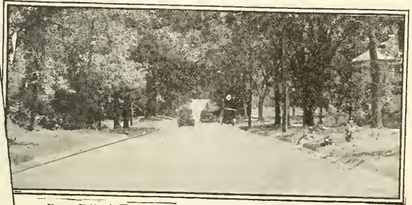
Upper—Hubbards Woods, Green Bay Road, Winnetka, Ill. Original treatment, "Tarvia-A" over macadam in 1907. Kept in prime condition up-to-date with the same material.
