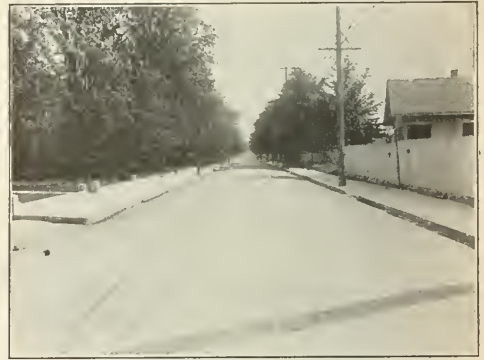
KENTUCKY ROCK ASPHALT PAVEMENT ON VIRGINIA AVE., HOPKINSVILLE, KENTUCKY. LAID IN 1917 ON A BROKEN STONE BASE.
