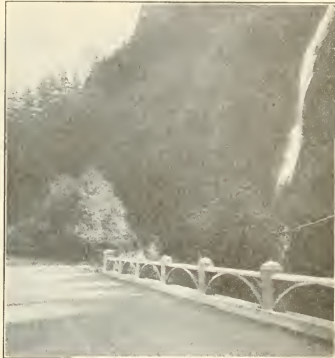
WARRENITE-BITULITHIC PAVEMENT LAID OVER OLD MACADAM.
