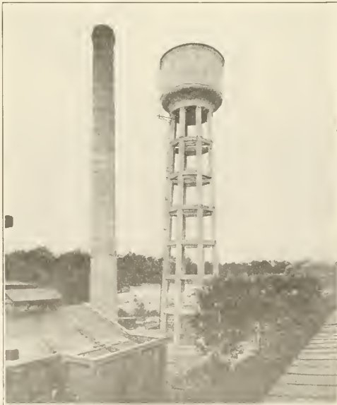
REINFORCED CONCRETE WATER TANK OF BUCKEYE COTTON OIL MILLS CO., ATLANTA, GA.
