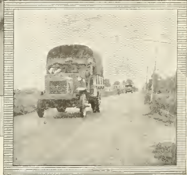
Ridout Road, Toledo, Ohio. All during 1918 this road was traversed by Army trucks being driven to the Atlantic seaboard. Macadam road resurfaced with "Tarvia-X" in 1918 and treated with "Tarvia-B" in 1916 and 1918.
