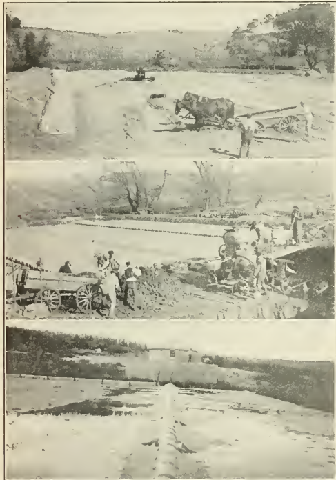
VIEWS OF FILTER BEDS OF MONTEZUMA, IOWA, SEWAGE TREATMENT PLANT.
