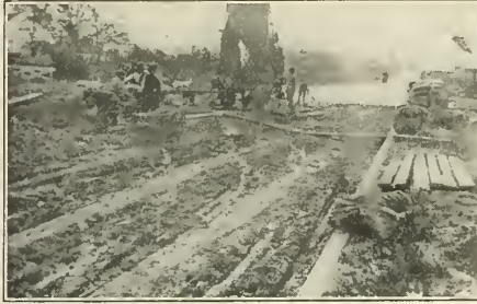
FIG. 5. THE SURFACE OF A ROLLER FINISHED CONCRETE BASE. FIG. 6. OPERATING A ROLLER ON A CONCRETE FOUNDATION TO BE COVERED WITH AN ASPHALT PAVEMENT.
