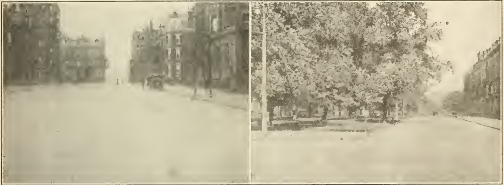
VIEWS OF WARRENITE-BITULITHIC PAVEMENT LAID ON OLD MACADAM FOUNDATION. Left: Dartmouth Street, Boston, Mass. Right: Commonwealth Avenue, Boston, Mass.
