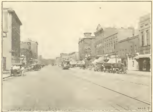
VIEW ILLUSTRATING SMOOTHNESS OF BRICK PAVEMENT WITH ASPHALTIC FILLER, MAIN STREET, GALESBURG, ILL.
