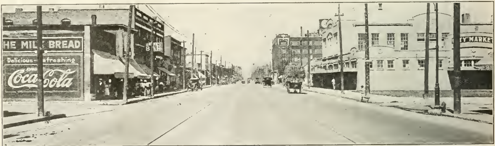
VIEW OF 4-INCH VITRIFIED VERTICAL FIBER BRICK BLOCK PAVING, WITH SQUEEGEED ASPHALT FILLER, ON SOUTH MAIN STREET, JOPLIN, MO.
