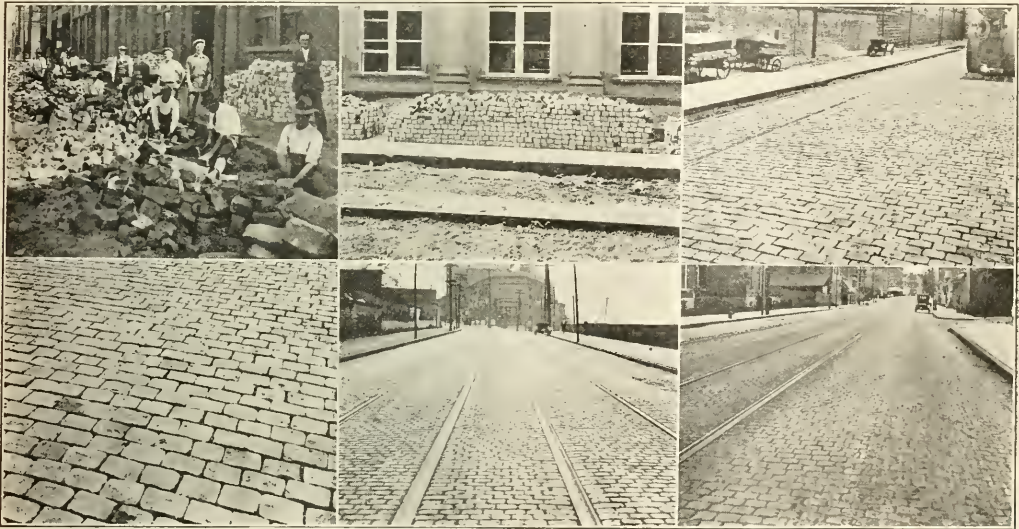
VIEWS OF GRANITE BLOCK PAVEMENTS IN CINCINNATI, OHIO.
