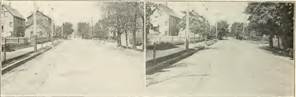
LOCUST STREET LOOKING WEST FROM EIGHTH STREET, MILWAUKEE, WIS., BEFORE AND AFTER RESURFACING OLD MACADAM WITH TARVIA X.
