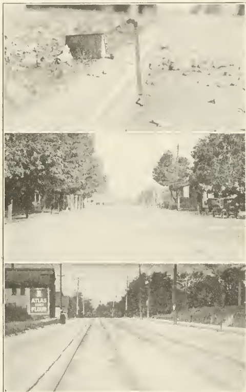
FIG. 4. FIVE INCH CURB ON STREET PAVED WITH CEMENT CONCRETE.
