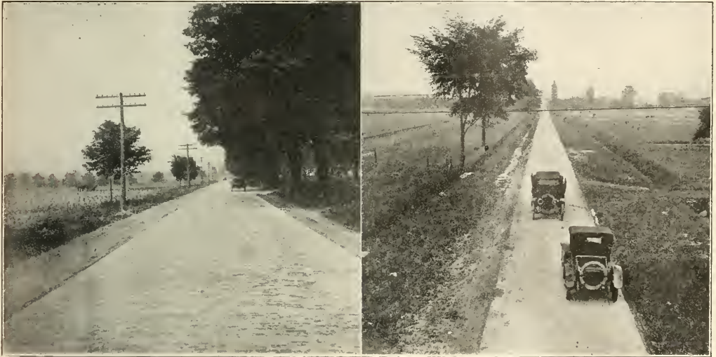
VIEWES OF TYPICAL, MODERN BRICK HIGHWAYS.
