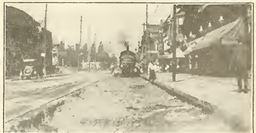
VIEW OF GRADE AS LEFT BY STEAM SHOVEL ON REPAVING OF DETROIT AVENUE, CLEVELAND.
