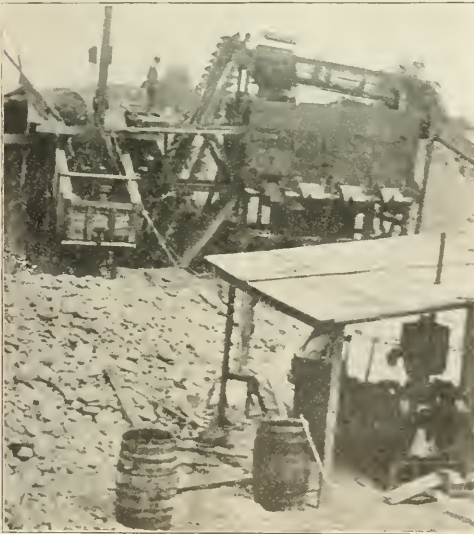
TWO MEN SCREEN 100 YDS. A DAY. One man in pit and one at hoisting engine of cableway operate this Oakland County (Mich.) plant.
