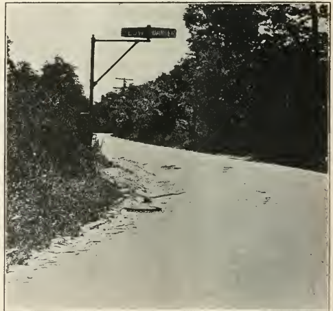
A. G. A. ACETYLENE-LIGHTED HIGHWAY DANGER SIGNAL AT DANGEROUS CURVE ON SHERIDAN ROAD, NORTH OF CHICAGO.
