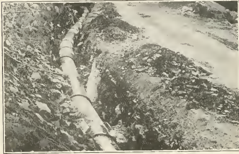
COMPOUND CURVE IN LINE OF 24-IN. "NATIONAL" MATHESON JOINT PIPE.
