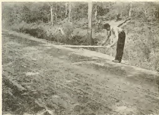
FIG. 4.—ROADWAY WELL ARCHED FOR DRAINAGE.
