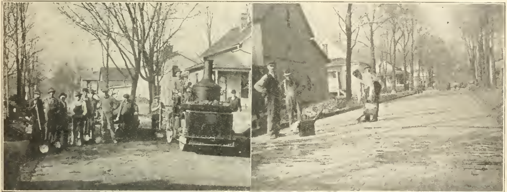
VIEWS ON BRICK PAVEMENT CONSTRUCTION AT MOUNT VERNON, OHIO.
