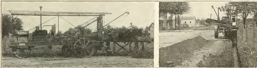
SIDE AND END VIEWS OF BUCKEYE CURB TRENCH EXCAVATOR.
