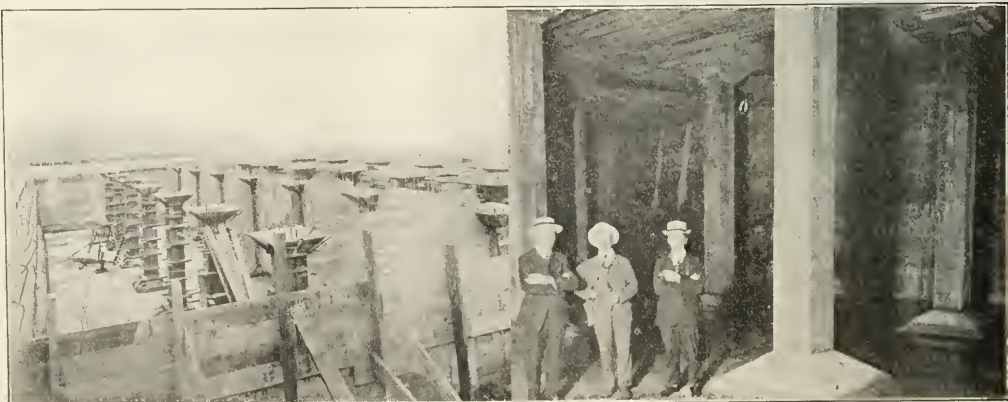
VIEWS OF REMODELED RESERVOIR OF OSHKOSH WATER WORKS.
