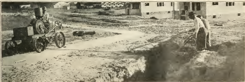
THE DETROIT WATER COMMISSIONERS USE TWO OF THESE OSHKOSH BACKFILLERS ON SMALL TRENCHES.
