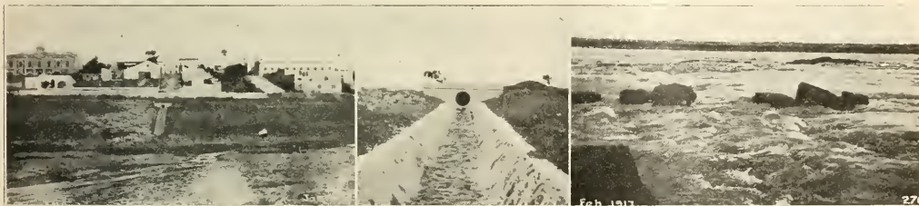
VIEWS OF WATER AND SEWERAGE WORKS AT SALTO, URUGUAY, SOUTH AMERICA.
