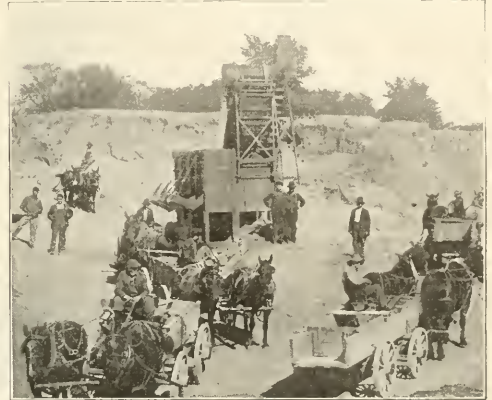
SCREENING PLANT OWNED BY TOWNSHIP. This "Ever Clean" Gravel Screener keeps 35 teams busy hauling away gravel.
