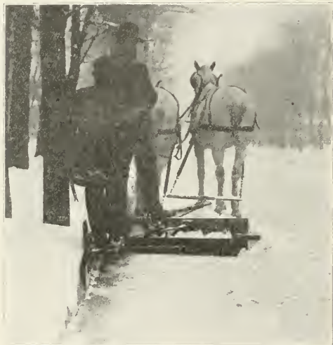
USING THE MARTIN DITCHER AND ROAD GRADER TO REMOVE SNOW FROM GUTTER TO FACILITATE RUNOFF OF SNOW WATER.
