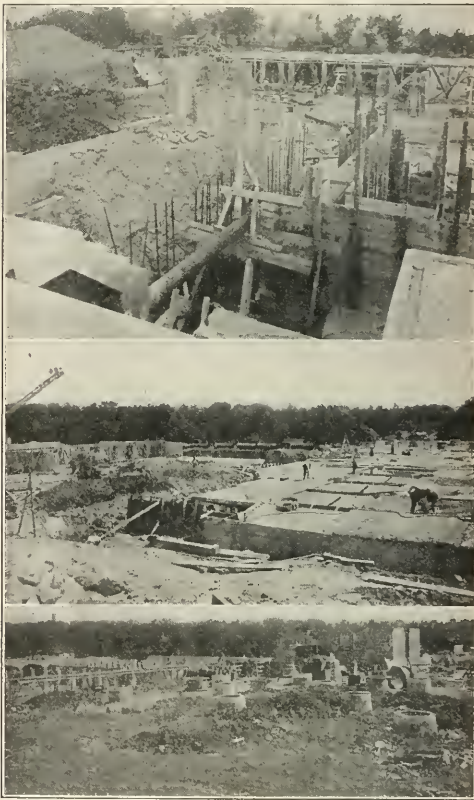
CONSTRUCTION VIEWS ON AUBURN, N. Y., FILTER PLANT.
