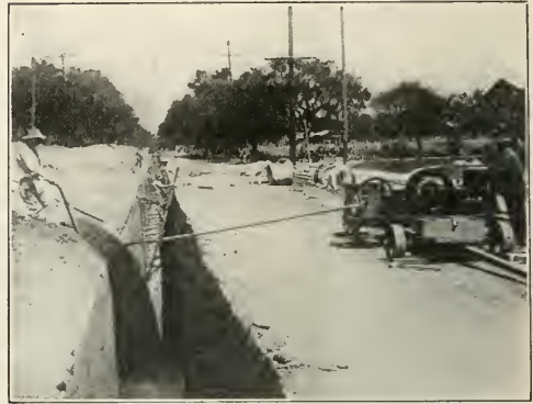
NON-TRACTION TYPE OF SMALL BACKFILLER. One of these Wonder "Double Quick" Machines Backfilled 14,986 Lin. Ft. at Average Cost of 3.1 Cents per Ft.
