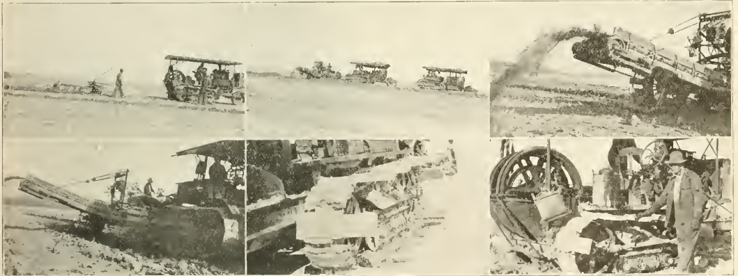
CONSTRUCTION EQUIPMENT USED ON LINCOLN HIGHWAY CUT-OFF AT GOLD HILL, UTAH.
