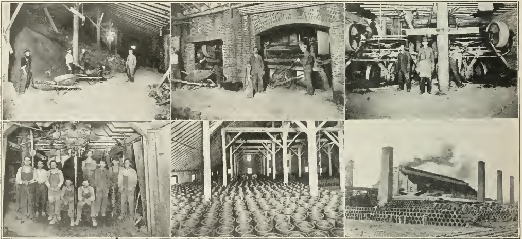
VIEWS OF REPRESENTATIVE VITRIFIED CLAY PIPE FACTORY.
