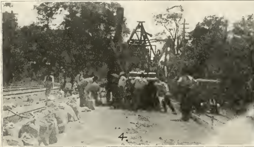
FIG. 4. ONLY FIVE WORKMEN NEEDED AT CHARGING END OF MIXER. FIG. 5. MEN'S ACTIONS BECOME ALMOST AUTOMATIC.
