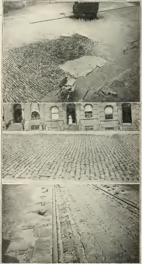
FILLER IN BLOCK PAVEMENTS.
