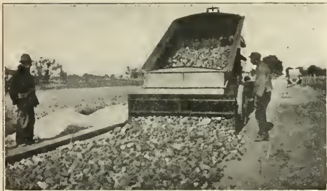
BURCH STONE SPREADER IN OPERATION.
