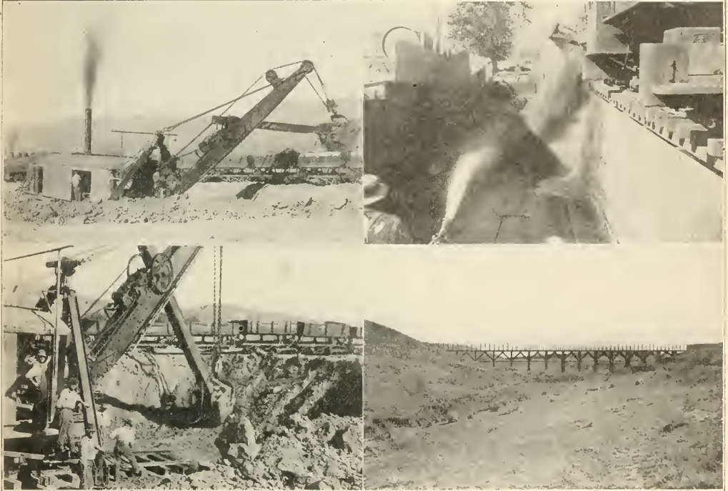
CONSTRUCTION VIEWS ON LOS ANGELES AQUEDUCT IRRIGATION DEVELOPMENT.
