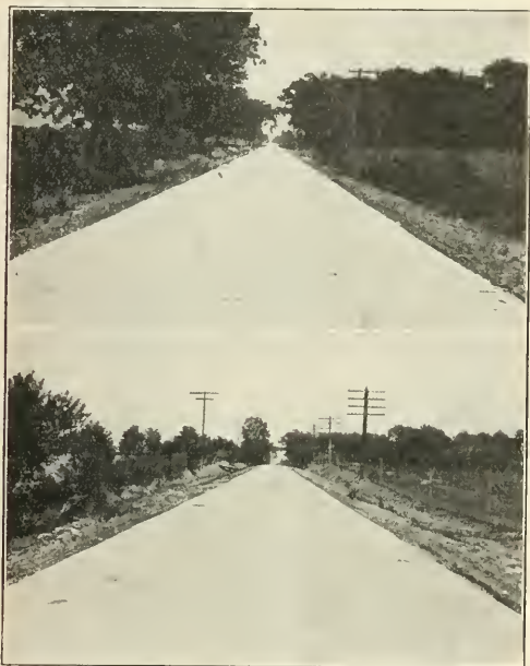
VIEWS ON BLAST FURNACE SLAG SECTION OF YOUNGSTOWN-AKRON (OHIO) CONCRETE ROAD.
