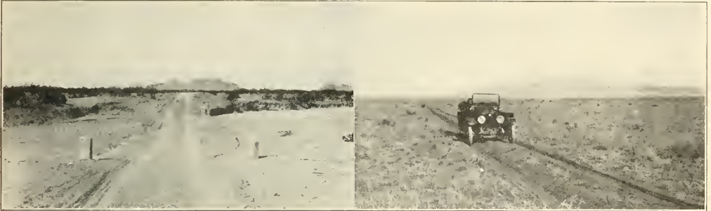
LEFT: (NO. 1, SEE TEXT) CONCRETE FLOORING ON STATE ROAD NO. 3. IN DONA ANA COUNTY, NEW MEXICO. RIGHT: (NO. 7) TYPE OF PRAIRIE ROAD USED IN SANDY, GRASSY PLAINS COUNTRY.
