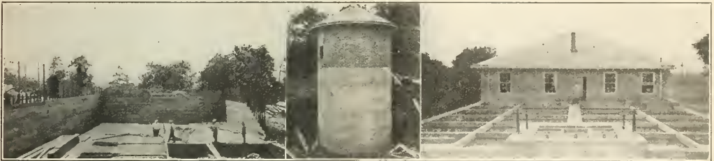
VIEWS OF NEW WATER PURIFICATION WORKS AT CHECOTAH, OKLA.
