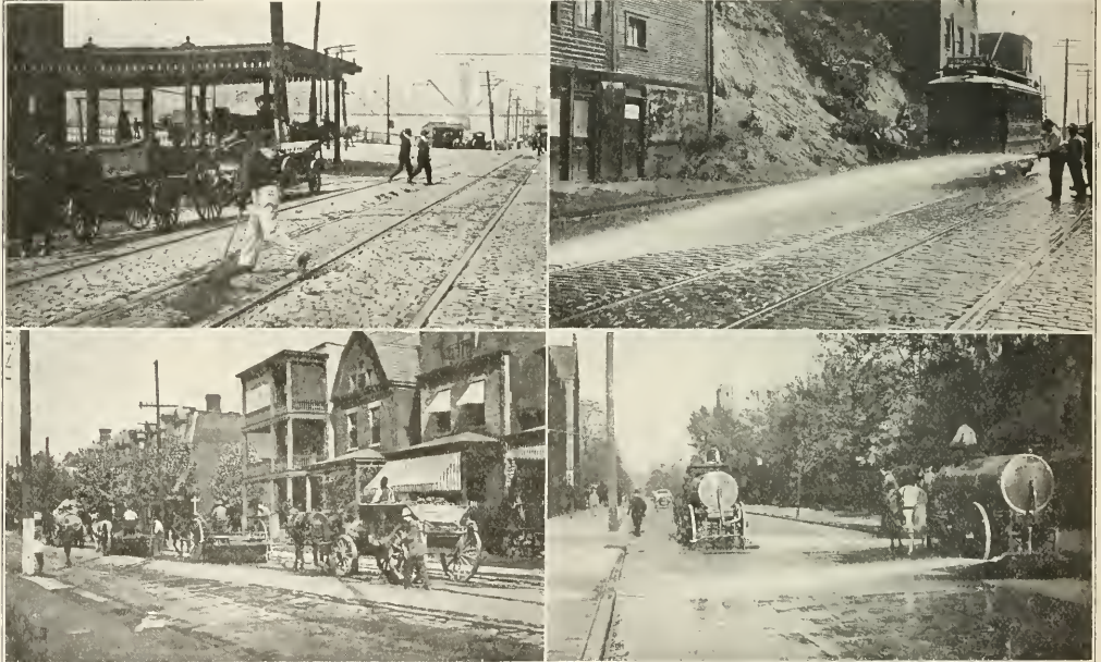
VIEWS ILLUSTRATING STREET CLEANING METHODS AND EQUIPMENT EMPLOYED IN PITTSBURGH, PA.
