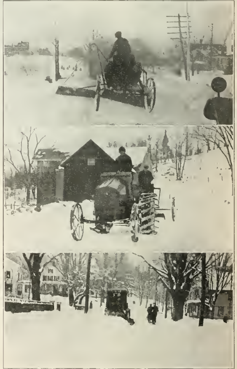
VIEWS SHOWING REMOVAL OF SNOW FROM CONNECTICUT TRUNK LINE HIGHWAYS.
