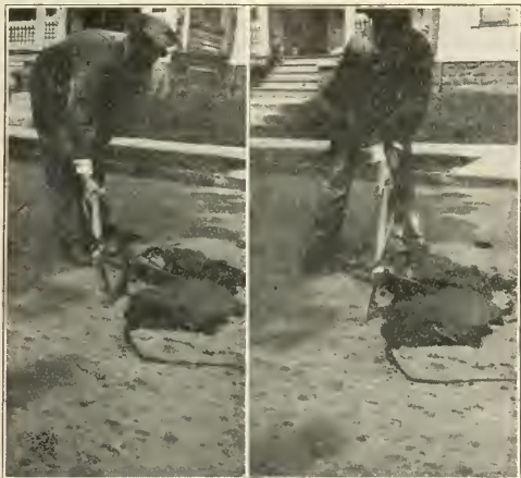
VIEWS ILLUSTRATING WRONG AND RIGHT METHODS OF HOLDING ASPHALT CUTTING TOOLS.
