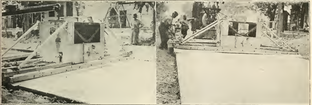
VIEWS OF NEW LAKEWOOD CONCRETE ROAD FINISHER IN USE ON 15 FT. BELLEVILLE (ILL.) SCOTT FIELD ROAD IN ST. CLAIR COUNTY.
