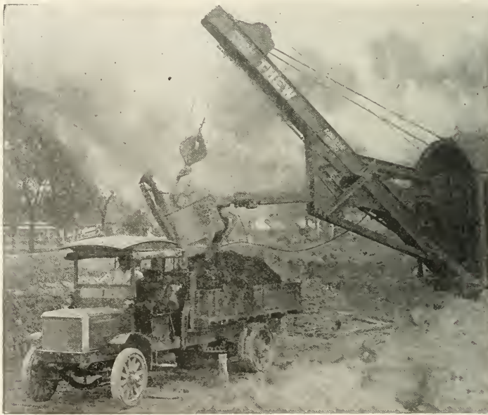
FEDERAL TRUCK HAULING EXCAVATED MATERIAL, HENRY FORD HOSPITAL CONSTRUCTION, DETROIT, MICH.
