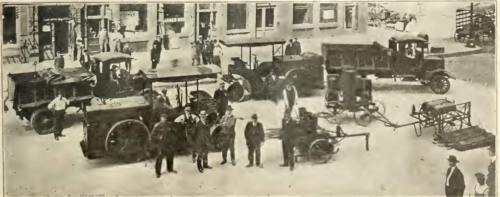
VIEW OF SMOKELESS EQUIPMENT USED IN REPAIRING ASPHALT STREETS IN CHICAGO.
