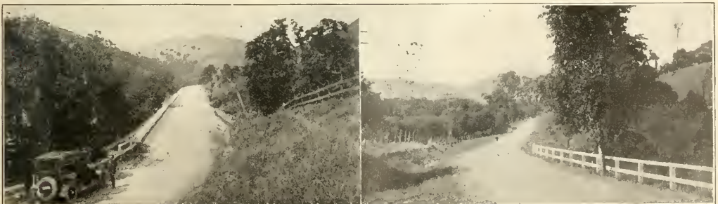
VIEWS OF CONCRETE PAVEMENTS ON CALIFORNIA STATE HIGHWAYS.
