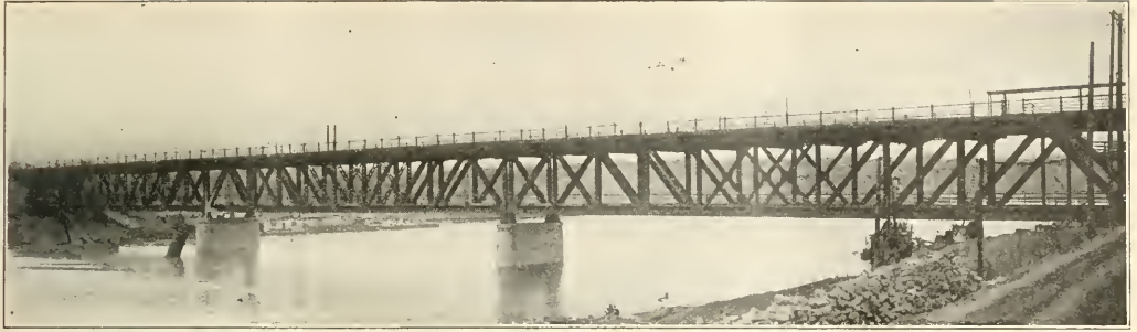
VIEW OF THREE-SPAN, DOUBLE DECK BRIDGE ACROSS KANSAS RIVER, AT KANSAS CITY, KANS.
