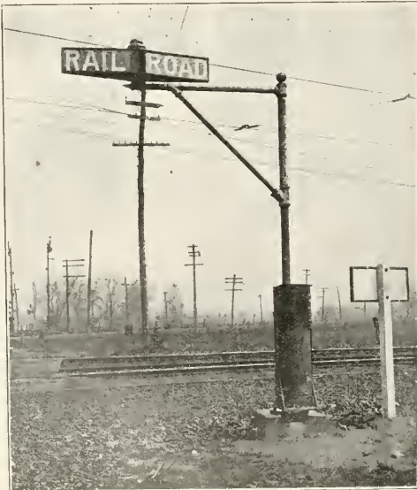
HIGHWAY DANGER SIGNAL OF A. G. A. TYPE INSTALLED BY INDIANA UNION TRACTION CO. AT CROSSING OF ITS ANDERSON LINE WITH ORCHARD AVE., A HIGHWAY, JUST OUTSIDE OF INDIANAPOLIS.
