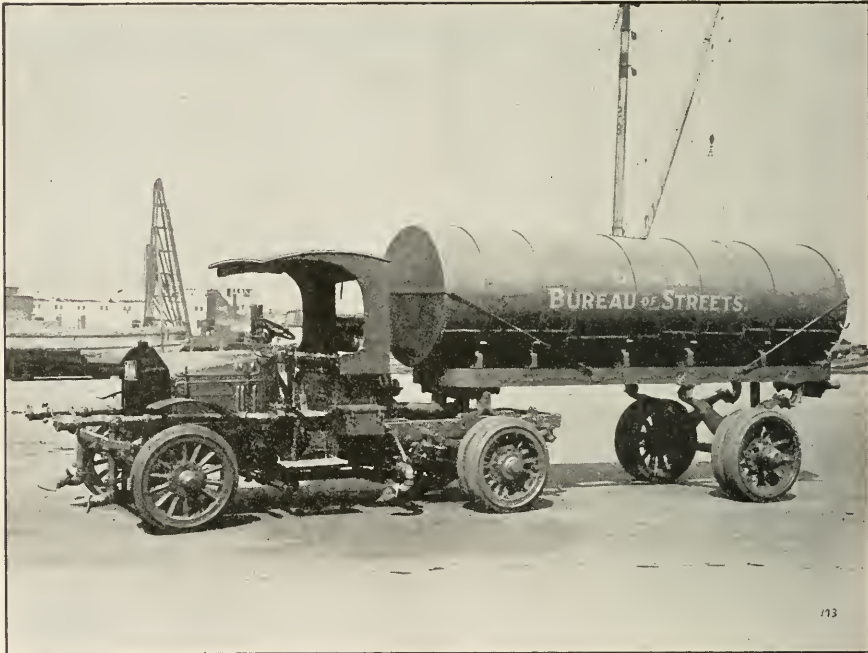
MOTOR FLUSHING AND SPRINKLING UNIT OPERATED BY BUREAU OF STREETS, BUFFALO, N. Y.
