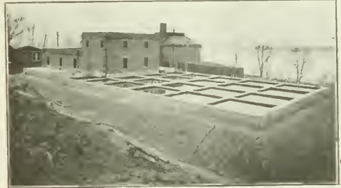
VIEW OF WATER PURIFICATION PLANT, HENDERSON, KY., WHERE SEDIMENTATION AND MECHANICAL FILTRATION ARE FOLLOWED BY ULTRA-VIOLET RAY STERILIZATION.
