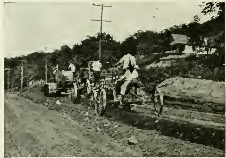
BLADE GRADER AND REVERSIBLE GRADER HITCHED TANDEM AND DRAWN BY CATERPILLAR TRACTOR.
