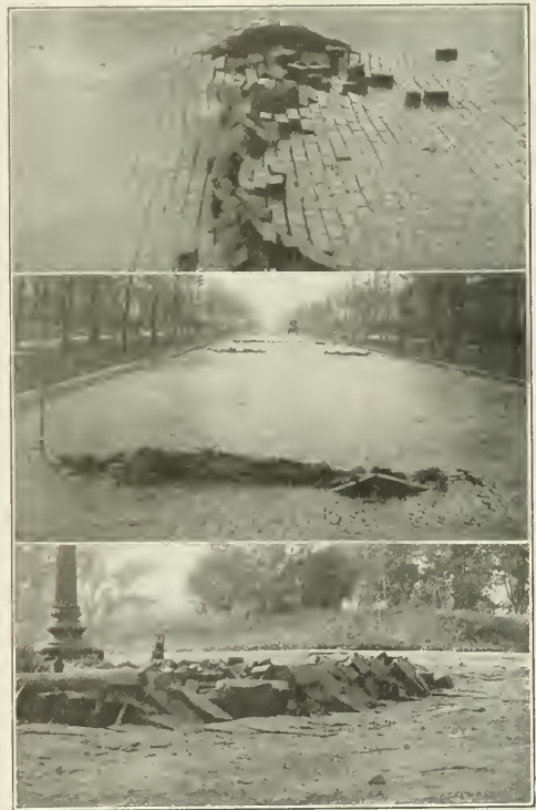
VIEWS SHOWING BULGING OF TAR-AND-OIL TREATED BLOCK PAVEMENTS, INDIANAPOLIS, IND.
