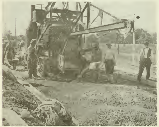
SPRINKLING SUB-GRADE PREPARATORY TO PLACING CONCRETE
