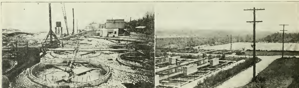
LEFT: VIEW OF ACTIVATED SLUDGE AERATING TANKS, MILWAUKEE WIS. RIGHT: VIEW OF IMHOFF TANKS AND TRICKLING FILTERS AT FITCHBURG, MASS.
