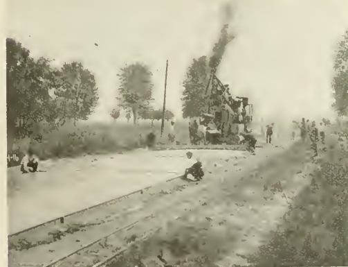
FINAL FINISHING WITH A CANVAS BELT ON WAYNE COUNTY CONCRETE ROADS.
