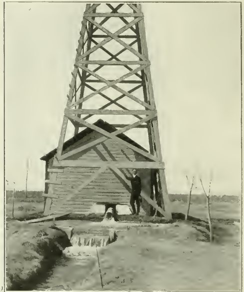
IRRIGATION PUMPING STATION AT PLAINVIEW, TEXAS. PUMP IS AMERICAN 24 IN., 2-STAGE, DEEP WELL CENTRIFUGAL BELTED TO OIL ENGINE, DELIVERING 1,500 G. P. M. AGAINST TOTAL HEAD OF 75 FT.
