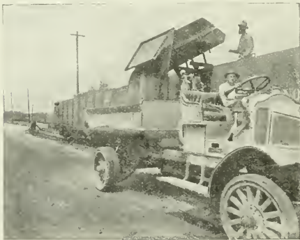
THE HELTZEL LIGHTNING LOADER SKIP AS OPERATED IN CONJUNCTION WITH MOTOR TRUCKS.
