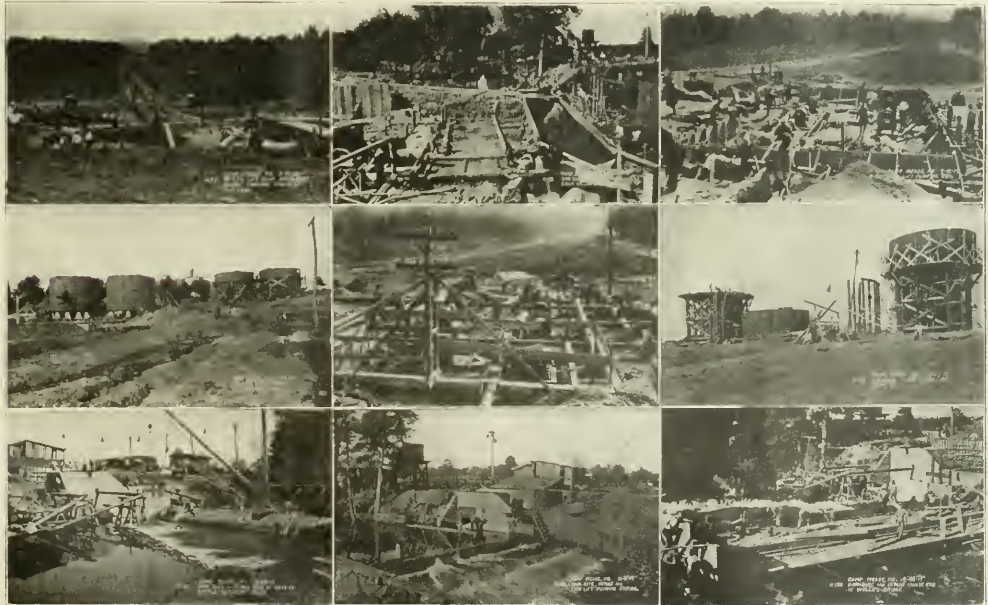
VIEWS SHOWING CONSTRUCTION OF CAMP MEADE, MD., WATER SUPPLY WORKS.
