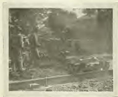
THE MECHANICAL TAMPING TEMPLATE CUTS OFF THE CONCRETE AND TAMPs IT TO UNIFORM DENSITY AND SMOOTH SURFACE. NOTE THE ROCKER-ARM WHICH TRANSMITS THE TAMPING MOTION. THE TEMPLATE IS DRAWN FORWARD BY THE WIRE ROPE WINDING ON THE DRUM
