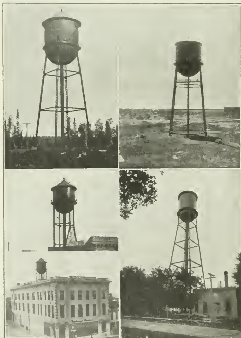
RECENT WATER TANKS WITH NOVEL FEATURES.
