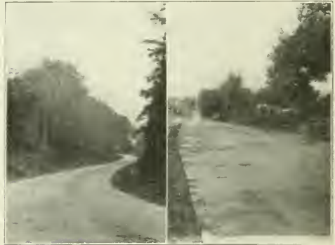
TYPICAL VIEWS OF CONCRETE ROADS IN WOOD COUNTY, W. VA.
