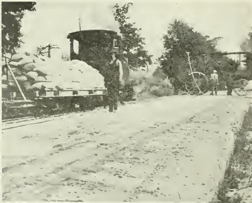
HAULING CEMENT UP 6 PER CENT. GRADE ON INDUSTRIAL RAILROAD.
