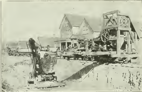
SPECIAL BACKFILLING MACHINE USED ON HEAVY SEWER CONSTRUCTION IN CHICAGO.
