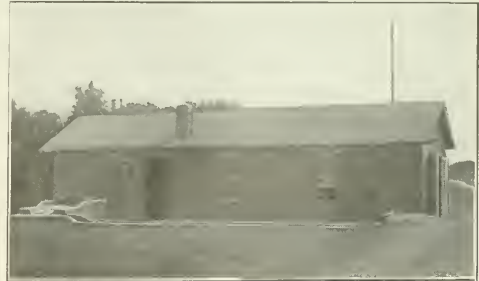
ONE OF TWO IRRIGATION PUMPING PLANTS IRRIGATING 240 ACRES NEAR LARNED, KANS.
