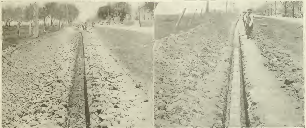
VIEWS SHOWING CONSTRUCTION OF TELEPHONE CONDUIT IN SUBURBAN DISTRICT.
