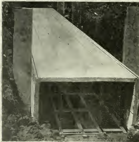
VIEW OF COLLAPSIBLE CULVERT FORM IN CONCRETING POSITION.
