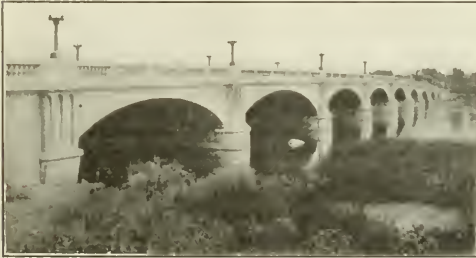
VIEW OF THE FRANKLIN STREET REINFORCED CONCRETE BRIDGE, WATERLOO, IA.
