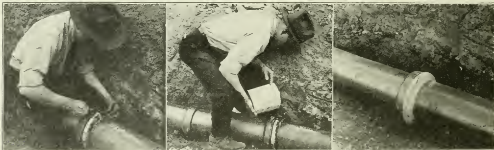
MODERN METHOD OF POURING JOINTS IN PIPE SEWER CONSTRUCTION.
