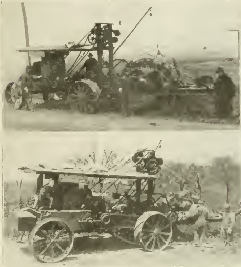
VIEWS OF TYPE 122 PAWLING & HARNISCHFEGER TRENCH EXCAVATOR DIGGING TRENCH FOR SUBURBAN TELEPHONE CONDUITS.
