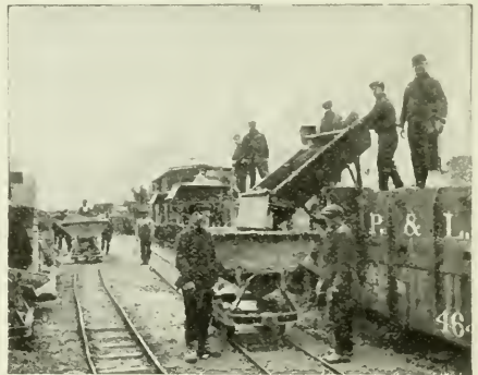
THE HELTZEL LIGHTNING LOADER SKIP AS OPERATED WITH INDUSTRIAL RAILWAY.
