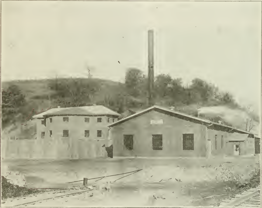
VIEW OF RECONSTRUCTED WATER WORKS PLANT AT FORT MADISON, IOWA. Pumping Station and Coal Storage on Right. Settling Basin, Filter House and Head House on Left.
