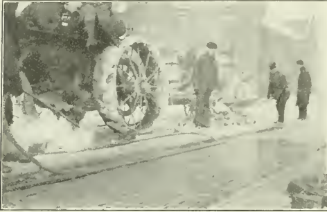
STEAMING SNOW FROM WOOD BLOCKS BEFORE APPLYING PITCH FILLER, TOLEDO, OHIO.
