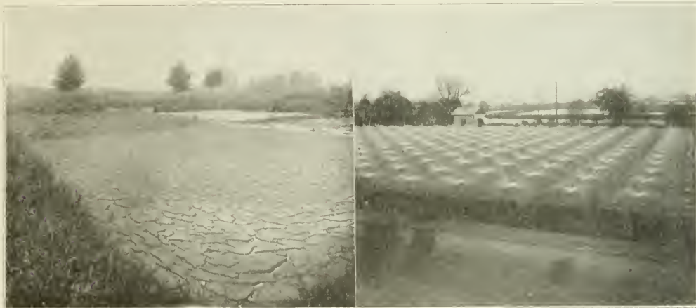
VIEWS OF SLUDGE DRYING BEDS AND TRICKLING FILTERS IN OPERATION, PHILADELPHIA, PA., SEWAGE TREATMENT WORKS.
