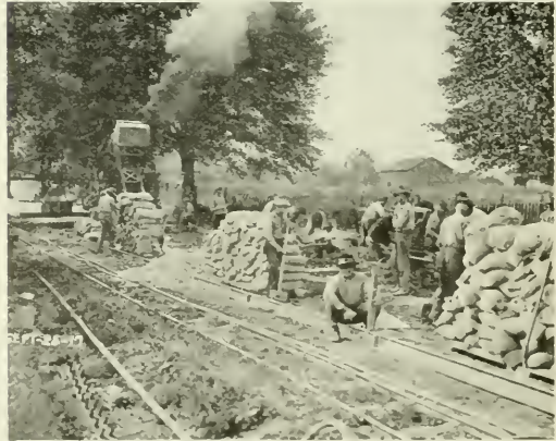
MATERIALS SPACED ON GRADE READY FOR MIXER.
