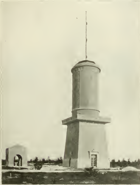
VIEW OF 100,000-GAL. REINFORCED CONCRETE WATER TANK AT ALTON BEACH, MIAMI, FLORIDA.
