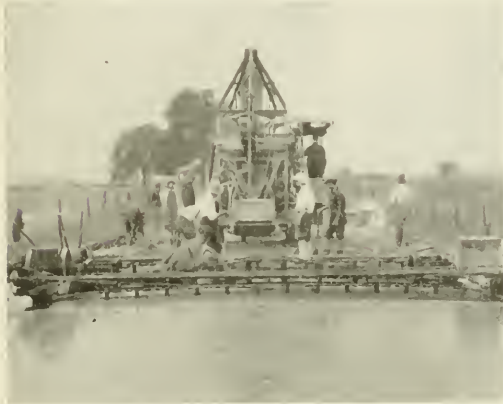
FINISHING MACHINE STRIKING OFF, FLOATING, LEVELING AND FINISHING SURFACE ON AN 18-FT. WAYNE COUNTY CONCRETE ROAD.
