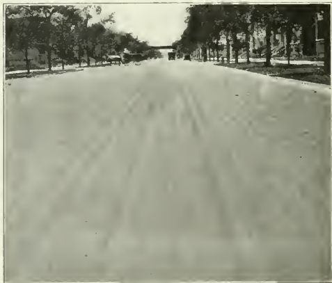
SHEET ASPHALT SURFACE SHOWING GROOVES PRODUCED BY LARGE VOLUME OF LIGHT MOTOR TRAFFIC.
