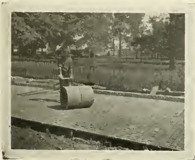
BRICK LAID AND ROLLED, READY FOR GROUTING WITHIN 25 FT. OF MIXER.
