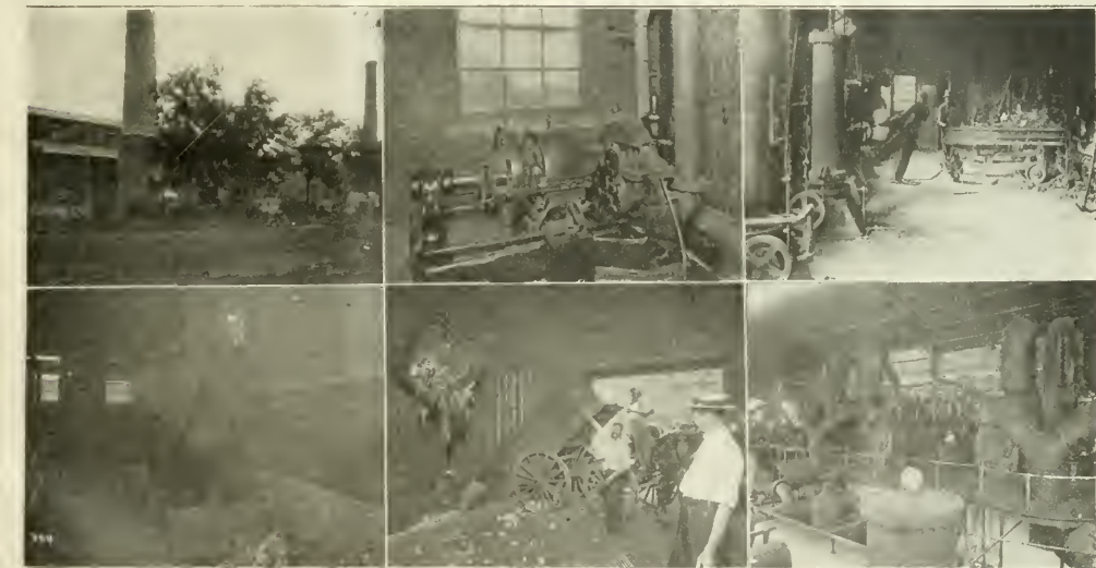
VIEWS OF REFUSE DESTRUCTOR, SAVANNAH, GA., IN SUCCESSFUL OPERATION FOR NEARLY FOUR YEARS.
