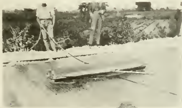
ROLLER FINISHING A CONCRETE ROAD.
