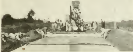
CONSTRUCTION OF LINCOLN HIGHWAY ON ELKHART-GOSHEN, IND. ROAD.
