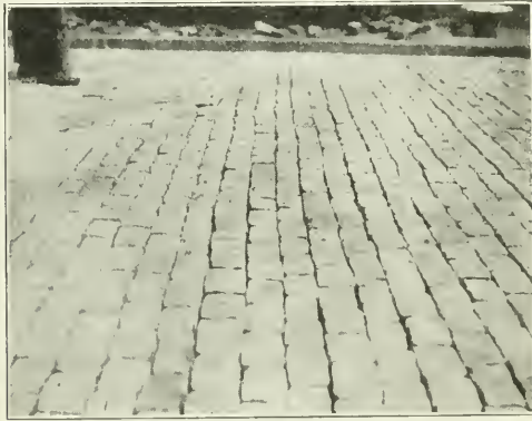
RECUT GRANITE BLOCKS LAID ACROSS CENTRAL PARK, NEW YORK CITY, READY FOR JOINT GROUTING.
