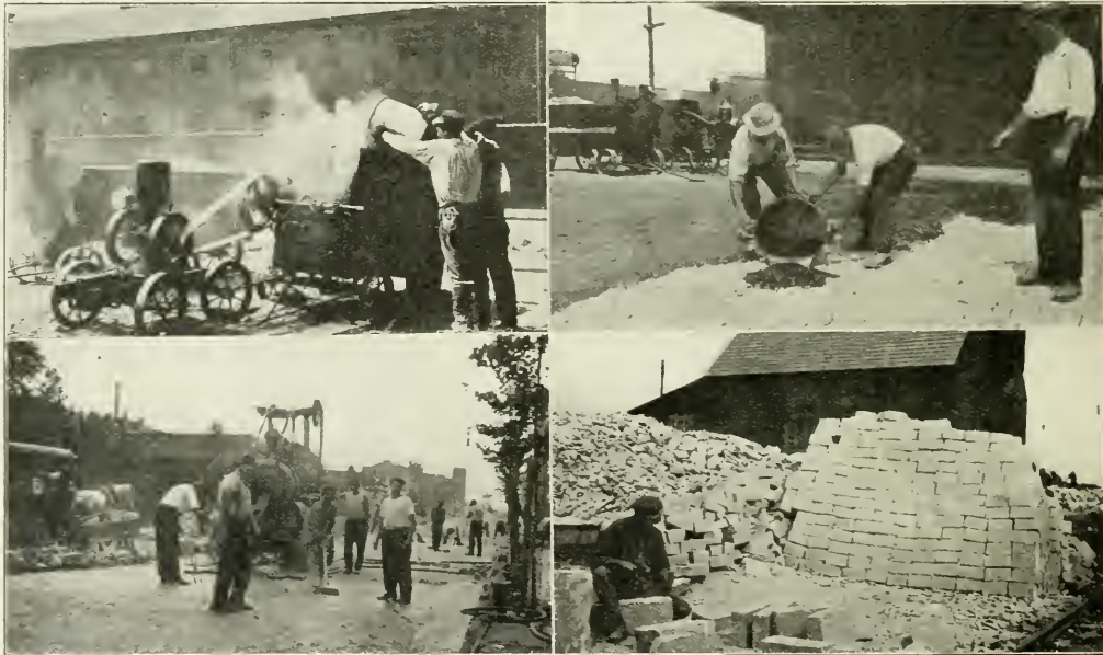
CONSTRUCTING THE MODERN GRANITE BLOCK PAVEMENT (LEFT TO RIGHT): MIXING BITUMINOUS FILLER AND SAND—POURING BITUMINOUS FILLER—GROUTING GRANITE BLOCK PAVEMENT—PILE OF WELL CUT GRANITE PAVING BLOCKS.
