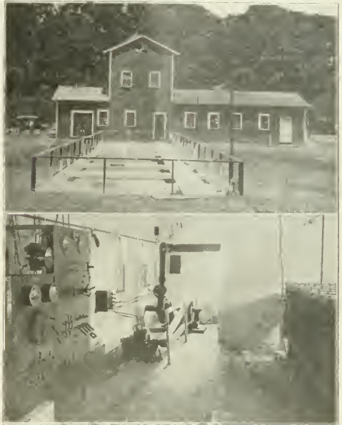
VIEWS OF ELECTRO-CHEMICAL EXPERIMENTAL SEWAGE TREATMENT PLANT AT DECATUR, ILL.
