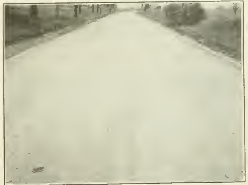
VIEW OF ASPHALT-ON-CONCRETE BASE ROAD BUILT ON BUSTLETON AVE., BY PHILADELPHIA BUREAU OF HIGHWAYS.
