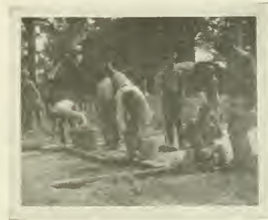
A SMOOTH SURFACE IS PREPARED FOR LAYING BRICK.
