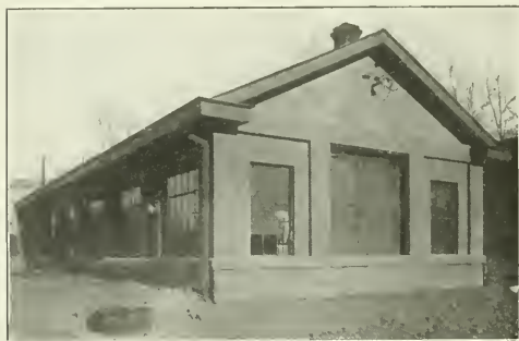
EXTERIOR VIEW REINFORCED CONCRETE LOW SERVICE PUMP STATION, GREAT FALLS, MONTANA, WATER PURIFYING AND SOFTENING PLANT.
