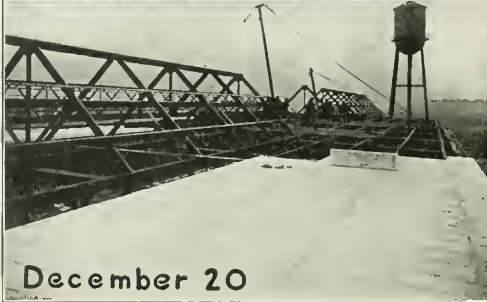
VIEWS SHOW RAPID PROGRESS IN FIREPROOF ROOF CONSTRUCTION ON A CHICAGO BUILDING.
