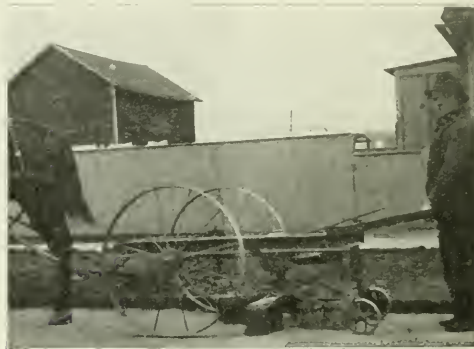
SAND SWEEPING MACHINE USED ON PAVEMENT CONSTRUCTION.
