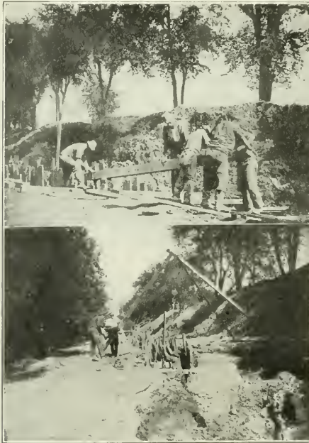
TWO METHODS OF PULLING SHEETING ON CHICAGO SEWER CONSTRUCTION.
