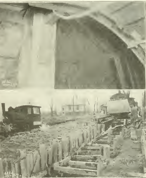
CONSTRUCTION VIEWS ON TUNNEL AND OPEN CUT SECTIONS OF 10-FT. SEWER IN LAKE ST., EVANSTON, ILL.
