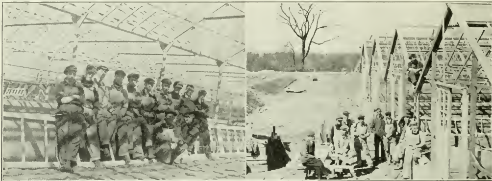
VIEWS OF GLASS COVERING OF GREEN-HOUSE TYPE OVER SEWAGE SLUDGE BEDS, ALLIANCE, OHIO. Rigid Steel Framework and Wood Sash Hinged at Top and Connected to Operating Apparatus.
