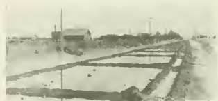
CURING A GREEN CONCRETE ROAD BY THE PONDING METHOD.
