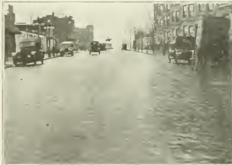
VIEW OF NEW GRANITE BLOCK PAVEMENT ON BEDFORD AVE., BROOKLYN, SOUTH FROM ST. JOHNS PLACE
