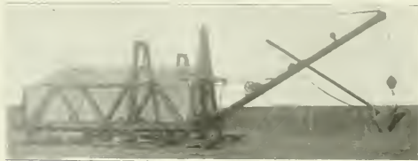
NEW BAY CITY LAND DREDGE OF THE WALKING TYPE.
