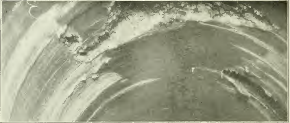
STALACTITES AND DISINTEGRATION IN THE CROWN OF THE SEWER.
