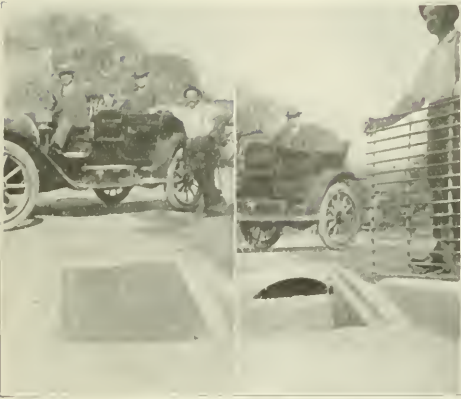
LEFT: GRATING OVER CATCHBASIN AND ENTRANCE TO DRAIN UNDER STREET INTERSECTION. RIGHT: GRATING REMOVED, SHOWING BASIN AND END OF PART-CIRCLE CULVERT.
