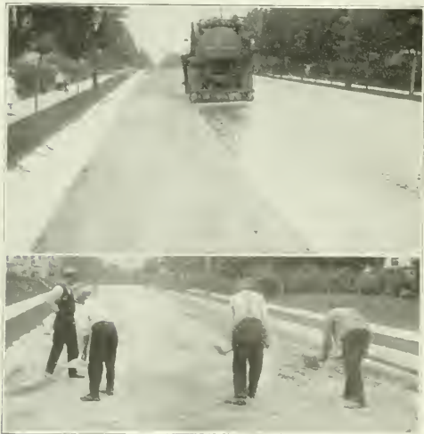
ABOVE: APPLYING BITUMINOUS MATERIAL WITH AUTO PRESSURE DISTRIBUTER.
