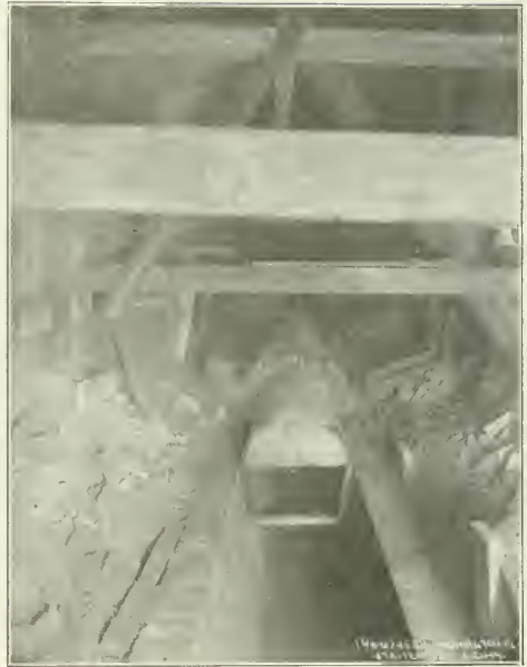
TWO-RING EGG-SHAPED SEWER. INVERT COMPLETED. ARCH-FORM IN PLACE READY FOR WORK. A PIPE SEWER CONNECTION SET AT SPRINGING LINE READY FOR BRICKING INTO THE ARCH. NOTE METHOD OF SUPPORTING ARCH FORM ON SIDEWALLS OF INVERT.
