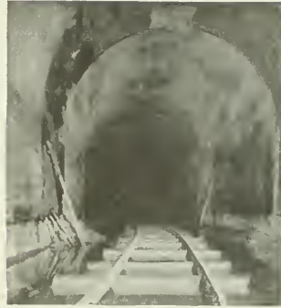
COMPLETED AND LINED SECTION, MILL CREEK TUNNEL.
