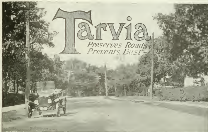
Everett Avenue, Winchester, Mass. Constructed with "Tarvia-X" in 1915. Treated with "Tarvia-B" in 1916.
