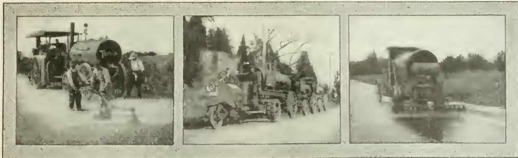
DISTRIBUTING TARVIA ON WEARING SURFACE.
