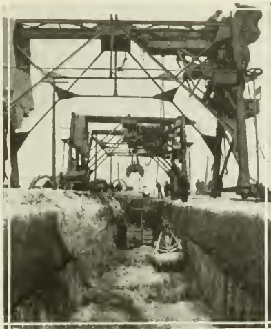
VIEW OF TRENCH, SHOWING THE SHEET PILING AND TWO ELECTRIC CRANES.
