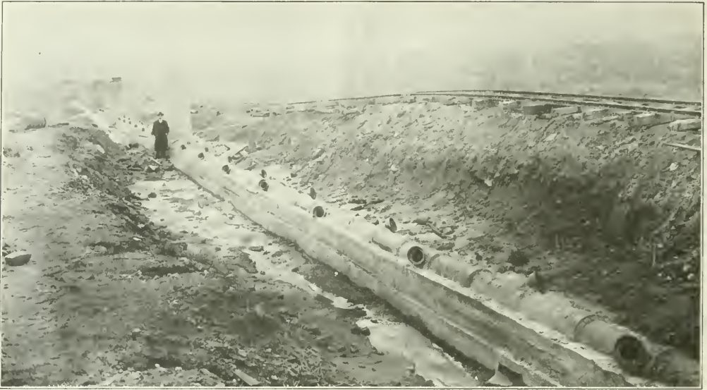
VITRIFIED SEWER ON CONCRETE FOUNDATION ON A MARSH NEAR SALT MARSH, BORO OF BRONX, NEW YORK.
