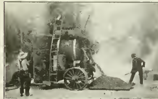
2—Discharging stone mixed with hot Tarvia.
