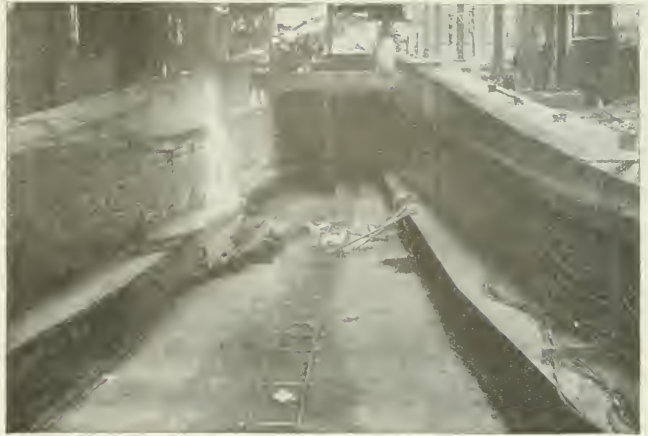
GENERAL VIEW, VAN BUREN STREET TUNNEL ALTERATION.
