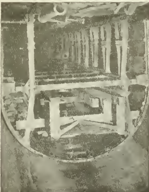
PORTABLE STEEL CONCRETE FORMS IN PLACE. BRACING FOR THE ARCH.
