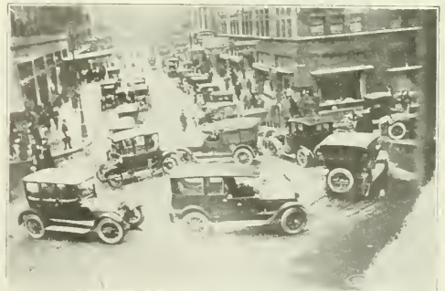
PLATE VI. A small rotary traffic circle at Grand River avenue and Farmer street, Detroit, Michigan, which has eliminated the traffic officer formerly stationed there. While this circle may always be busy, foot passengers have little trouble in crossing any of the four streets, especially if a traffic separator or isle of safety is placed in the middle of each, just outside the rotary traffic circle.
