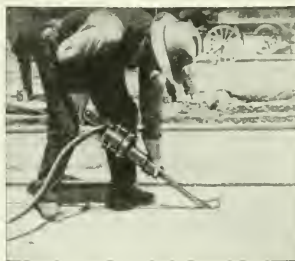
LINING THE ASPHALT WITH CHANNELING BIT.
