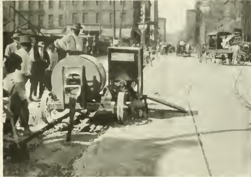
CONCRETE MIXER DISCHARGING DIRECT INTO PAVEMENT CUT.
