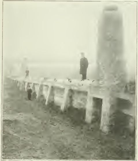
VITRIFIED SEWER ACROSS SALT MARSH IN SHALLOW TRENCH, BORO OF BRONX, NEW YORK.
