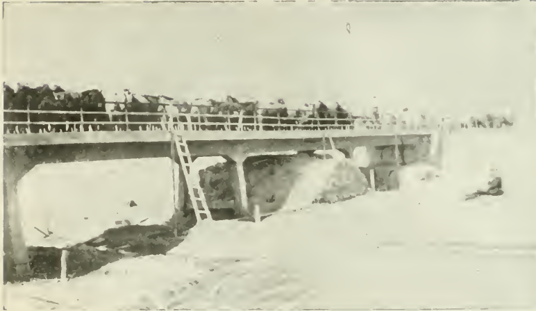
LOADING TESTS ON KAHN SYSTEM BRIDGE.
