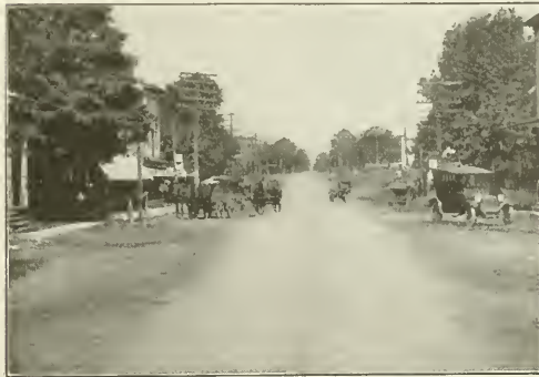
Main Street, Covert, Michigan. Sixteen feet in center treated with "Tarvia-B."
