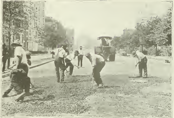
LAYING BITULITHIC SURFACE OVER OLD MACADAM, COMMONWEALTH AVENUE, NEAR CHARLES GATE WEST, 1916.
