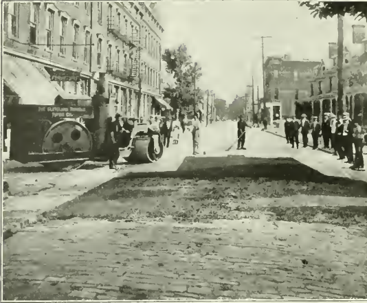
RESURFACING OLD GRANITE BLOCK PAVEMENT WITH ASPHALT ON THIRTIETH STREET NORTH OF MT. VERNON STREET, COLUMBUS, O., 1915.
