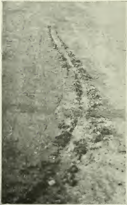
FIG. 2. BLEEDING ON A LIGHT TRAFFIC STREET. THE OIL FILLER, AND SURFACE COVER OF SAND HAVE FORMED A COMPARATIVELY NON-ADHESIVE MASS ON THE PAVEMENT THAT IS OVER 2\frac{1}{2} INCHES THICK AT THE POINT PHOTOGRAPHED.
