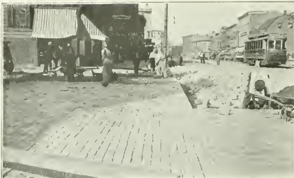
STRAIGHT COURSES AND NARROW JOINTS ARE EASY TO OBTAIN.
