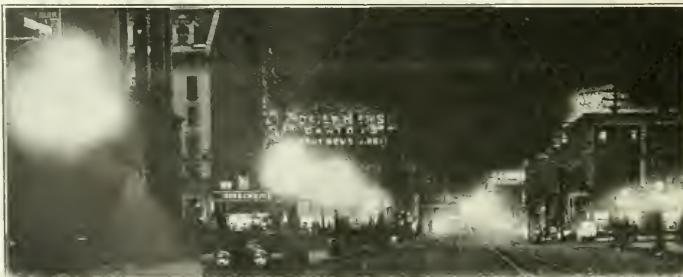
ORNAMENTAL GAS STREET LIGHTING.
