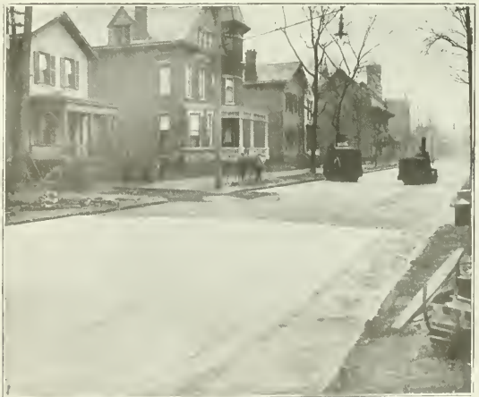
SHEET ASPHALT SURFACING OVER OLD BRICK PAVEMENTS ON SIXTH STREET, COLUMBUS, O., 1½-INCH BINDER AND 1½-INCH TOP, 1912.
