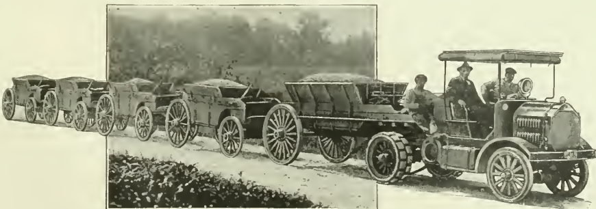
KNOX TRACTOR AS OPERATED BY PETERS & BAIRD, WADSWORTH, O. HAULING SEMI-TRAILER AND FOUR DUMP WAGONS (BOTTOM DUMP) ON SIX-MILE HIKE.
