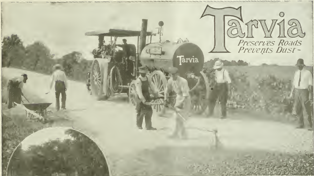
The illustration shows "Tarvia-X" being applied under pressure on the wearing-course—at this step the road is about half constructed. The view in the circle is the finished road at Green Lake, Wis. Note that the speeding auto leaves no trail of dust.
