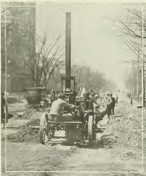
P. AND H. TRENCH TAMPER AT WORK COMPACTING A SEWER TRENCH.
