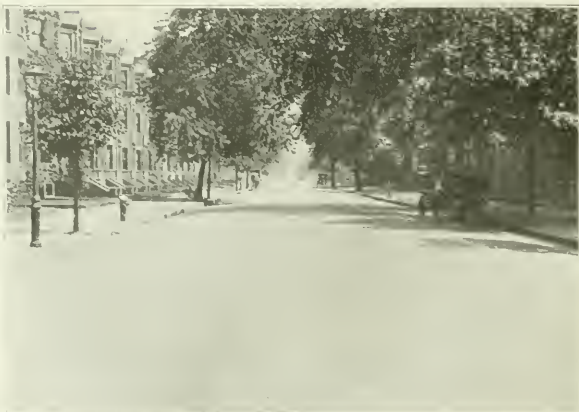
BITULITHIC PAVEMENT IN MARLBORO STREET EAST OF MASSACHUSETTS AVENUE, LAID OVER OLD MACADAM IN 1914.
