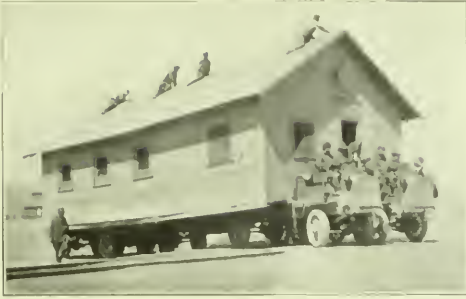
FOUR E. W. D. TRUCKS AS OPERATED TO MOVE NATIONAL GUARD COMPANY HOUSE DISTANCE OF 7½ MILES AT CAMP STEWART ON MEXICAN BORDER.
