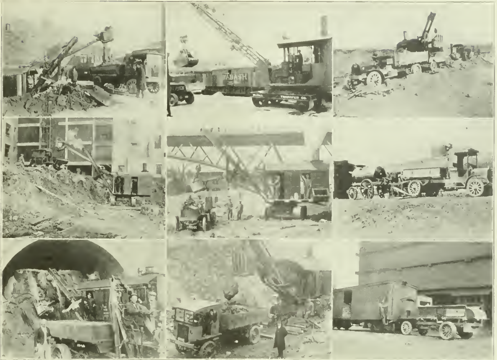
GARFORD, PACKARD AND U. S. MOTOR TRUCKS AS OPERATED IN CONJUNCTION WITH STEAM SHOVELS, CRANES AND OTHER TYPES OF MACHINERY BY CONTRACTORS IN NEW YORK, CHICAGO, LOS ANGELES, ALBANY, PHILADELPHIA, BROOKLYN AND HANNIBAL. (FULLY DESCRIBED IN THIS ISSUE.)
