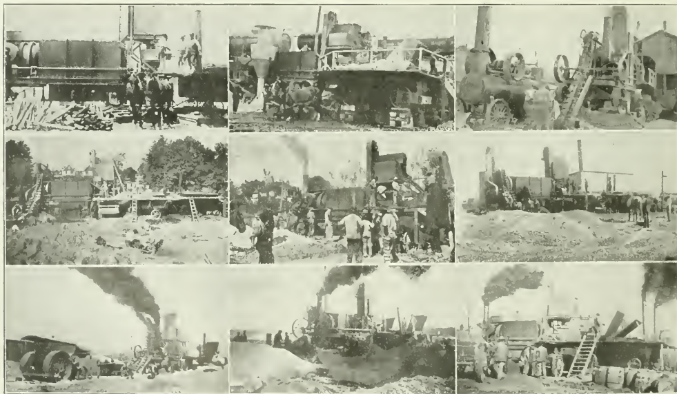
CUMMER PORTABLE ROAD ASPHALT PAVING PLANTS IN OPERATION.
