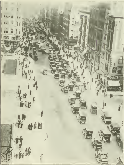
PLATE IV. Illustration of block system, showing congestion behind block and vacant street space before it, thus using but half the street at a time and increasing rather than distributing the density of traffic along the street.
