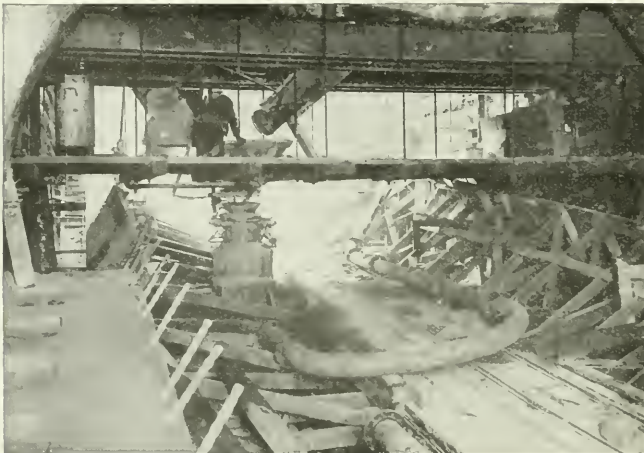
PNEUMATIC CONCRETE EQUIPMENT IN THE VAN BUREN STREET TUNNEL.
