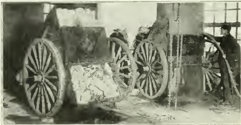
A SANITARY GARBAGE CART SUCH AS SHOULD BE USED, WHETHER TWO OR FOUR-WHEELED. GARBAGE WRAPPED IN PAPER, AS SHOWN HERE, IMPROVES SANITARY CONDITION IN GARBAGE CAN AND IN COLLECTION. AT THE RIGHT A CART IS BEING WASHED BY STEAM BEFORE STARTING FOR ANOTHER LOAD.
