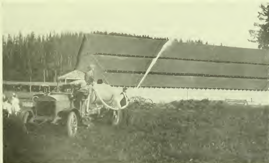
G. M. C. 2-TON TRUCK AS OPERATED IN ROAD SPRINKLING, TREE SPRAYING AND FIRE FIGHTING. CAPACITY 3 BARRELS PER MINUTE.
