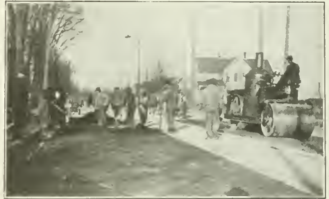
LAYING ASPHALTIC CONCRETE ON THIRD STREET, DEPERE, WIS. WILLISTON CONSTRUCTION CO.
