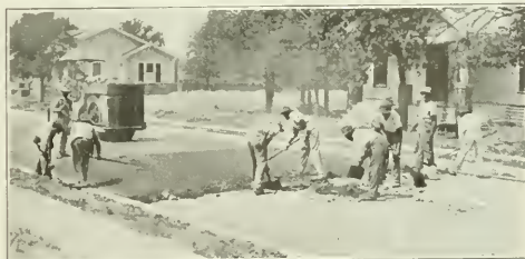
RESURFACING OLD BRICK PAVEMENT WITH ASPHALT. AUSTIN MOTOR ROLLER IN BACKGROUND.
