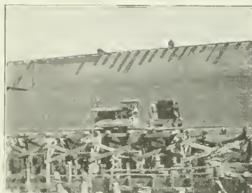
NOTE LOCOMOTIVES RUNNING ALONG TRESTLE—OHIO RIVER DAM 48 JOB.
