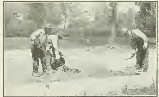
6—Applying squeeze coat of Tarvia and covering with fine stone.
