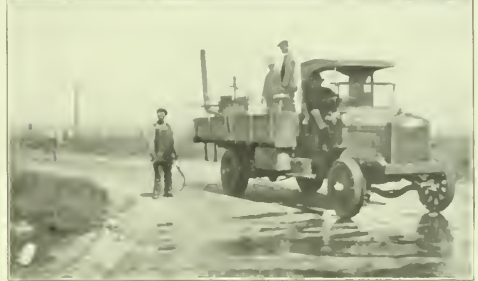
ONE OF SEVEN 1-TON MORELAND TRUCKS AS OPERATED ON ROAD MAINTENANCE BY LOS ANGELES COUNTY, CAL.
