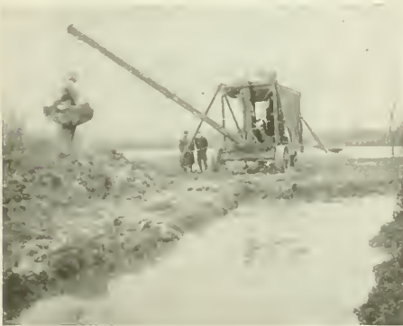
DIGGING DRAINAGE DITCH IN INDIANA. M. W. HOLBEN, GARY, IND.
