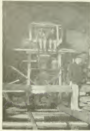
HOPPER AT FOOT OF WELL DRILL HOLE FROM SURFACE, AND PNEUMATIC CONCRETE MIXER.
