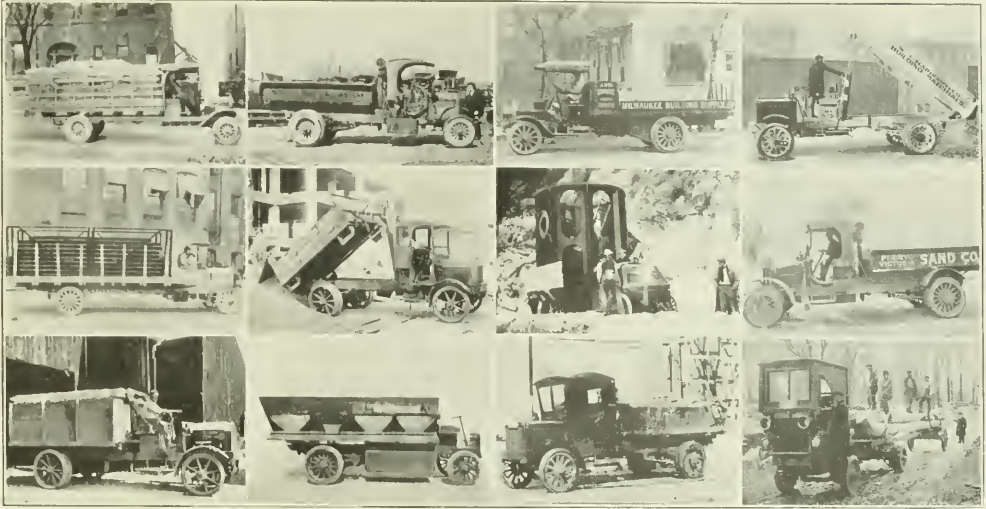
MOTOR TRUCKS AS USED IN BUILDING AND BRIDGE CONSTRUCTION.
