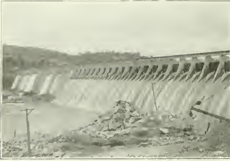
2. THE FINISHED AUSTIN DAM, SHOWING THE DOWN-STREAM FACE. THE LARGE CREST GATES ARE SEEN, CLOSED. THEIR SUPPORTING PIERS, WHICH ARE EXTENSIONS OF THE TRANSVERSE WALLS IN THE DAM ITSELF, SUPPORT THE CONCRETE BRIDGE ABOVE.
