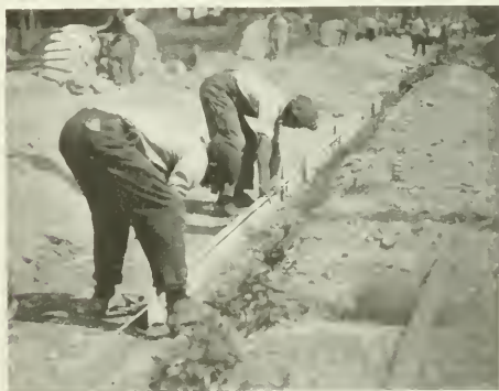
SETTING BAKER INDESTRUCTIBLE SIDE FORMS.
