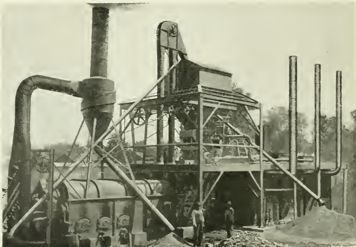
SEMI-PORTABLE HETHERINGTON AND BERNER ASPHALT PAVING PLANT, SAME DESIGN AS THAT FURNISHED FOR THE MUNICIPAL PLANT AT FLINT, MICHIGAN.
