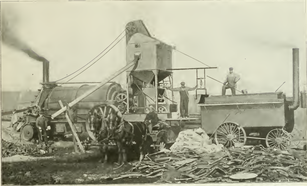
PORTABLE ROAD ASPHALT PLANT CONSTRUCTED BY HETHERINGTON AND BERNER, WHICH CAN READILY BE ADAPTED FOR BITUMINOUS MACADAM, ASPHALTIC CONCRETE, ASPHALT BINDER OR TOP, FIBERED ASPHALT OR ANY OTHER DESIRED MIXTURE.
