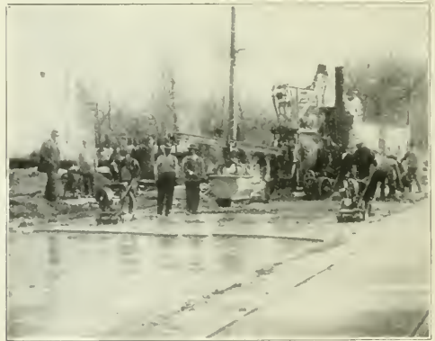
KOEHRING PAVER AND PATENTED GASOLINE ENGINE VIBRATOR AS USED IN CONSTRUCTING A VIBROLIOTHIC PAVEMENT AT WHITE LAINS, NEW YORK.
