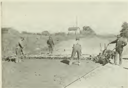
FINISHING MACHINE ON WAYNE COUNTY ROADS, DETROIT. BAKER SIDE FORMS AND ARMOUR PLATE USED.
