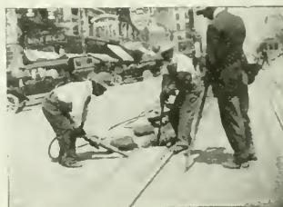
REMOVING THE ASPHALT WITH DRILL AND GAD.
