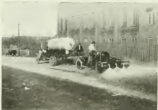
FIG. 1.—FINLEY METHOD SPRAY BINDER ON FRESHLY CLEANED ROADBED.
