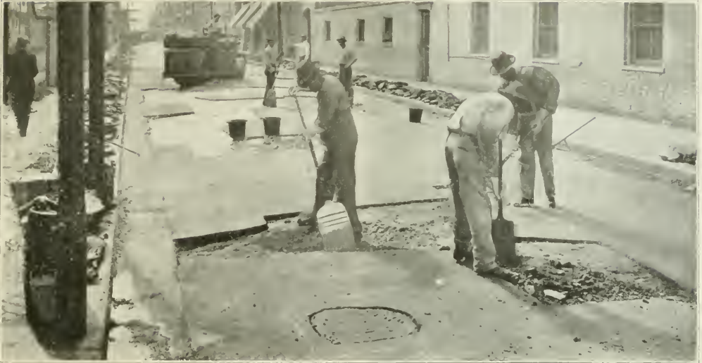
PROPER METHOD OF PREPARING ASPHALT STREET FOR PATCHING. PAINTING EDGES WITH ASPHALT CEMENT IN MIDDLE GROUND. AUSTIN MOTOR ROLLER IN REAR.
