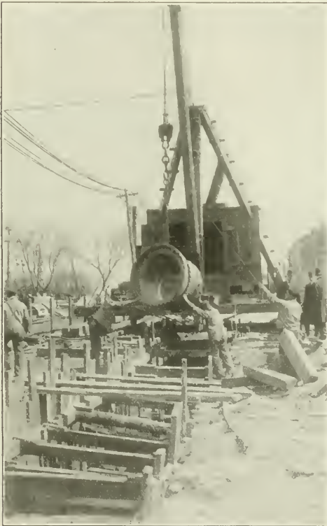
LOWERING LARGE SEWER PIPE INTO PLACE, BORO OF BROOKLYN, NEW YORK.
