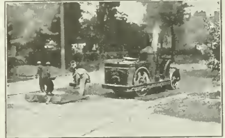
5—Rolling down the mixture with roller
