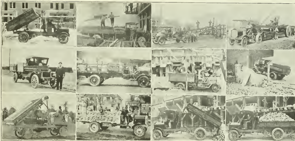
MOTOR TRUCKS AS USED IN BUILDING AND BRIDGE CONSTRUCTION.
