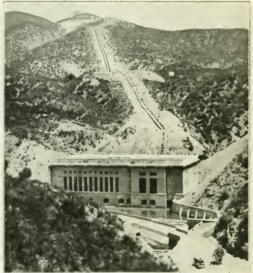
SAN FRANCISQUITO POWER HOUSE NO. 1, SHOWING ALSO THE PENSTOCK LINE AND THE SURGE TANK. THREE OF THE SIX UNITS HAVE BEEN INSTALLED AND FURNISH 37,500 HORSE POWER, PEAK LOAD.
