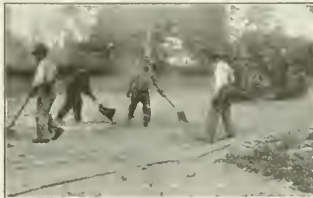
3—Spreading the soft, hot mixture in place.
