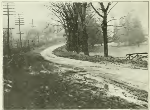
MORRISTOWN.—MENDHAM ROAD, WEST OF MORRISTOWN, N. J. EFFORT SEEMS TO HAVE BEEN EXPERTED HERE TO KEEP WATER ON THE ROAD RATHER THAN KEEP IT OFF, TO THE RUIN OF THE ROAD.
