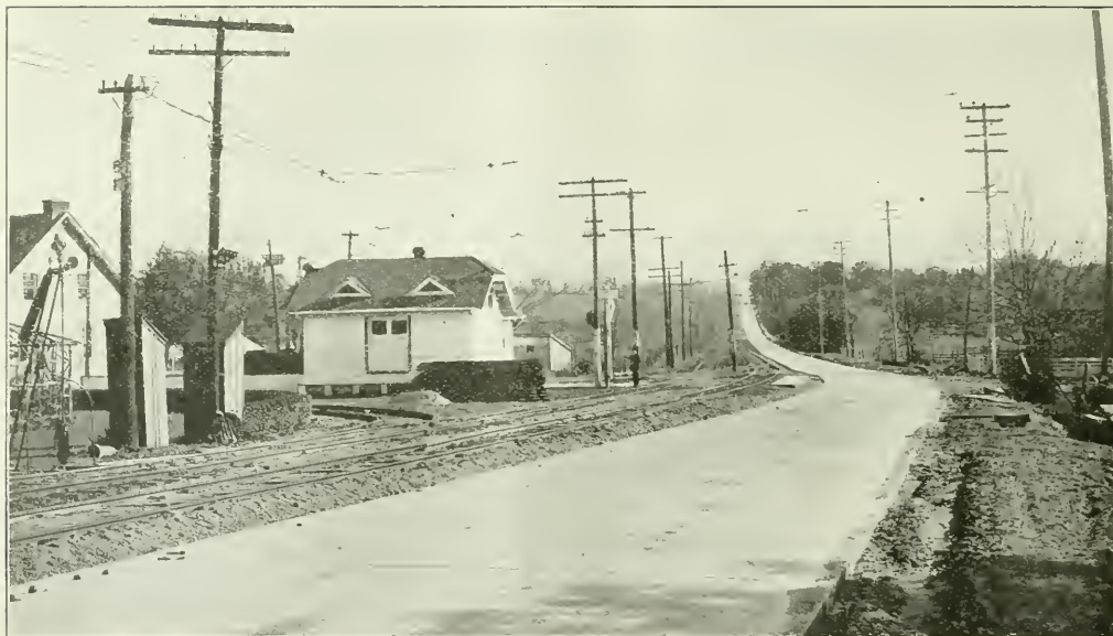
MACHINE FINISHED CONCRETE ROAD. BLOOMFIELD HILLS, WOODWARD AVE., NORTH OF DETROIT.
