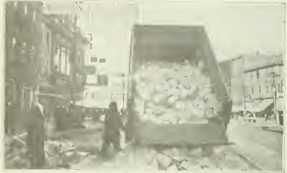
DUMPING GRANITE BLOCKS IN THIS WAY SAVES CHIPPING.
