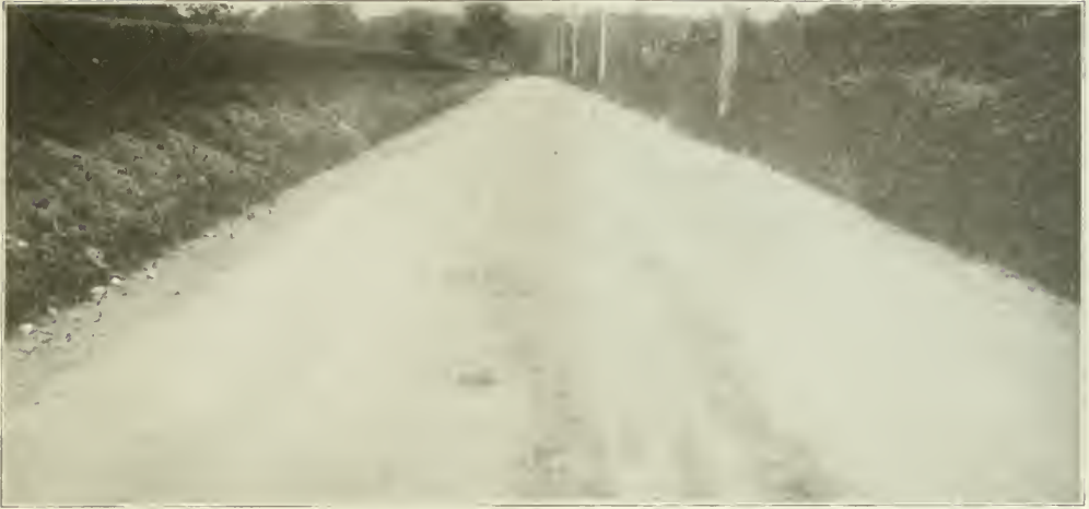
WATER-BOUND MACADAM ROAD WITH BITUMINOUS SURFACE TREATMENT, PHILADELPHIA, PA.
