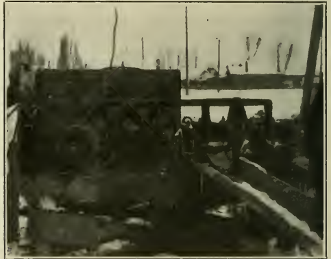
DOUBLE DIAPHRAGM PUMP electrically driven, pumping water from sewer trench, Salt Lake City, Utah.
