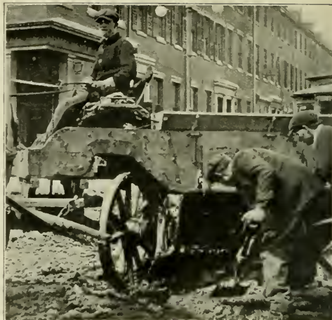
DUMPING AND SHOVELING SNOW INTO SEWER MANHOLE.
