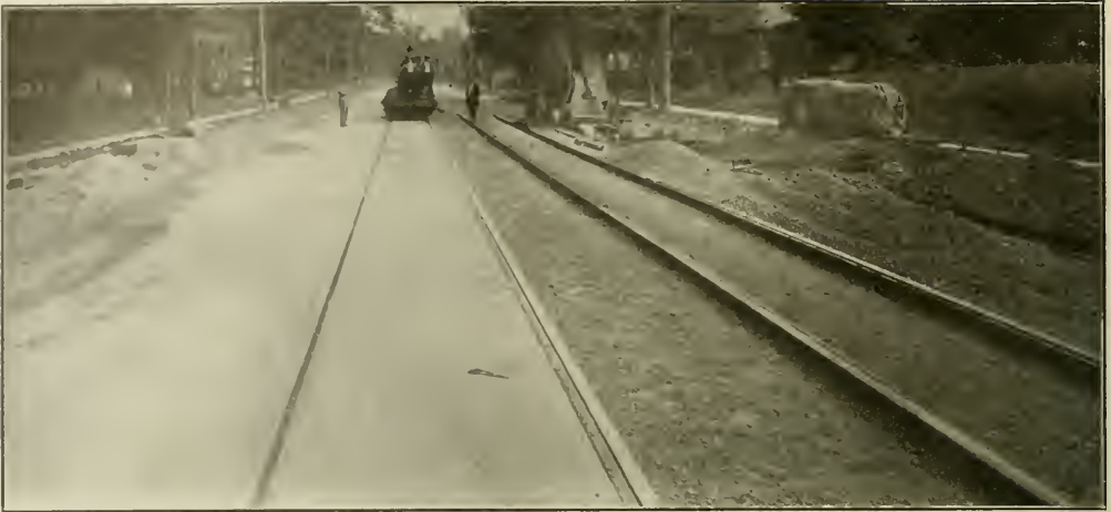
PELHAMDALE AVENUE concrete road. Concrete surface on half the road before bituminous top dressing was applied. Double track street railroad.
