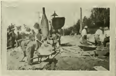
MIXING THE FOUNDATION.
