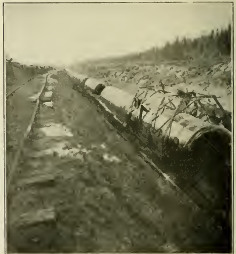
HANDLING FORMS BY TRAVELER, as done on three contracts. The concrete, mixed in a central plant, is delivered from cars by the railroad on the side of the trench, thru chutes into the forms.
