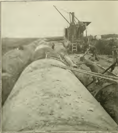
PLACING OUTSIDE FORMS in foreground with traveling derrick. The concrete mixing plant is seen on the track, ready to deposit concrete thru chute into the outside forms when all in place.
