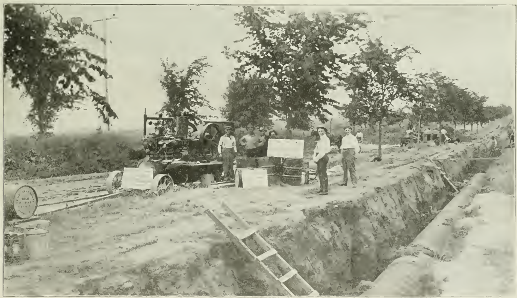
CHICAGO'S PNEUMATIC Portable Gasoline Driven Compressor used in construction of filtration plant by city of Minneapolis, Minn.
