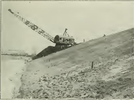
SLOPING AND FINISHING LEVEE BETWEEN BELT RAILROAD AND BELMONT AVENUE, NEAR NORTH END OF WORK. CONTRACTOR KEARN'S BIG DRAG LINE EXCAVATOR AT WORK. THE ORIGINAL GROUND FOUNDATION IS SEEN NEAR THE MACHINE, THE TOP OF THE LEVEE AT THE RIGHT AND THE FINISHED SLOPE IN THE FOREGROUND. THE EXCAVATOR TOOK MATERIAL FROM THE AREA AT THE LEFT WITH WHICH TO BUILD THE LEVEE, AS WELL AS THAT GRADED OFF THE BANK. BELT RAILROAD BRIDGE AT LEFT IN BACKGROUND.
