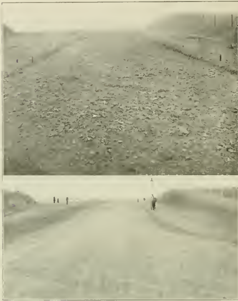
QUINCY SHORE BOULEVARD, CUT AT SAILORS' HOME HILL.
