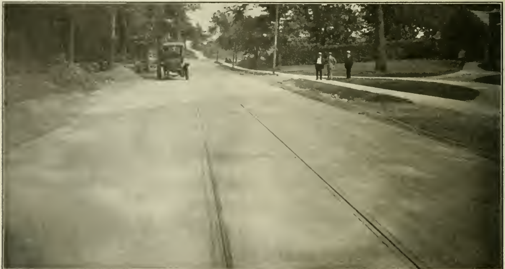
PELHAMDALE AVENUE concrete road, single track street railroad. Concrete completed, but bituminous top dressing not yet applied.
