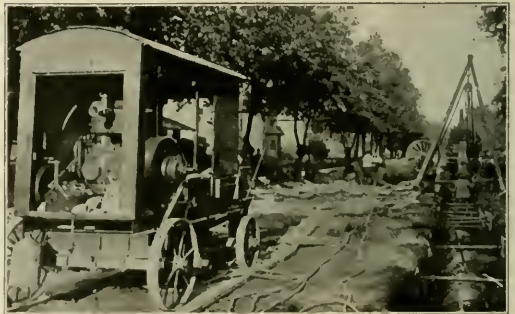
GARDNER PORTABLE AIR COMPRESSOR ON CHICAGO CALKING JOB.
