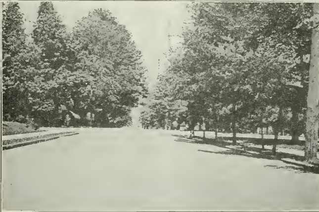
Portland, Oregon. Bitulithic Pavement, W. Park Street. Laid over old Macadam, 1913. Photograph taken May, 1915.
