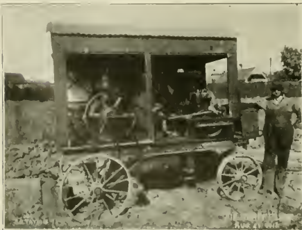
GARDNER PORTABLE AIR COMPRESSOR ON CHICAGO CALKING JOB.
