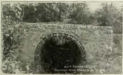
LARGE HIGHWAY CULVERT OF SEGMENTAL BLOCKS.
