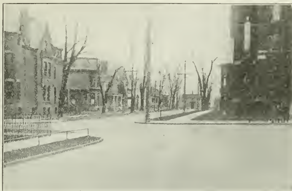
Bitulithic Pavement. Intersection N. Main and Church Sts., Court St. in background, Herkimer, N. Y. Church St. laid on 4-inch Concrete base 1908.
