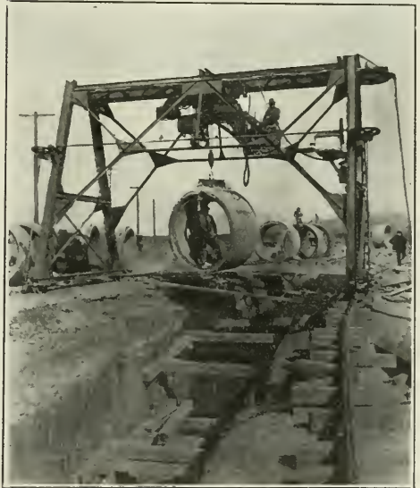
NEAR VIEW OF THE PIPE-LAYING CRANE showing electric hoist and a pipe on its way to the bottom of the trench.
