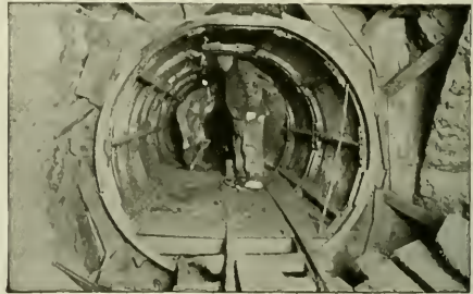
BLAW tunnel form on 76-inch full round tunnel; James Hanreddy, Chicago, Ill., Contractor.
