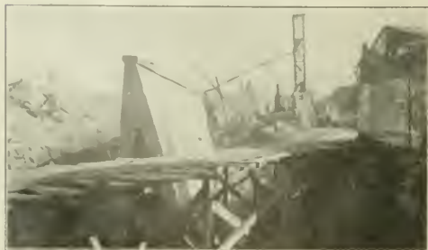
VIEW OF WALL UNDER CONSTRUCTION FROM DIRECTION OPPOSITE TO THAT OF THE PRECEDING PHOTOGRAPH. COMPLETED WALL IN FOREGROUND, SHOWING RECESS IN END TO AID IN BONDING WITH THE NEXT SECTION. CONCRETE MIXER, WITH ELEVATOR TOWER AND CHUTE BUILDING WALL, FARTHER BACK. IN BACKGROUND IS OUTFIT LAYING CONCRETE FOOTING ON WHICH THE WALL IS TO BE BUILT.
