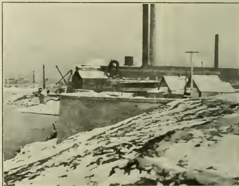
UPPER END OF CONCRETE RETAINING WALL AT STREET CAR PLANT, SHOWING CURVE TO CONNECT WALL WITH LEVEE, RIVER SLOPE OF WHICH IS IN THE FOREGROUND. REVERSE CURVE IN WALL IS SHOWN IN THE CORNER OF THE COPING. WALL CONSTRUCTION IN PROGRESS IN BACKGROUND.
