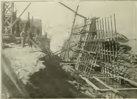
BUILDING THE CONCRETE RETAINING WALL ON THE FOOTING SHOWN IN PRECEDING PHOTOGRAPH. STEEL FRAMES FOR FORMS IN FOREGROUND, WITH COMPLETED FORMS FARTHER BACK, AND COMPLETED WALL STILL FARTHER BEYOND. NOTE THE CABLES NECESSARY TO PREVENT THE FORMS MOVING TO THE RIGHT WHEN FILLED WITH CONCRETE.
