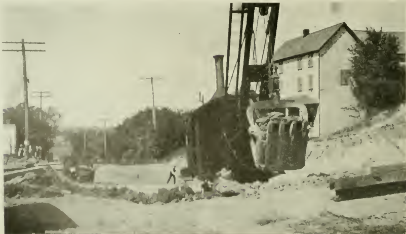
SHOVEL IN SHALLOW EXCAVATION. Clinton Contracting Co., Contractors.
