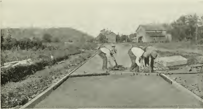
Showing the facility with which Pittsburgh Paving Joint can be laid. Note the absence of melting tank and other cumbersome apparatus
