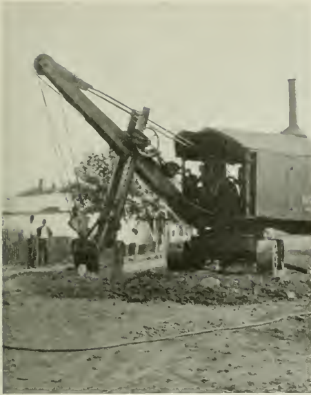
SHOVEL IN SHALLOW EXCAVATION. Maryland State Roads Commission. Barker & Bonner, Inc., N. Y., Contractors.
