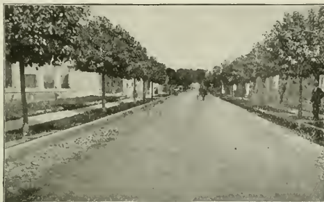
View 1—Looking down General Lee Street from intersection of Dolores Street, Marianao, Cuba. View taken April 1915. Plain macadam laid in October 1914. Note destruction of gutters by tropical rains.
