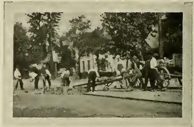
USING A GRAVITY BRICK CARRIER.
