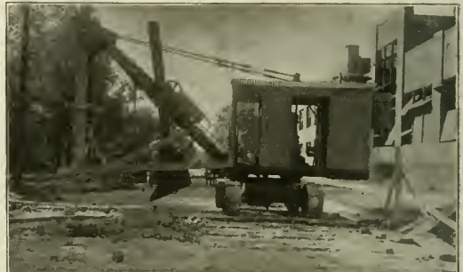
ERIE SHOVEL on shallow excavation encountered in road construction.
