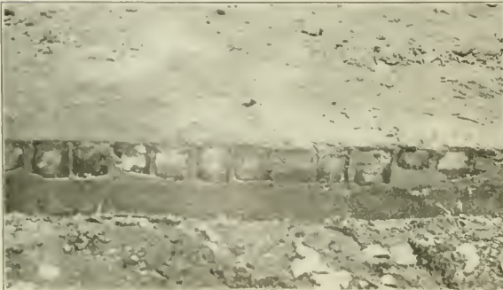
GROUT FILLER is shown extending to bottom of brick, thus bonding foundation and brick surface into a solid monolith.
