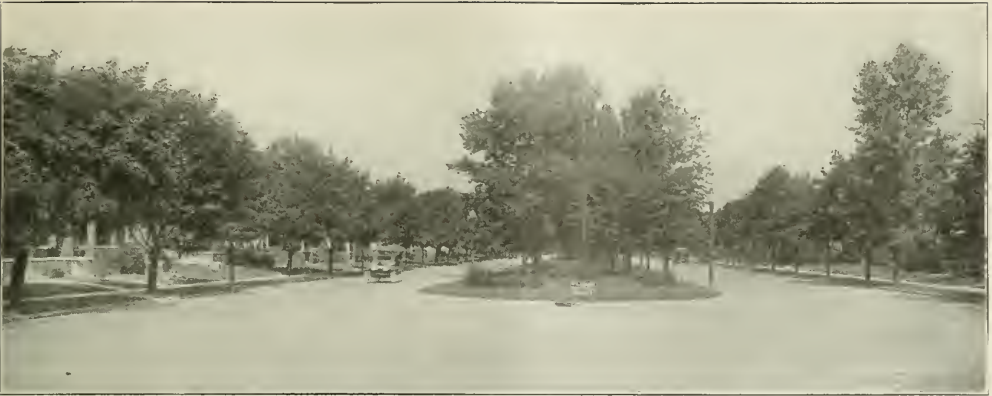
EAST GRAND BOULEVARD, DETROIT, MICHIGAN, A NOTABLE THOROUGHFARE PAVED WITH SHEET ASPHALT LAID BY THE MUNICIPAL ASPHALT PLANT DEPARTMENT.
