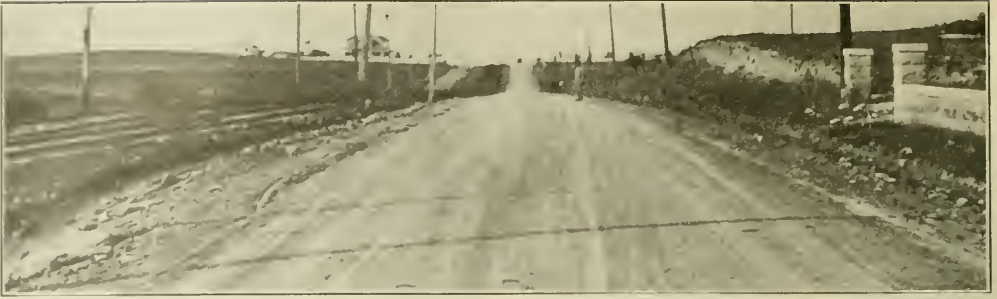
WEATHERFORD PIKE, a main county road of asphalt macadam, eighteen feet wide, constructed by the penetration method under Travilla's Class A specifications.
