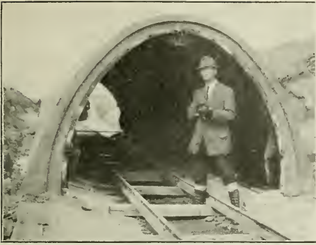
COMPLETED SECTION of plain concrete conduit, horseshoe form of section, where there is no internal water pressure. Note wooden strip water stop imbedded in the surface of the invert side of the joint between invert and arch; also the copper strip around the arch to prevent leakage thru the expansion joint provided at this point.
