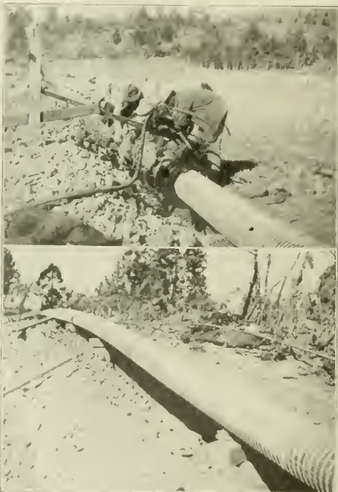
ELECTRICALLY WELDED WIRE-WOUND WOOD-STAVE PIPE.
