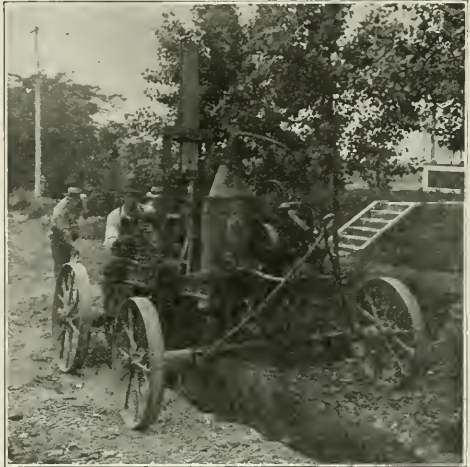
A TRENCH TAMPER THAT DOES NOT SOLDIER.
