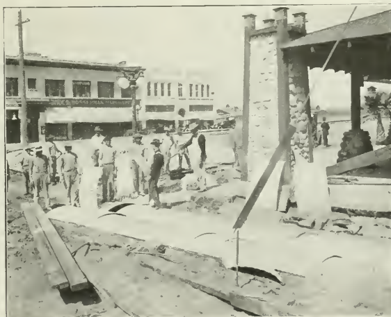
Installation of No. 10 Gauge, Corrugated Pure Iron Arches at Glendale, Calif.
