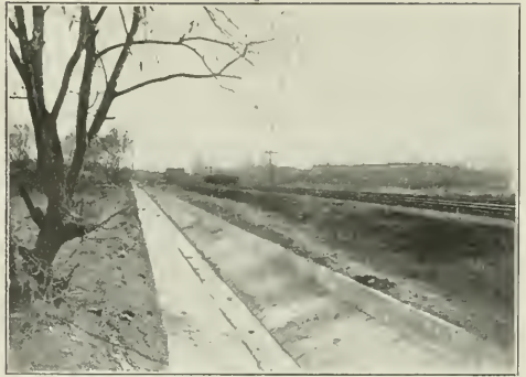
PAXTON CREEK after it had been regulated, giving a concrete-lined channel designed to carry the low-water flow and also the flood flow, and to be self-cleansing under both conditions. The section shown is along the railroad, but there is evident opportunity for beautifying the adjoining ground and thus giving the transient traveler on the passing train a pleasant memory of the city.
