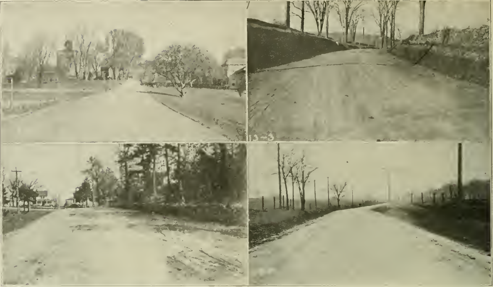
RED SHALE ROAD AT PRINCETON UNIVERSITY, NEW JERSEY; PROBABLY THE FIRST SUCCESSFUL SHALE ROAD BUILT IN THAT STATE, TREATED IN 1913.
