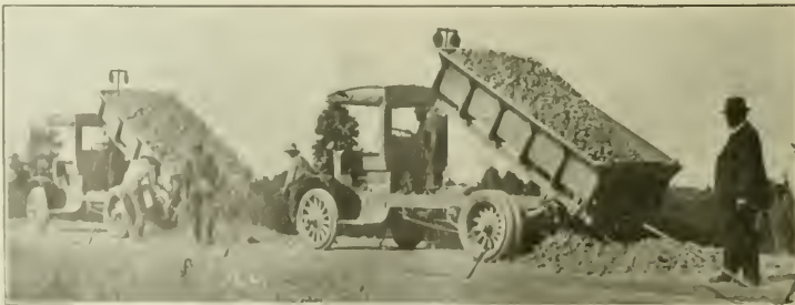
DELIVERING ROAD CONSTRUCTION MATERIAL BY MOTOR TRUCKS.
