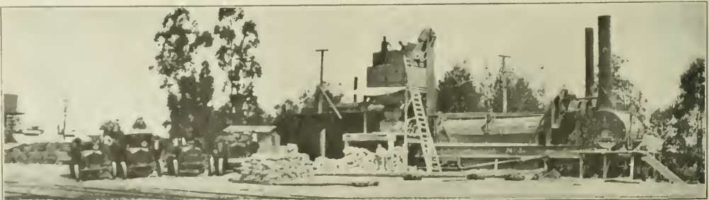
FRONT VIEW OF CUMMER MIXING PLANT.
