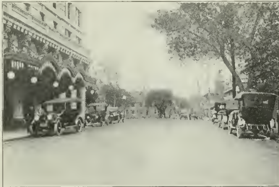
Wilmington, Delaware. Eleventh Street, looking West from Market. Showing Hotel DuPont at left. Bitulithic Pavement laid over Old Brick in 1910. Photograph taken September 15, 1915.
