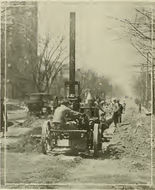
SHOWING MACHINE TAMPING SURFACE FILL. NOTE COMPACTING EFFECT OF TAMPER HEAD.
