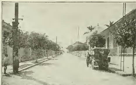
View 2—Looking up General Lee Street from intersection of Dolores Street, Marianao, Cuba. View taken April 1915. Tarvia macadam laid in August 1914.
