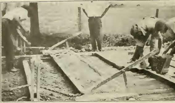
TEMPLATE by which dry mortar mix is spread on green concrete base just in advance of brick laying.
