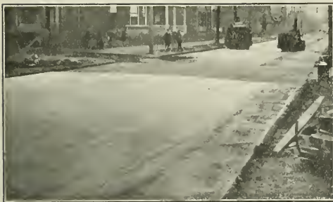
RESURFACING SIXTH STREET, Columbus, O., with Trinidad sheet asphalt, using 1½-inch binder and 1½-inch top. Laid in 1912 over old brick street. Shows the steps in the process.
