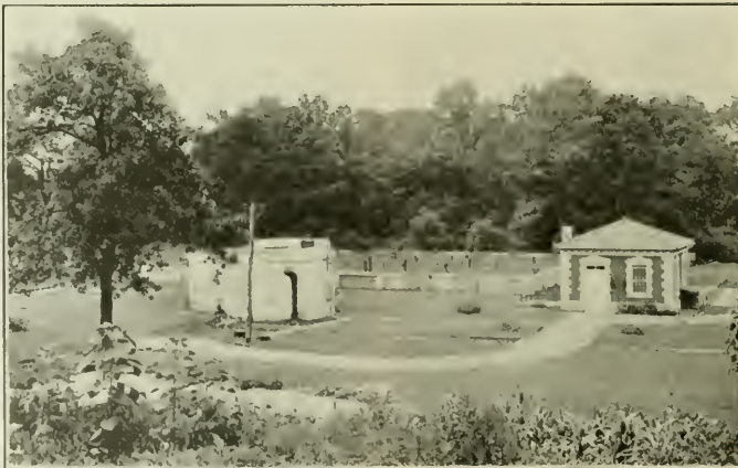
CIVIC BEAUTY IN A SEWAGE DISPOSAL PLANT. DESIGNED BY ALEXANDER POTTER, C. E.
