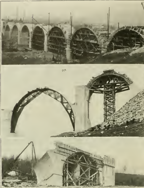
METHODS OF CENTERING and of supporting Centers and Forms.
