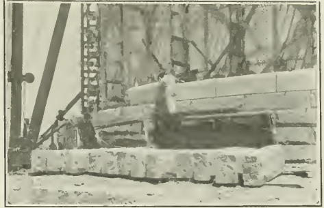
LAYING COURSED ASHLAR in the masonry wall surrounding the steel tank. Note space between masonry and steel.
