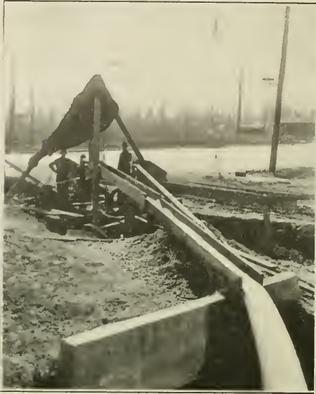
ELECTRICALLY DRIVEN CENTRIFUGAL PUMP taking water from man-hole in 16-foot trench. The portable sub-station is at the left in the background behind the line pole.
