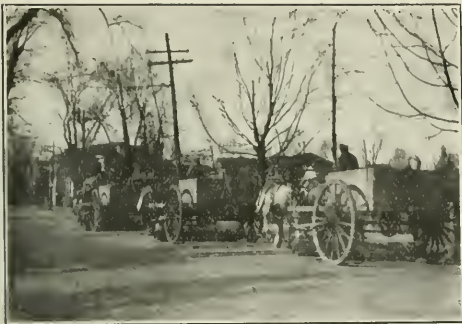
THREE SQUEEGEE MACHINES running in a gang, preceded at some distance by a street sprinkler to soften up the dirt on the pavement.
