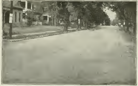
West Walnut St., Springfield, Mo., showing "Tarvia-X" wearing course over old brick.
