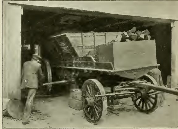
VIEW SHOWS 120 CUBIC FOOT TRAILER BENEATH MIXER, ILLUSTRATING METHOD OF JACKING UP FROM EXTRA SET OF WHEELS SO THAT TRACTOR CAN BE PLACED UNDERNEATH.
