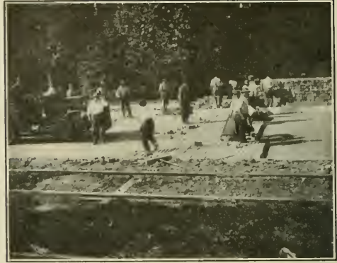
LAYING AND ROLLING brick surface on old macadam base on Cedar Glen Hill, near Cleveland, O.
