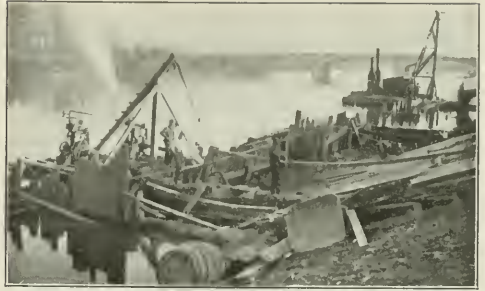
LAYING CONCRETE RIP-RAP BELOW THE WATER LINE AT TOE OF LEVEE SLOPE, UNDER PROTECTION OF COFFER DAM. MICHIGAN STREET BRIDGE IN BACKGROUND. THIS BRIDGE WILL BE LENGTHENED TOWARD THE LEFT WHEN THE EAST BANK OF THE RIVER IS IMPROVED.
