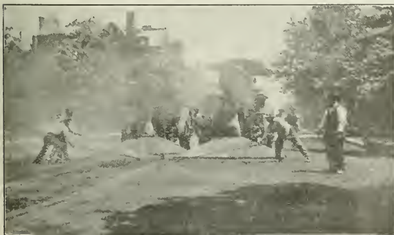
USING TWO LUTZ SURFACE HEATERS ON WEST END AVENUE TO DETERMINE THEIR ADVANTAGE OVER SMALL HAND BURNERS.
