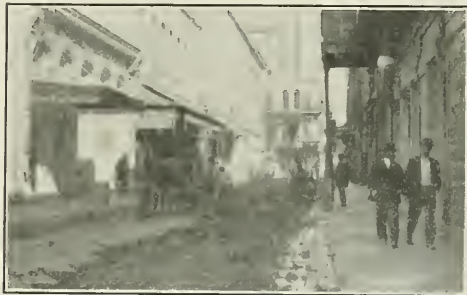
PAVEMENT NEARLY ONE HUNDRED YEARS old being removed to replace with wood block.
