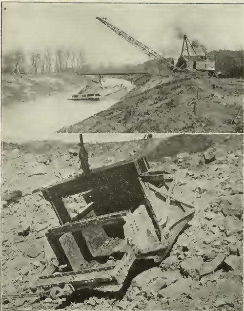
BROWNHOIST SCHNABLE BUCKET as used on Chicago Drainage Canal construction.
