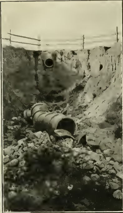
H EAVY FLOOD and consequent wash-out produced this condition of the small vitrified pipe culvert which was sufficient for all ordinary conditions.
