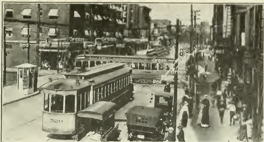
S EMAPHORE STREET CAR SIGNALS at crossing in Cleveland, O. Starter's box at left. Note carefully red signals on near sides of crossings for stop signs, green signals on far sides for safety signs. Both cannot show at once. Lights by night and discs by day.
