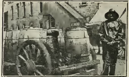
TAR in these barrels removed from sewer by turbine sewer cleaner.
