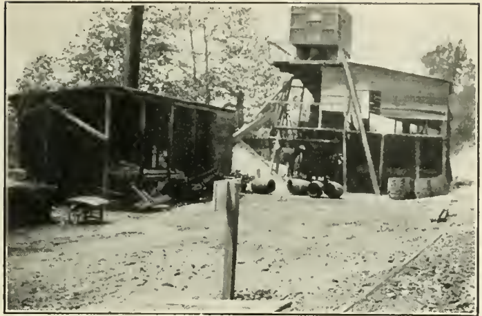
General view of bitu- lithic paving plant, with dryers in the foreground.
