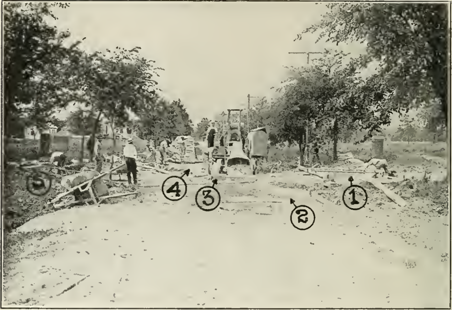
M -C RAIL TRACK paving mixer at work at Wilmette, Ill., showing order of construction of street intersection at treatment of manhole.
