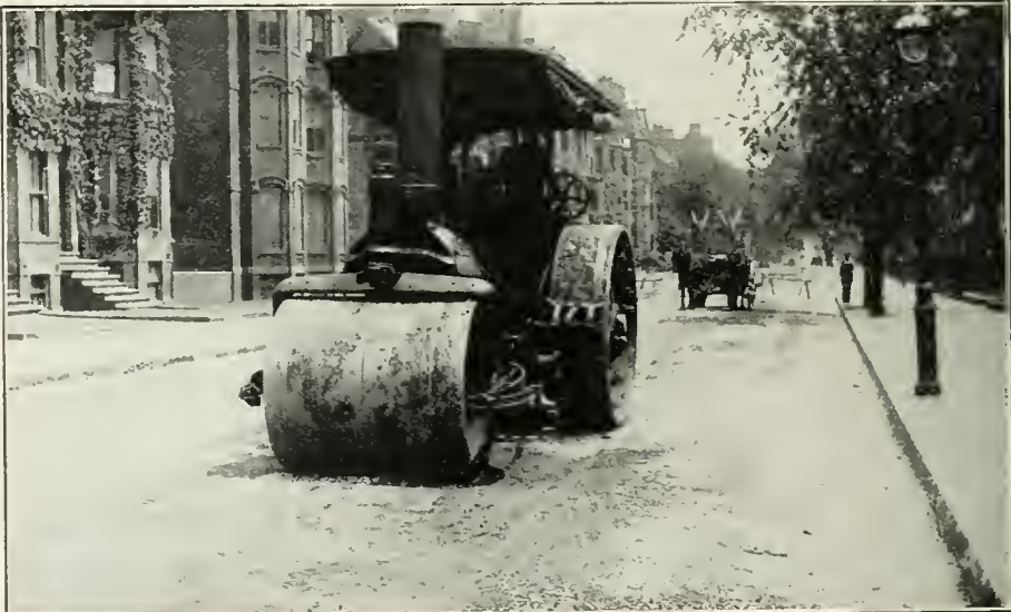
MARLBORO STREET, Boston, Mass. Rolling the regulated old macadam roadway preparatory to laying bitulithic wearing surface.
