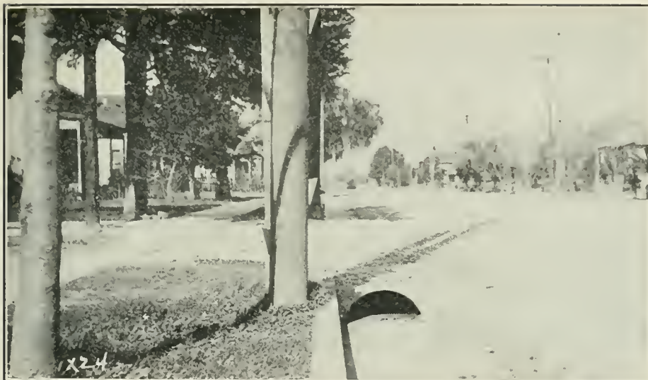
C ORRUGATED IRON CULVERT at street intersection in San Bernardino, Cal. One of many part-circle culverts, specially adapted for such work, where depth is not available.
