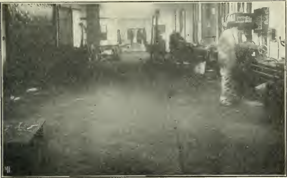
SHOP FLOOR paved with creosoted wood blocks.
