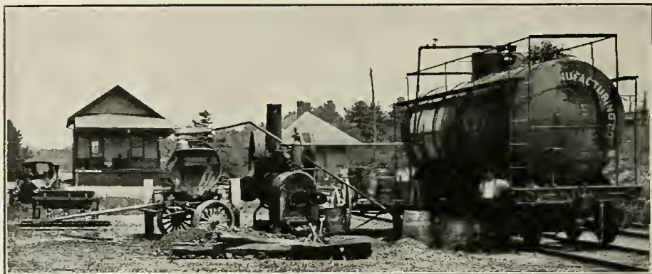
TANK CAR HEATED BY STEAM FROM BOILER AND UNLOADED BY STEAM PUMP TAKING THE TAR THRU DOME OF TANK CAR FOR MASSACHUSETTS HIGHWAY COMMISSION AT PONDVILLE.
