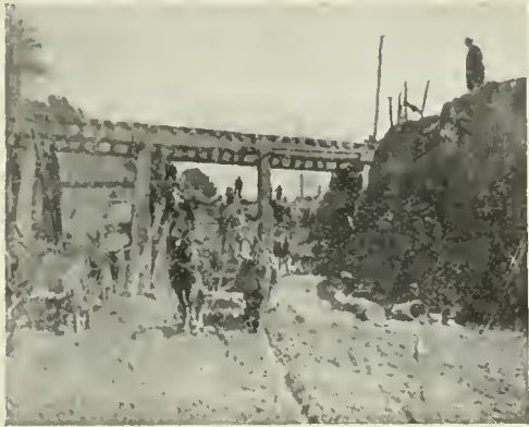
E ELIMINATING GRADE CROSSING by lowering grade of highway, work done by Fulton county, Georgia, convict labor.
