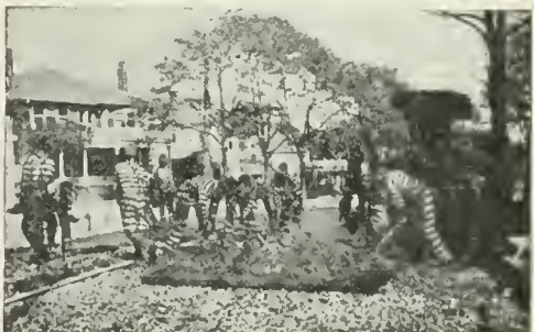
C ONVICTS in Fulton county, Georgia, spreading Warrenite road surface.
