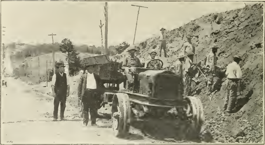
F IVE-TON TRUCK on road work in Cabarrus County, N. C. Convict labor is used. Note the steep hills to the fill at the bottom to reduce the grades.
