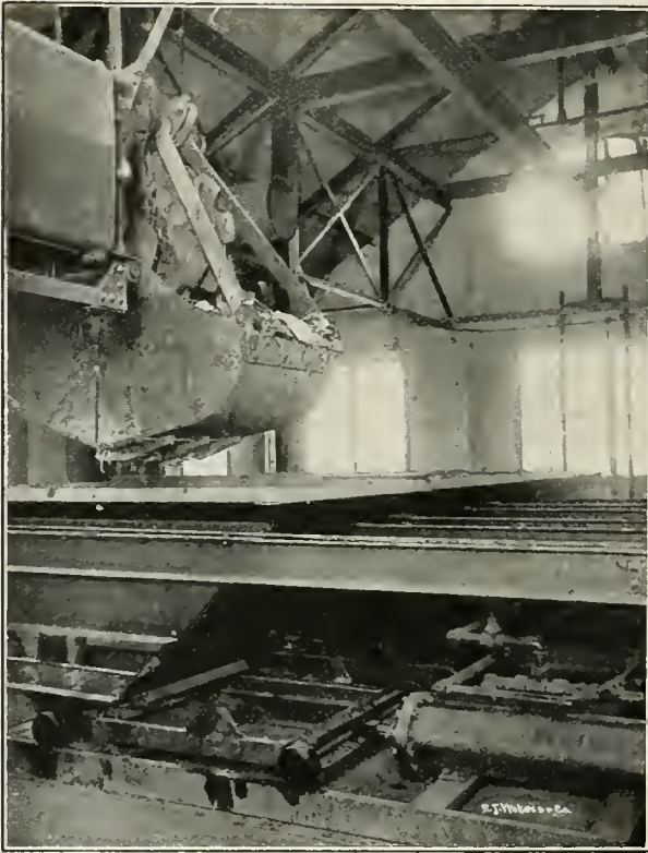
C HARGING FURNACE with garbage by means of grab-bucket.
