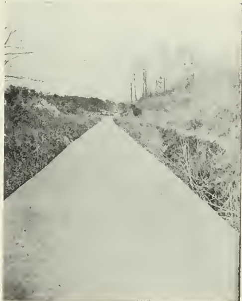
C ONCRETE SEWER of fourteen feet diameter, built by Fulton county, Georgia, convicts.
