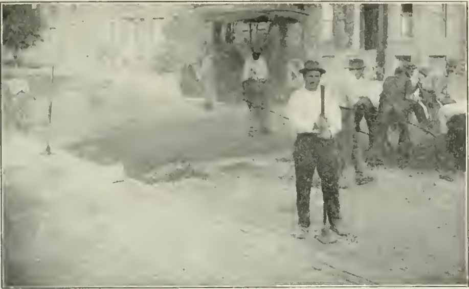
M ARLBORO STREET, Boston, Mass. Laying bitulithic surface over old macadam, after regulating the grade.
