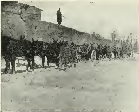
R OAD GRADING with outfit of four-wheeled scrapers, using Fulton county, Georgia, convict labor.
