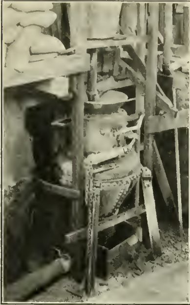
N EARER VIEW OF MIXER and conveyor. Two men handle all the work at this point.
