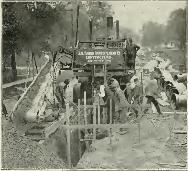
LAYING PIPE SEWER in Des Moines, Iowa, with trench machine and conveyor for back-filling.
