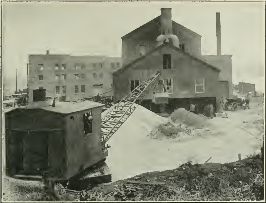
P ITTSBURG'S ASPHALT PLANT for North Side, completed, looking south. Stone and sand storage in foreground with portable crane unloader. This is the same end shown in the first photograph.
