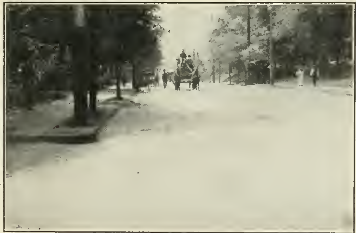
Peachtree street, looking south from Eighth street. Finished street, after placing flush coating of asphaltic cement and fine stone, and rolling. View taken two hours after work was finished.
