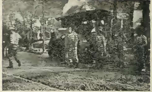
ROLLING Warrenite road surface in Fulton county, Georgia, using convict labor.
