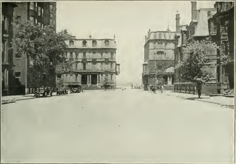
D ARTMOUTH STREET, Boston, Mass., June 15, 1914, from Marlboro street, looking toward Beacon street. Bitulithic surface, laid on old macadam foundation in 1903.
