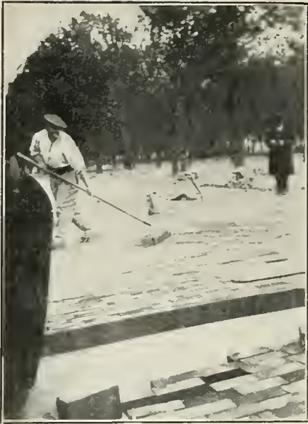
PARIS WOOD BLOCK PAVING. Applying cement and sand grout to surface of completed pavement in Cours la Reine.
