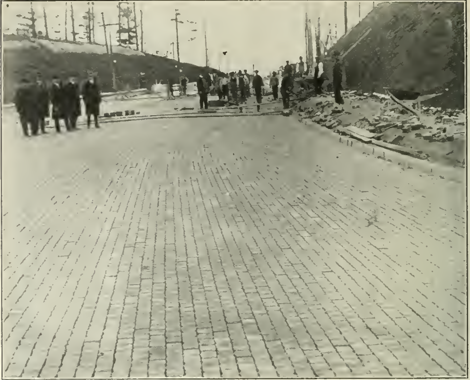
C HRISTIE STREET, Toronto, under construction. Laying wire-cut-lug hillside blocks on 6.25 per cent. grade, city work by day labor.
