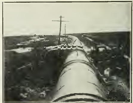
A TLANTIC CITY WATER MAIN. Section partly buried, with one of the eleven valves which divide the 23,000 feet of pipe into sections.
