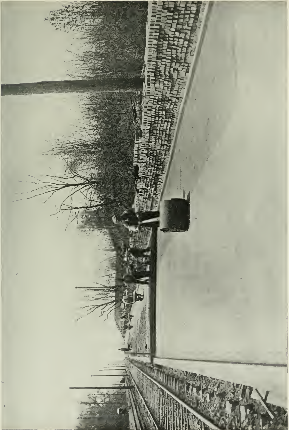
Fig. 2. Thoro compression of sand cushion essential.
