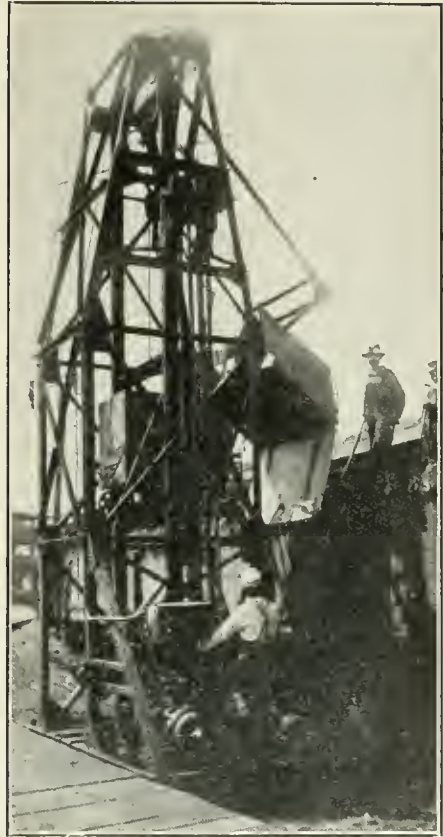
U NLOADING ELEVATOR, running on track parallel to railroad cars, lifts refuse cars and dumps them into the flat cars.
