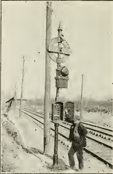
C CROSSING SIGNAL at Hume, Va., operated by cars on either track. The word "Danger" is lighted and the bell is rung by car approaching on its proper track.
