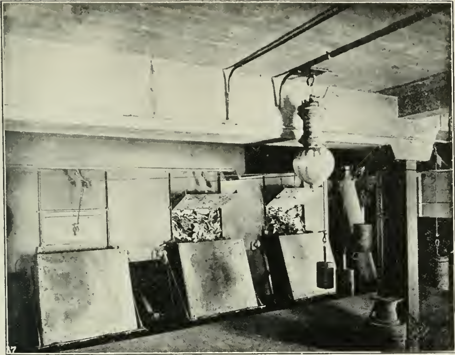
FRONT of garbage and refuse hopper, showing container system.
