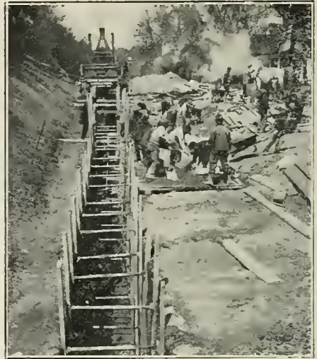
CONCRETE SEWER, Des Moines, Iowa, 3 feet wide by 3.5 feet high; trench 20 feet deep, 4 feet wide.
