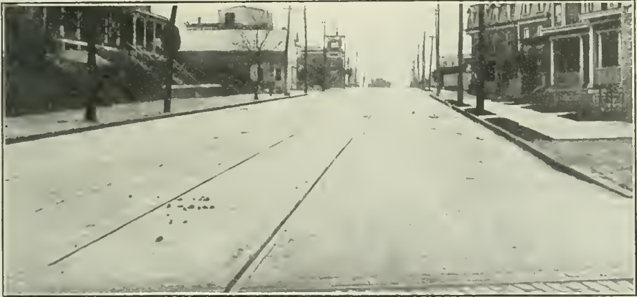
MARKET STREET, WILMINGTON, DEL. BITULITHIC PAVEMENT WITH STONE BETWEEN STREET RAILWAY TRACKS.
