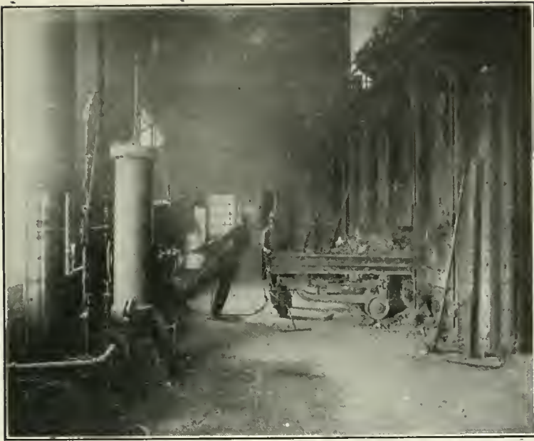
S AVANNAH DESTRUCTOR. Drawing clinker from grate into clinker car. Note greater ease of drawing clinker by means of the apparatus provided than removing by hand, as in earlier furnaces.
