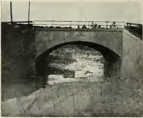
Concrete bridge built by Fulton county, Georgia, convicts. Forty feet span, sixty feet width.
