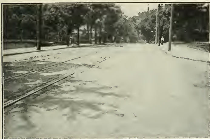
Park street, looking west from Hammond street, in use ten years. Bad condition along car track is due to settling of the track.
