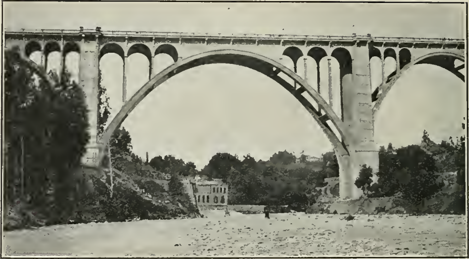
COLORADO STREET BRIDGE. Pasadena, Cal., showing the main 210-foot span and the height of the bridge above the bottom of the Arroyo.
