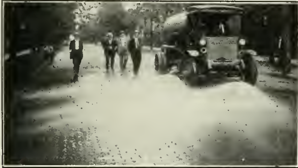
THE ETNYRE STREET FLUSHER with constant water pressure.
