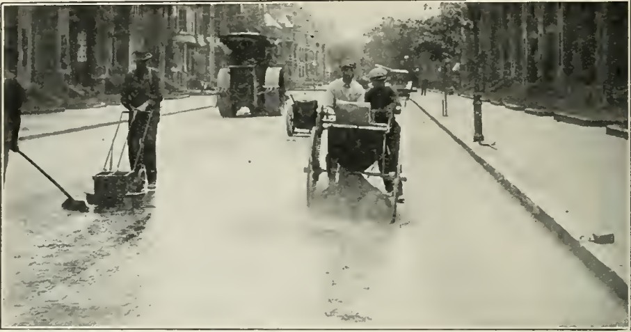
MARLBORO STREET, Boston, Mass. Spreading flush coat of bitumen and stone chips over bitulithic surface.
