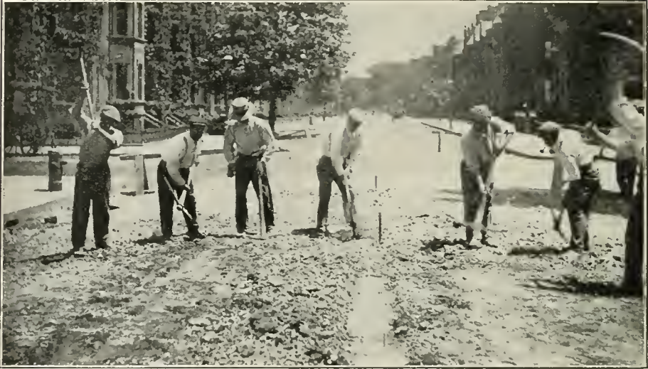
MARLBORO STREET, Boston, Mass. Picking surface of old macadam to reduce crown preparatory to laying new bitulithic surface.
