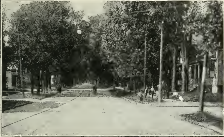
West Dominick Street, Rome, N. Y., looking west from the Wood Creek Bridge, 3,600 feet. This street, before being improved, was the worst roadway in Oacida County.
