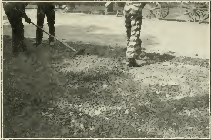
Peachtree street, looking toward Eighth street. Bitulithic surface after rolling to grade and before placing flush coating of asphaltic cement and fine stone.
