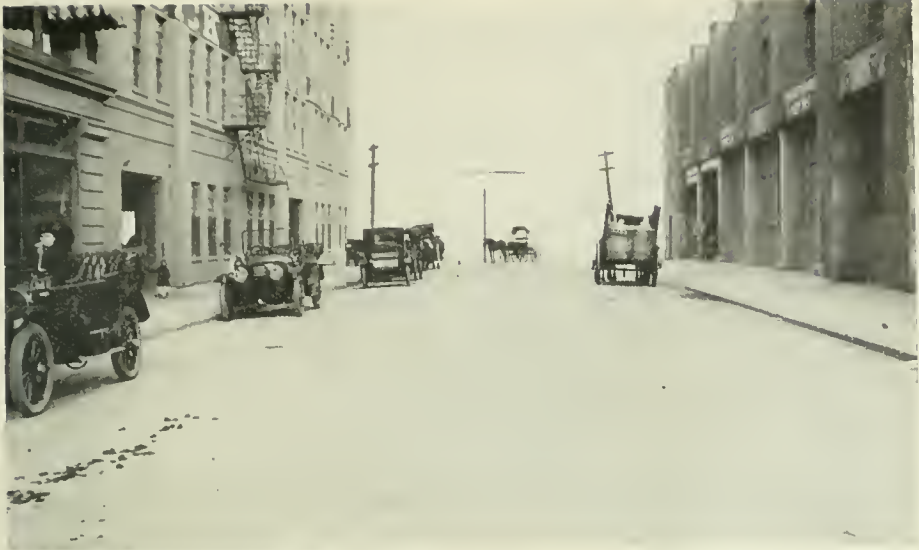
T WO-COURSE PAVEMENT for heavy traffic on Twenty-first street, near the lake, Chicago.
