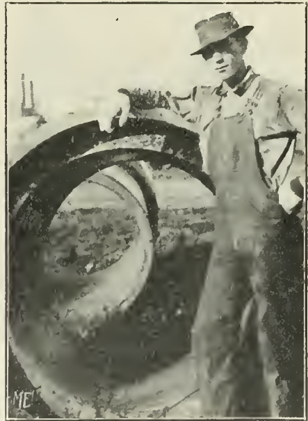
FORTY-TWO INCH VITRIFIED SEWER PIPE, ready for sewer near Chicago.
