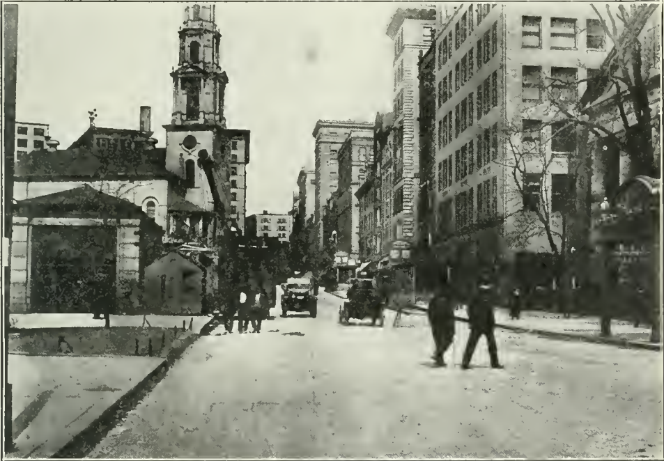
Tremont Street, near Temple, Boston, Mass. Laid in 1900—Southern Long Leaf Yellow Pine. This street is heavily traveled and in excellent condition today, having cost practically nothing for repairs.
