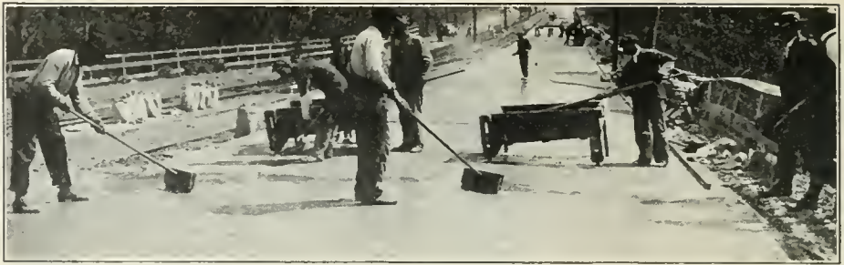
G ROUTING the Chevy Chase Sample brick road. Laying and rolling brick in background.
