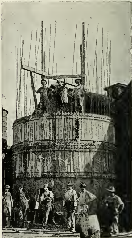
METHOD of constructing and reinforcing coniform chimney.
