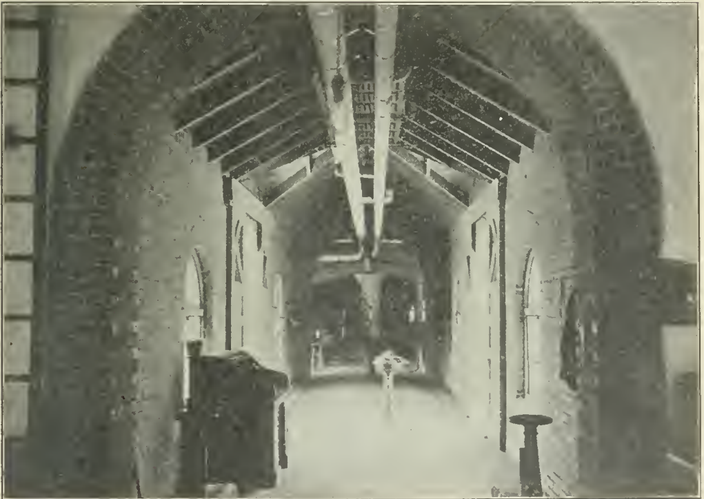
ARCADE connecting water softening and filtration plants, McKeesport, Pa.
