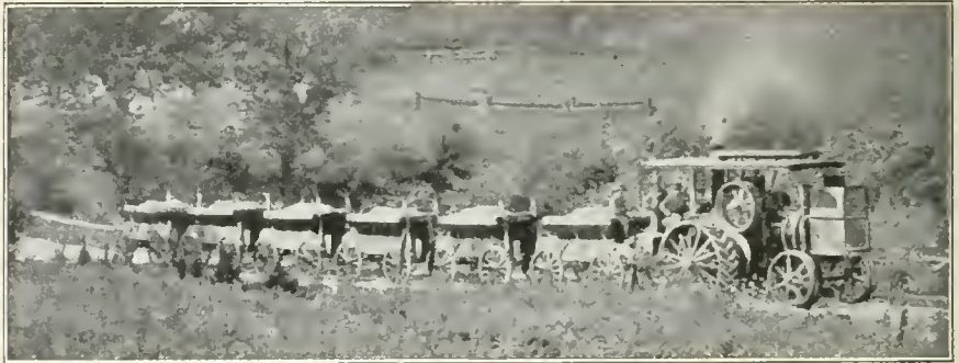
HUBER Traction Engine Hauling Broken Stone for Road Construction.
