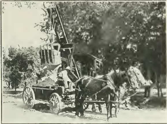
PAVING CONSTRUCTION in St. Paul, Minn. Excavating with steam shovel.
