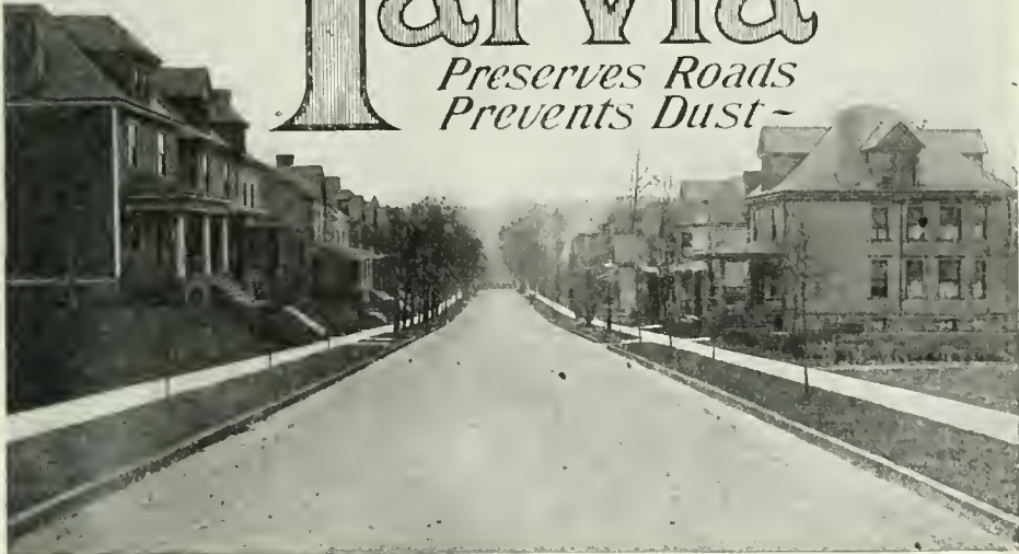
Monitor Avenue, Ben Avon, Pa. Constructed with "Tarvia X."
