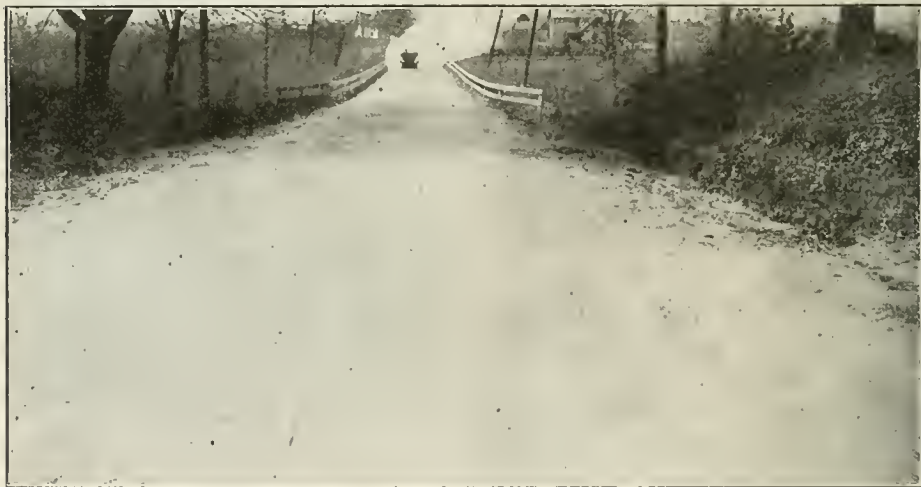
MACADAM on Center Road near Conneaut, O. Note heavy dust and cloud raised by automobile.
