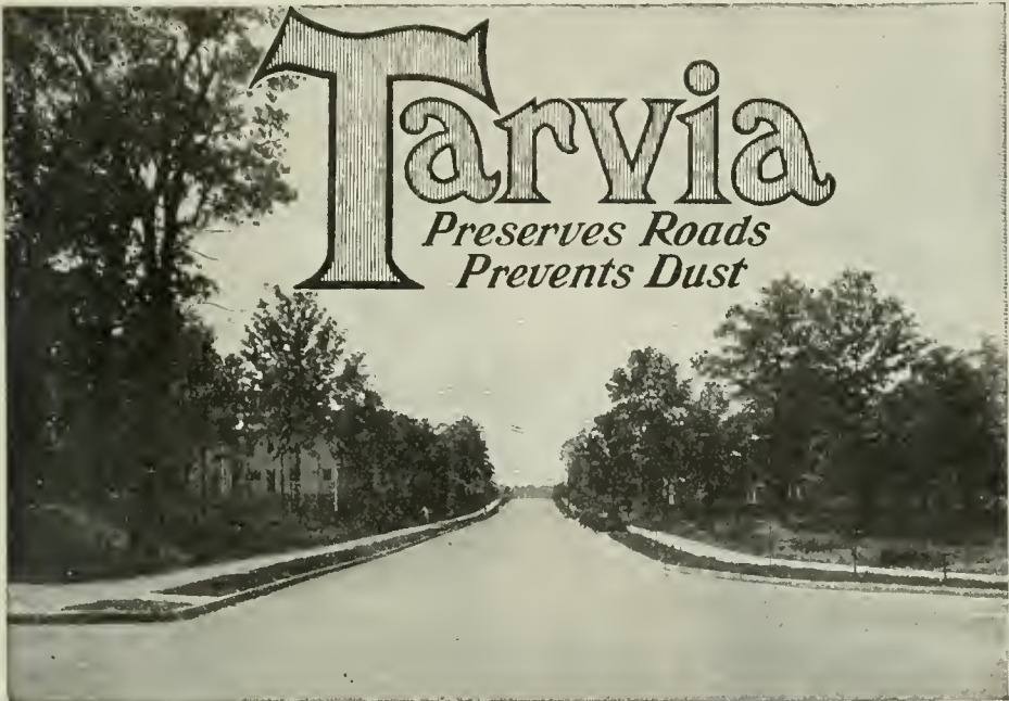
29th Street, Norwood, Birmingham, Ala. Road Built with "TARVIA X."
