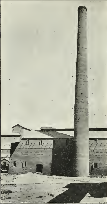
REINFORCED concrete chimney constructed for Lehigh Portland Cement Co. at Mason City, Ia. Total height 208 feet 9 inches.
