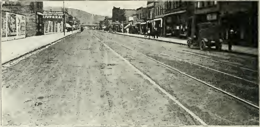
CREOSOTED YELLOW pine street, Duluth, Minn. On 15,940 square yards laid in 1904 to date there has been no up-keep or maintenance attached to this kind of pavement.
