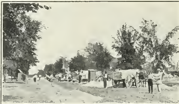
PAVING CONSTRUCTION in St. Paul, Minn. Hauling stone.
