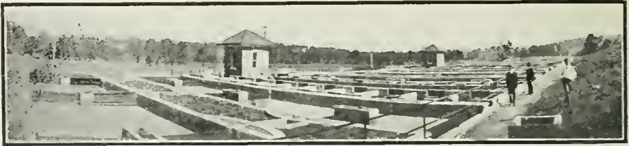
GENERAL view of Peachtree Creek Sewage Disposal Plant, Atlanta, Ga. Imhoff tanks in foreground. Sprinkling filters in rear at left of center. Grit chamber and sludge beds at extreme right in background. Towers indicate location of groups of roughing filters.
