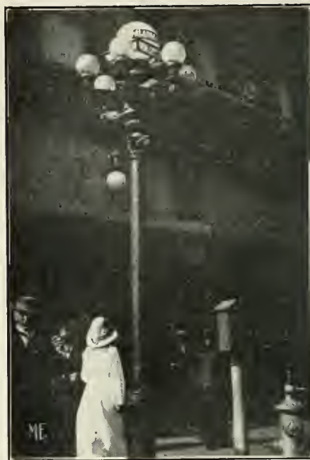
ORNAMENTAL Lighting Posts give prominence to fire box locations.
