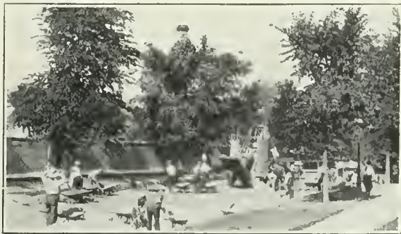
PAVING CONSTRUCTION in St. Paul, Minn. The concrete mixer gang laying pavement foundation.
