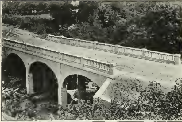
PARK BRIDGE, Marble Park, Iowa, built by Miller Hey Construction Co., Waterloo, Ia., in 1912.
