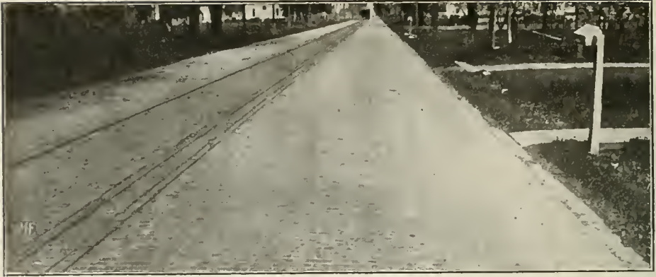
BRICK ROAD with cement filler near Conneaut, O. Note perfect surface.
