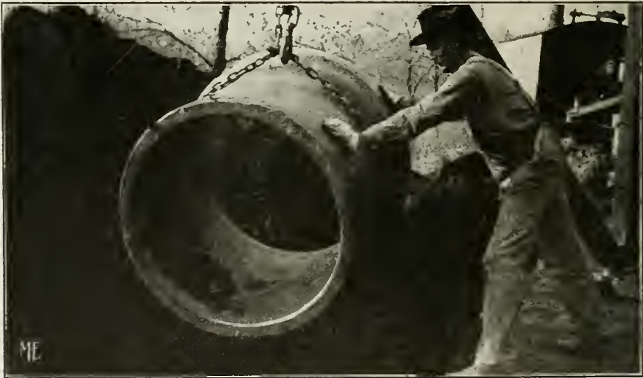
VITRIFIED PIPE, THIRTY-SIX INCHES DIAMETER, going into sewer trench near Chicago.
