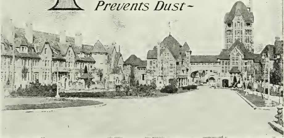
Sage Foundation Homes Co., Forest Hills, L. I. Constructed with "Tarvia X" 1910, Treated with "Tarvia B" 1913.
