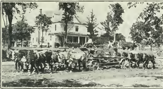
PAVING CONSTRUCTION in St. Paul, Minn. Grading with twelve-horse team.
