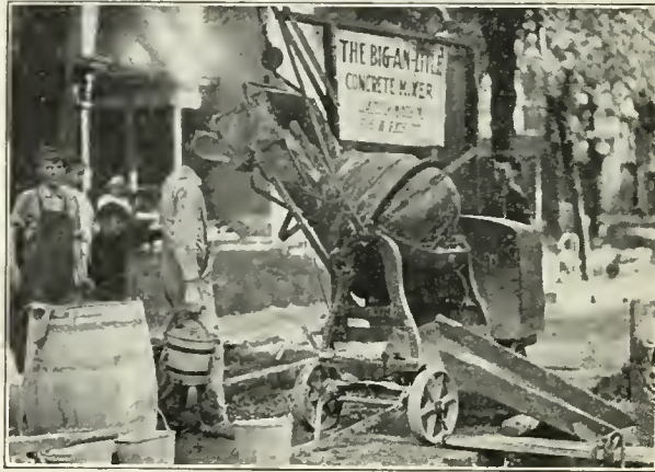
BIG-AN-LITTLE Concrete Mixer discharging into sewer forms from edge of trench.
