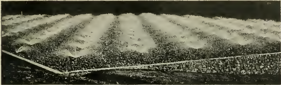
140 TAYLOR HEXAGONAL NOZZLES at Chambersburg, Pa., operated by one 20-in. Miller Sewage Siphon.
