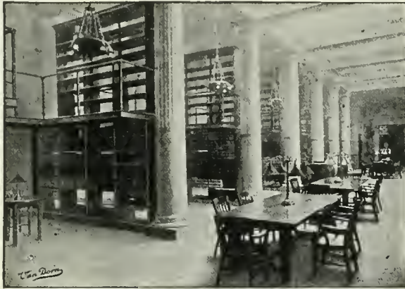
Enclosed Type Library Shelves and Mezzanine Floor, Law Library, Shelby County, Memphis, Tenn. Jas. Gauble Rogers (of Hale & Rogers, Architects).
