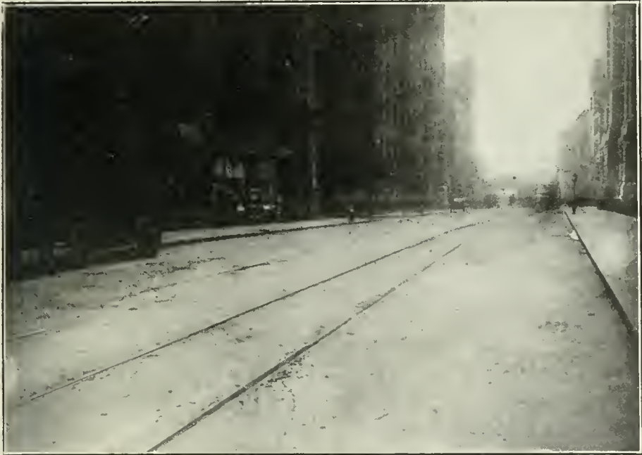
Yellow Pine Creosoted Blocks on Whitehall Street, New York City—very heavy traffic.
