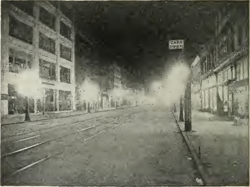
W ATER STREET, Elmira, N. Y. Note well distributed illumination. No deep shadows. Posts 60 feet apart, three 80 c.p. lights on each.
