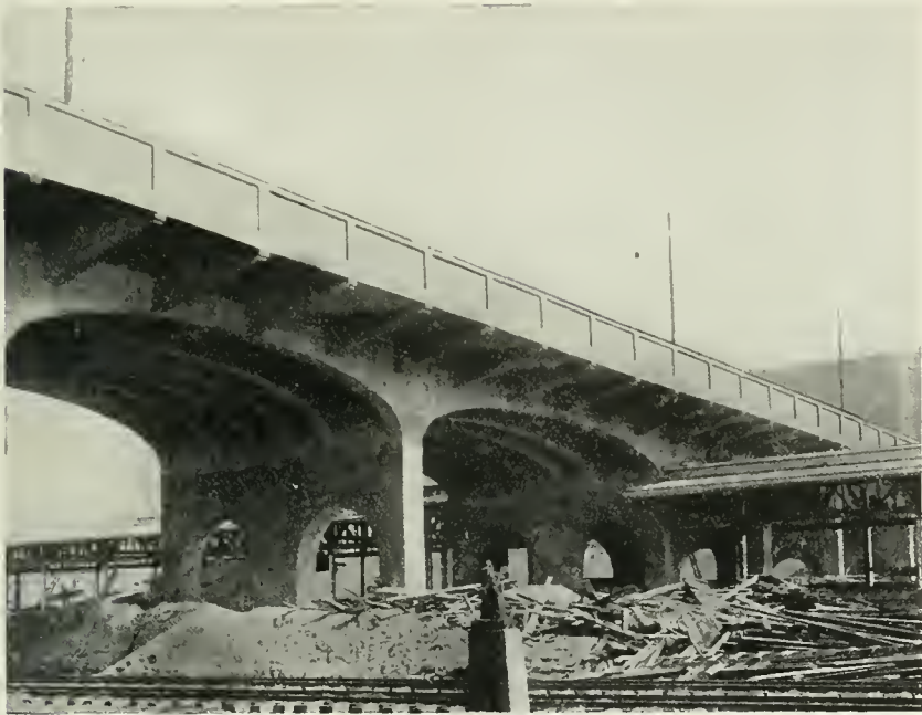
NELSON Street Viaduct, Atlanta, Ga., a Concrete Structure of Attractive Design.
