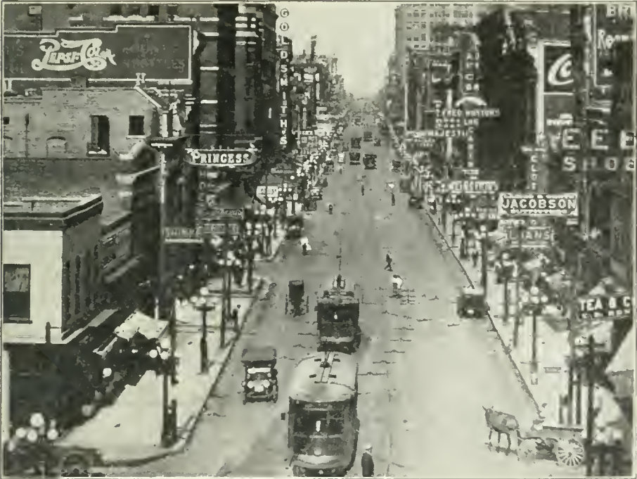
MAIN STREET, Memphis, Tenn., equipped with new ornamental lighting system.
