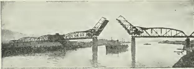
LARGEST Bascule Bridge in the World—4,800 feet long. Over Willamette River, Portland, Ore.
