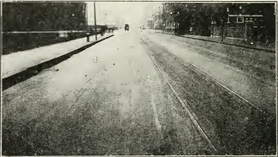
CREOSOTED wood block pavement in Boston, Beacon Street, near Bay State Road.
