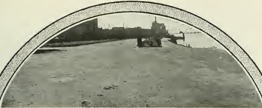
Asphalt Macadam Pavement, La Crosse, Wis. Constructed with Sarco Asphalt Binder No. 298.
