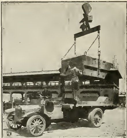
MOTOR TRUCK BODY IS REMOVABLE SKIP BUCKET. A five-ton Saurer truck, with body handled by a crane with a derrick boom.
