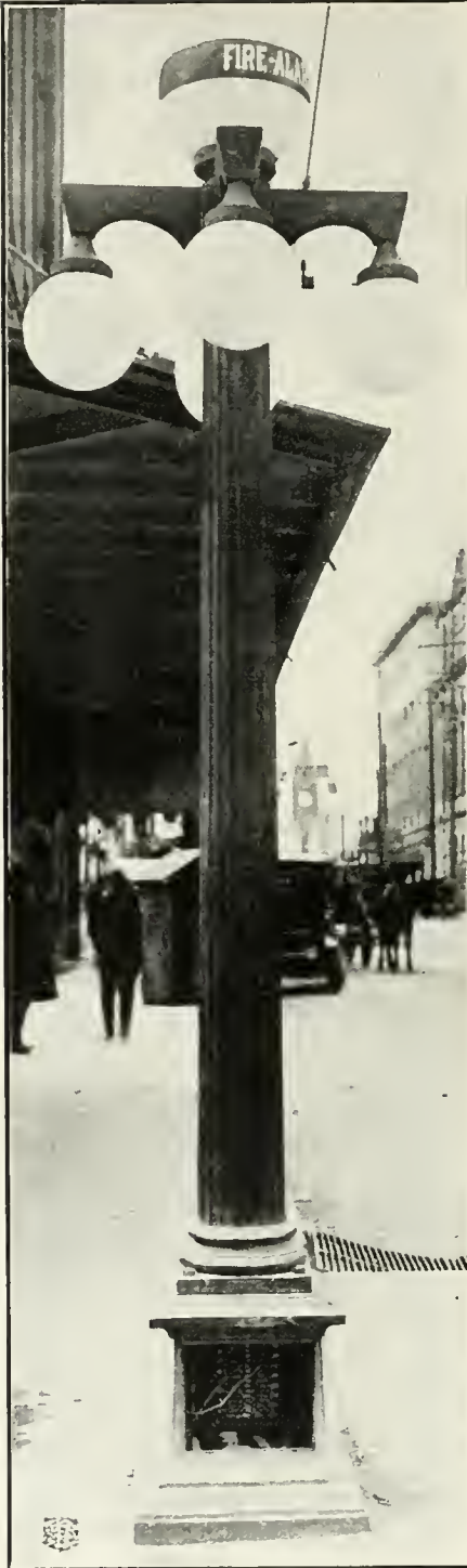
O RNAMENTAL standard to which are attached both Police and Fire Alarm Boxes.
