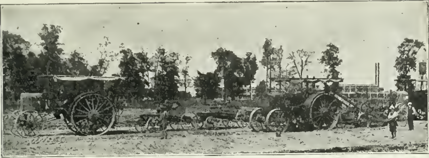
Huber Gas Tractors Grading and Hauling for Streets of Speedway City, Ind. (Much of the time running 24 hours per day.) C. C. King Brother & Son, Contractors.
