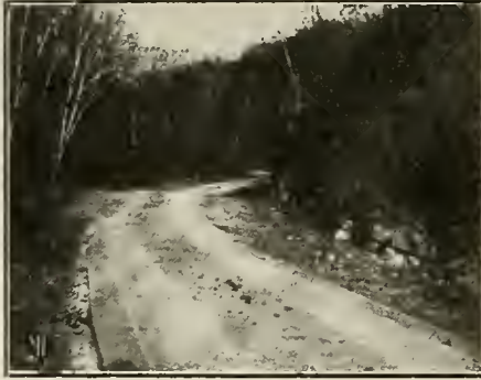
CONCRETE ROAD in Winona County, Minnesota. Gravel shoulders had not been put in when this photograph was taken.
