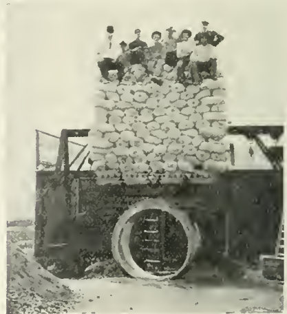
TEST of 60-inch Concrete Pipe, showing final load.
