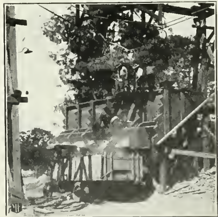
M ETHOD of loading Speedicell trucks by gravity—a method which eliminated costly delays and kept trucks moving almost constantly.
