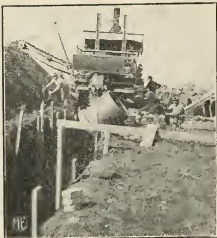
LOWERING THIRTY-INCH VITRIFIED PIPE into trench. Chicago sewer construction, 1912.
