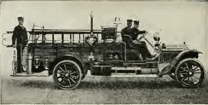
COMBINATION hose and chemical truck capable of a speed of fifty-five miles per hour. Manufactured by the White Company, Cleveland, Ohio.
