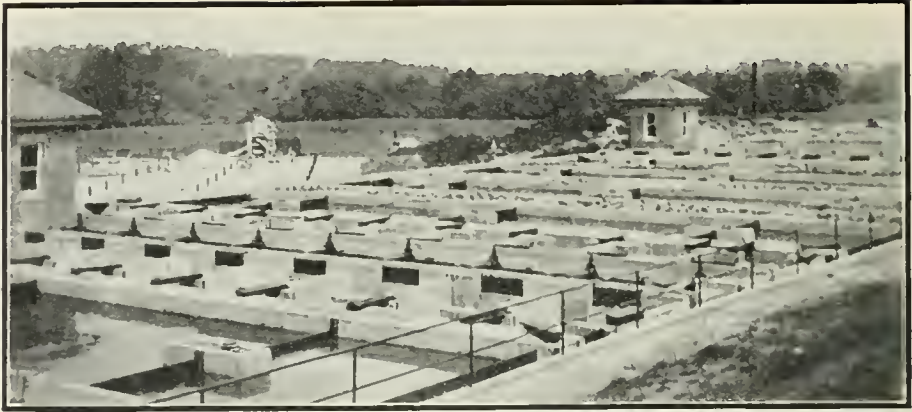
R OUGHING filters to remove solids from Imhoff tank effluent, Atlanta, Ga., Sewage Disposal Plant. Imhoff tank in left foreground. Roughing filters with gate and pumphouse next in rear. Then more Imhoff tanks, more roughing filters, and again more Imhoff tanks. Sprinkling filter bed in background.
