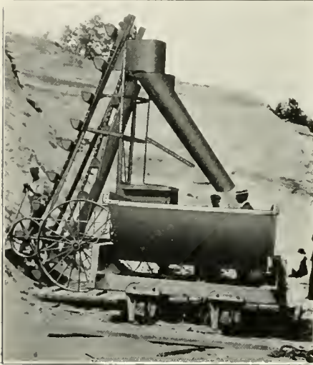
2. LINK-BELT machine equipped for loading sand.
