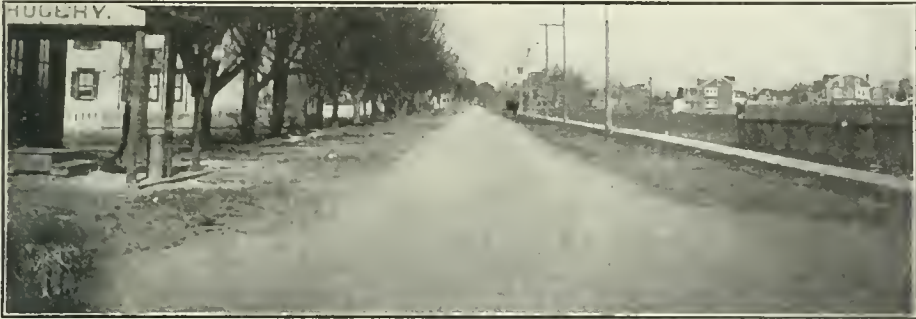
BITUMINOUS CONCRETE HIGHWAY, Chalmers and Liberty Streets, Mercer County, Trenton, N. J. This type of pavement is being used quite extensively through New Jersey and is proving successful.
