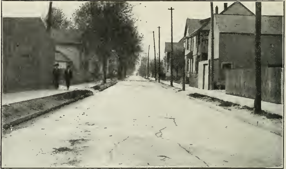
ELMWOOD AVENUE CONCRETE PAVEMENT, Detroit, Mich., not reinforced. Note cracks, longitudinal, transverse and irregular.
