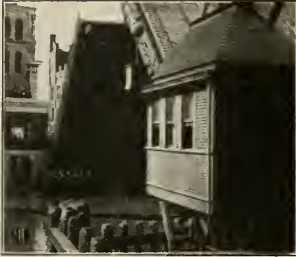
GRAND AVENUE LIFT BRIDGE, Milwaukee, Wis.
