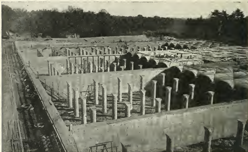
R ESERVOIR for filtered water as it appeared under construction. Forms for roof arches in place at the right.
