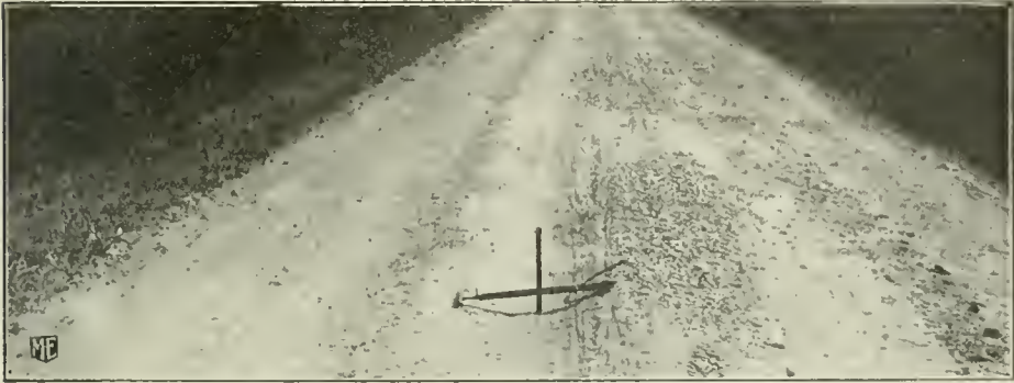
MACADAM ROAD near Conneaut, O. Note depth of rut.
