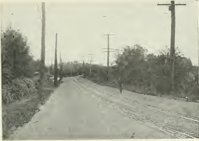
M ONTFORD AVENUE, Asheville, N. C., looking west. Fill, 19 feet deep in center of roadway and 45 feet on right side. Fill made and bitulithic pavement laid in 1906. No settlement to September, 1913, when this view was taken.
