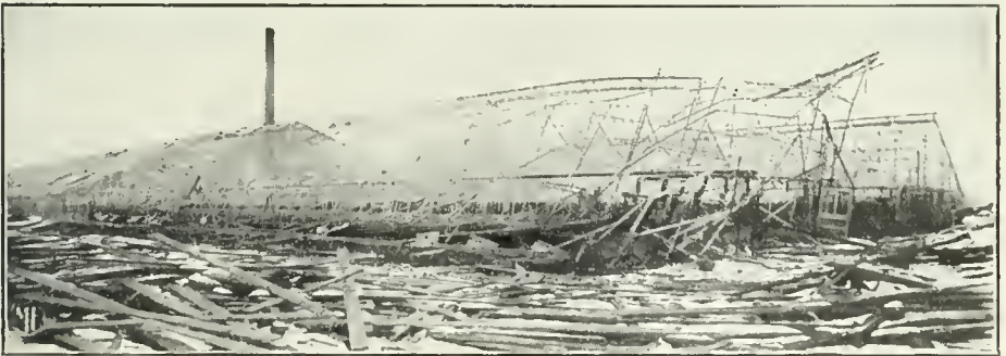
A CYCLONE caused this ruin at J. T. Wilcox & Sons' Plant, Council Bluffs, Iowa. Weber concrete chimney in rear remained uninjured.
