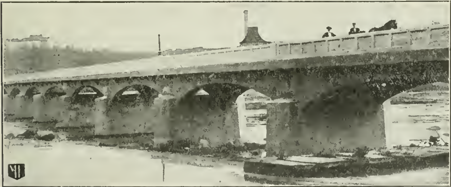
REINFORCED CONCRETE BRIDGE on Union Street, Danville, Va.
