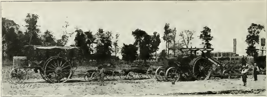
HUBER TRACTOR hauling stone for road construction.
