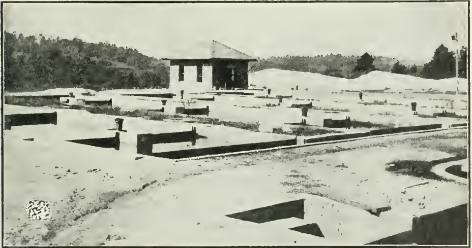
1. ATLANTA Sewage Disposal Plant. Parts of sand trap and grit chamber show in lower right-hand corner. Imhoff tanks in center, with screen and head house at rear corner, distributing sewage to filters beyond on the left.
