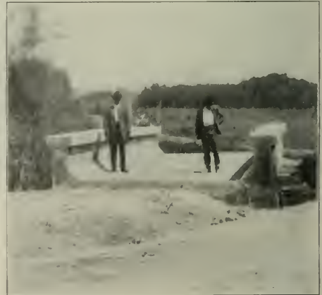
CONCRETE GIRDER BRIDGE. Near Pulaski, Va.
