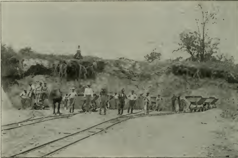
STREET EXCAVATION IN NEWCASTLE, PA.
