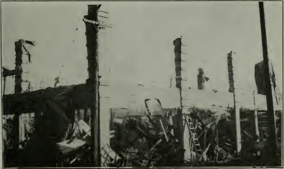
I. PREST-O-LITE BUILDING FAILURE.
