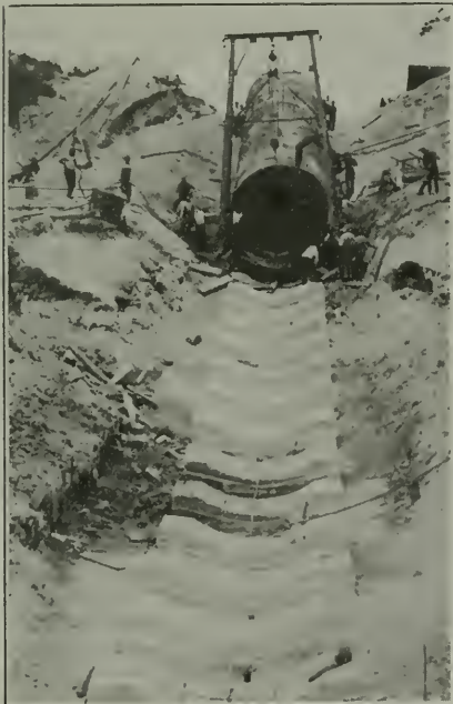
CASTKILL AQUEDUCT. STEEL PRESSURE SIPHON.
