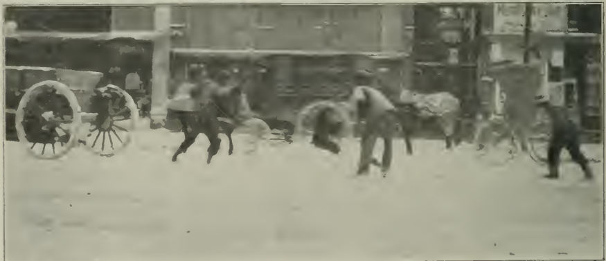
III. SNOW REMOVAL IN INDIANAPOLIS. Shoveling into Sewer.
