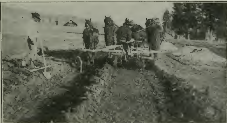
2. REVERSIBLE ROAD MACHINE ON STREET WORK IN LOS ANGELES.
