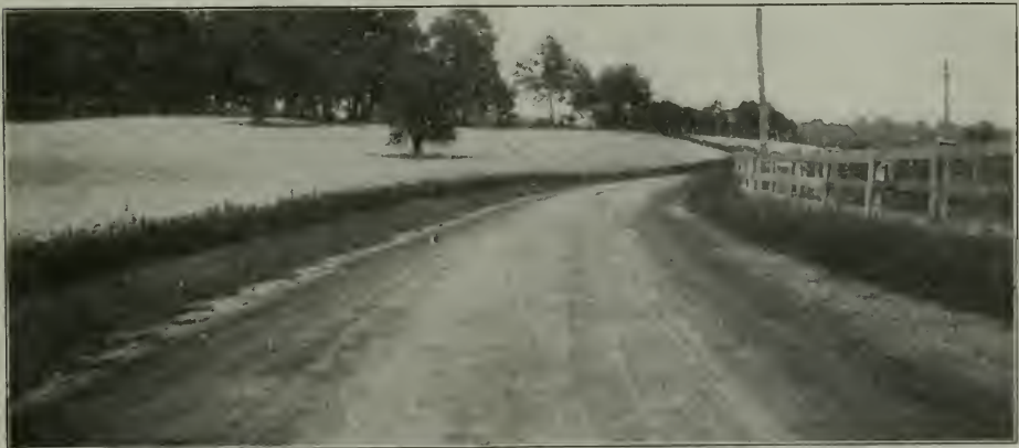
6. PARK HEIGHTS EXPERIMENTAL ROAD, BALTIMORE, MD. Section 29. Robeson Process Co., Glutrin.
