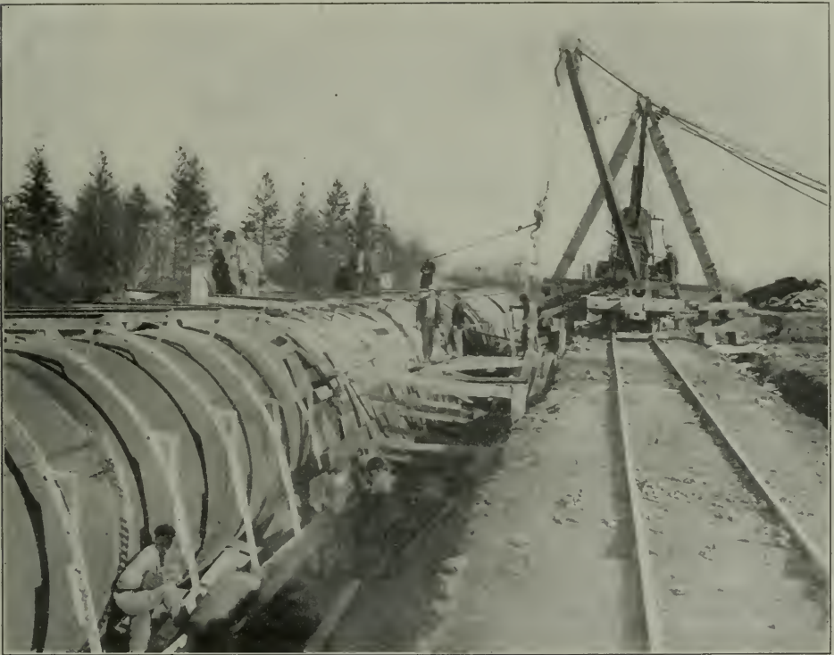
BRYN MAWR SIPHON. Placing Concrete Envelope Around Steel Pipe.
