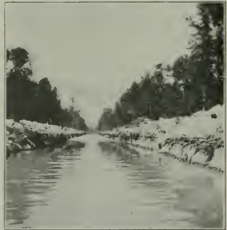
4. DRAINAGE CANAL BEFORE CONSTRUCTION OF ROAD ON EMBANKMENT.
