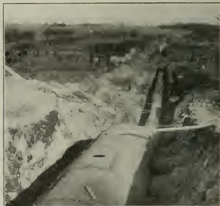
KENSICO SIPHON. Showing Temporary Manhole.
