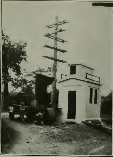
CONDUIT WORK IN WESTFIELD, MASS. Terminal House with Pole for Distributing Lines.
