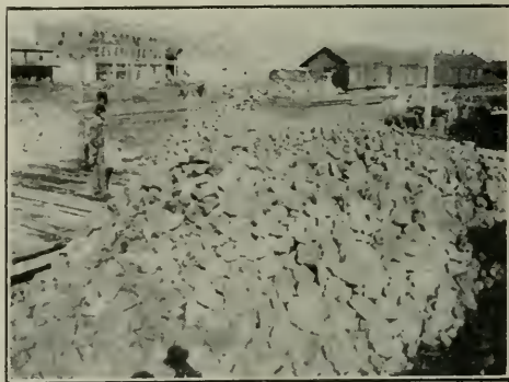
ARDMORE ASPHALT READY FOR SHIPMENT.
