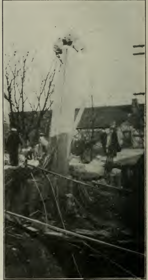
II. PREST-O-LITE BUILDING FAILURE. Two Columns at the S. E. Corner.
