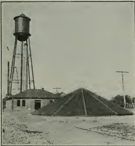
WATER WORKS PLANT AT CENTRALIA, MO.
