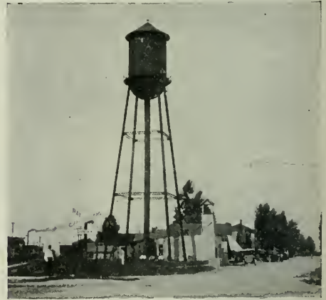
SHIRLEY IND., WATERWORKS. Tank, Pumping Station and City Hall.
