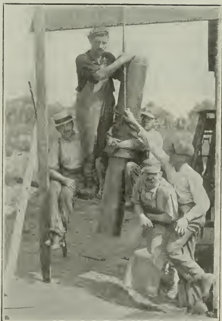
3. G-K COMPOUND JOINT UNDER TENSION.
