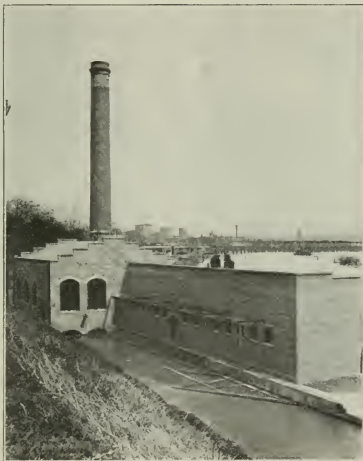
THE RICHMOND, VA., POWER PLANT.
