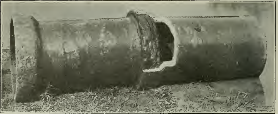
2. CUT SEWER PIPE JOINT SHOWING FILLING WITH G-K COMPOUND.
