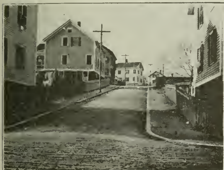
HARVEY STREET, PAWTUCKET, R. I. Bitulithic Pavement on 12 per cent. Grade. Macadam Street in Foreground.
