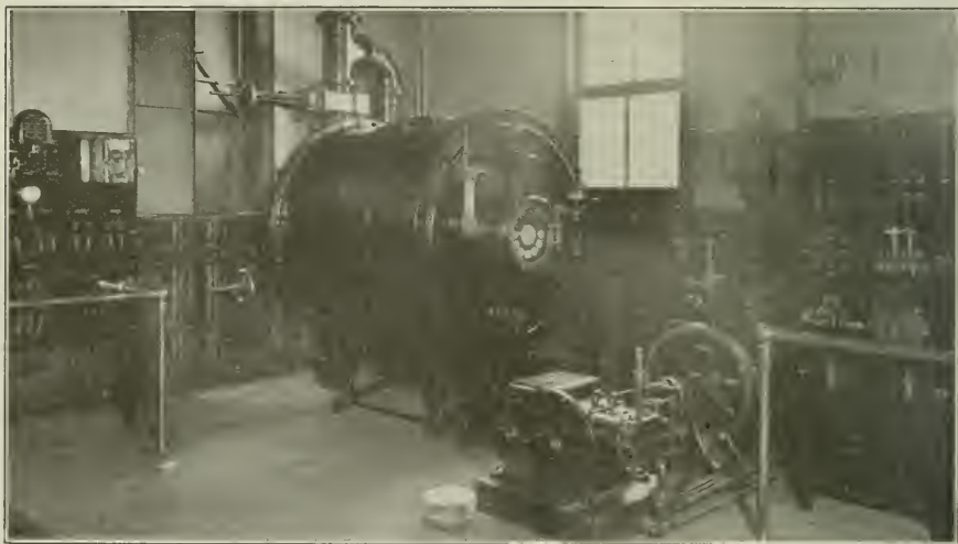
GAS METER AND ENGINE FOR HIGH PRESSURE FIRE SERVICE.
