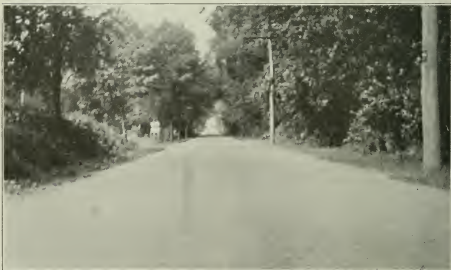
BARRINGTON, R. I., EXPERIMENTAL ROAD. IV. Tarite Asphalt, (10 Percent.)
