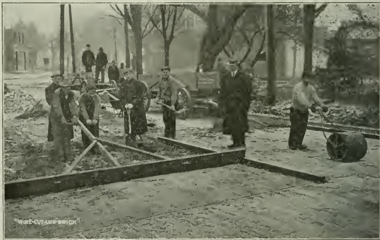
THE BUFFALO-WILLIAMSVILLE ROAD. Leveling the Sand Cushion.
