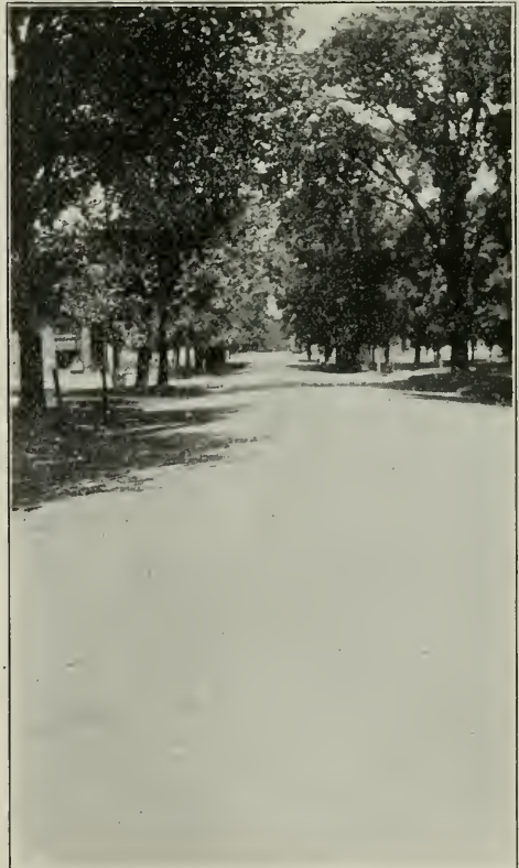
SECTION IV. TARVIA "X" BINDER. Ohio State Experimental Road.
