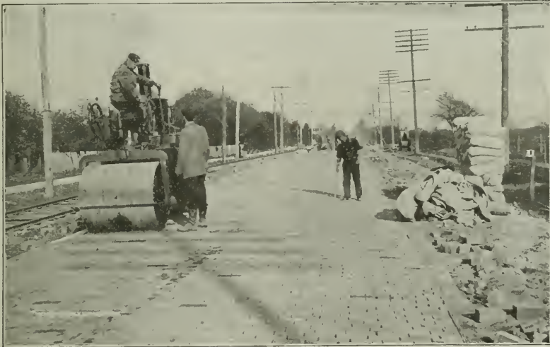
THE BUFFALO-WILLIAMSVILLE ROAD. Rolling—Preliminary to Applying the Grout.
