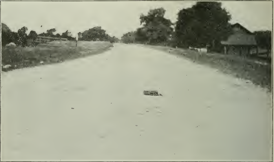
SECTION XV. LIMESTONE CONCRETE. Ohio State Experimental Road.
