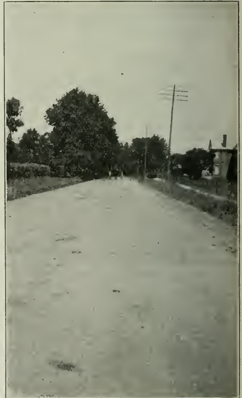
SECTION II STANDARD ASPHALT BINDER. Ohio State Experimental Road.
