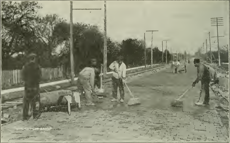
THE BUFFALO-WILLIAMSVILLE ROAD. Applying the Grout According to the N. B. M. A. Specifications.
