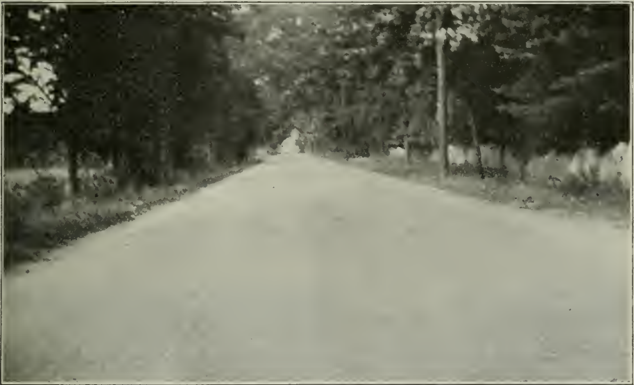
BARRINGTON, R. I., EXPERIMENTAL ROAD II. U. G. I. Road Compound No. 4.
