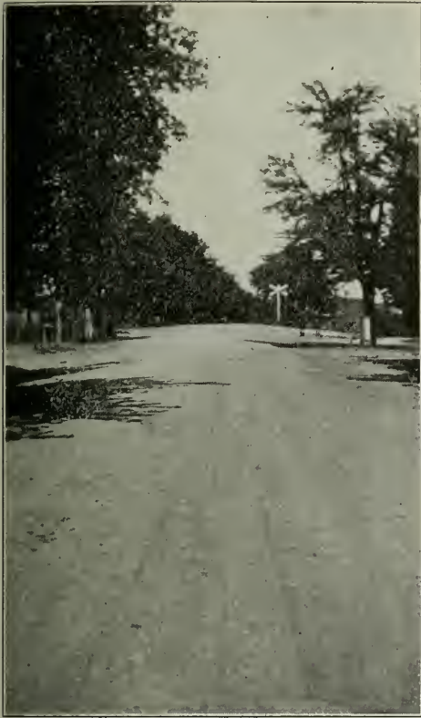
SECTION III. PIONEER ASPHALT BINDER. Ohio State Experimental Road.
