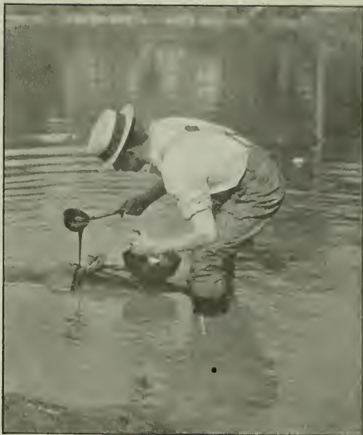
1. POURING G-K COMPOUND IN WATER COVERED JOINT.
