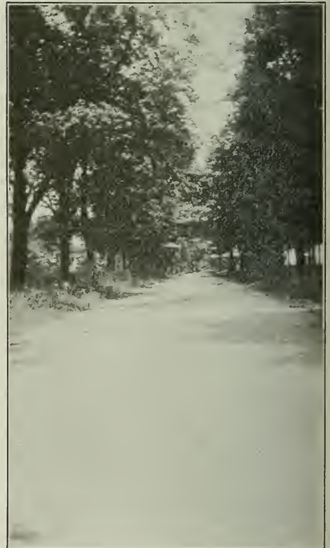
SECTION VI. LIQUID ASPHALT BINDER. Ohio State Experimental Road.
