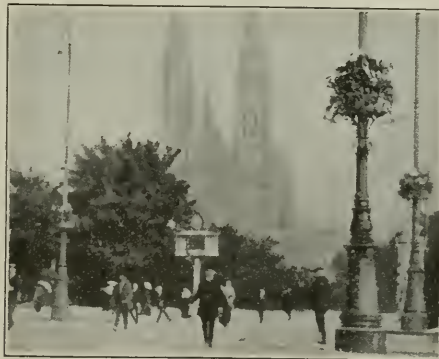
7. ORNAMENTED TRAMWAY POLES, VIENNA.
