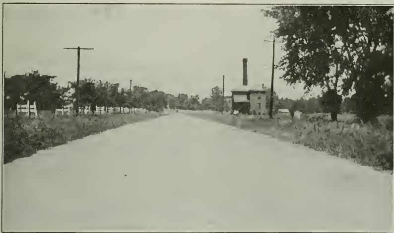
SECTION XI. CARBO-VIA BINDER. Ohio State Experimental Road.
