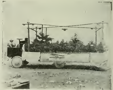
STANDARDS FOR ORNAMENTAL LIGHTS IN WARREN, OHIO.
