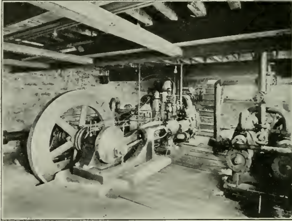
LOVELAND WATER WORKS, ELECTRIC LIGHT AND ICE PLANT. 3. Pumping Engines.
