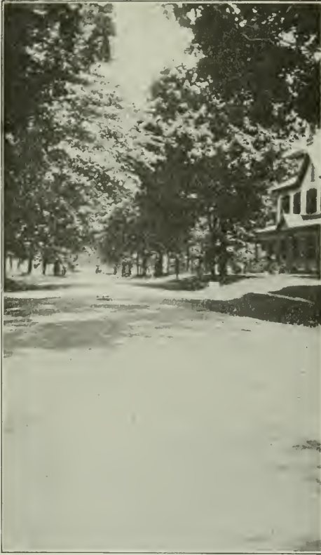
SECTION V. TARVIA "B" SURFACE TREATMENT Ohio State Experimental Road.
