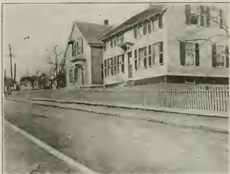
HARVEY STREET, PAWTUCKET, R. I. Bitulithic Pavement on 4.9 per cent. Grade.
