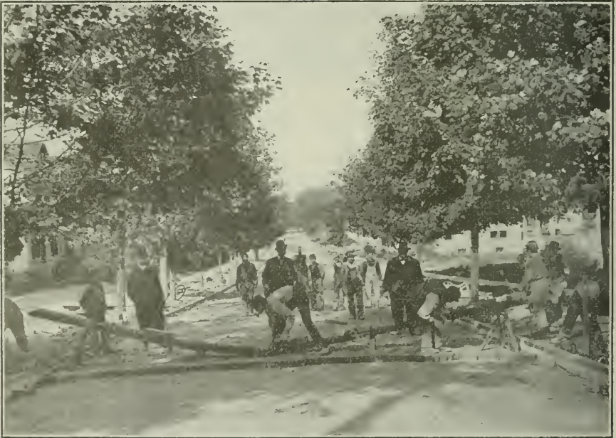
LAYING PAVING BRICK. SHOWING METHOD OF USING MATHEWS GRAVITY CARRIER.
