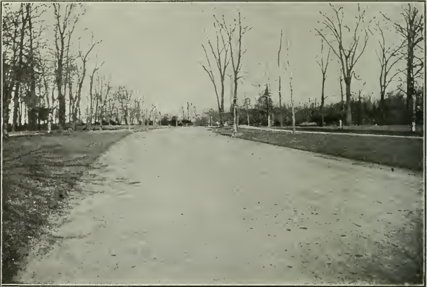
ROAD IN EDGEWATER PARK, CLEVELAND, TREATED WITH TARVIA A.
