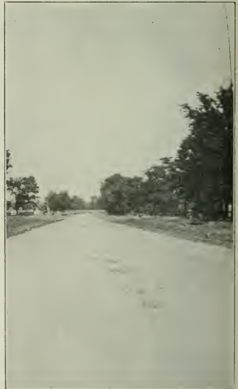
SECTION XIII. TAROID BINDER. Ohio State Experimental Road.
