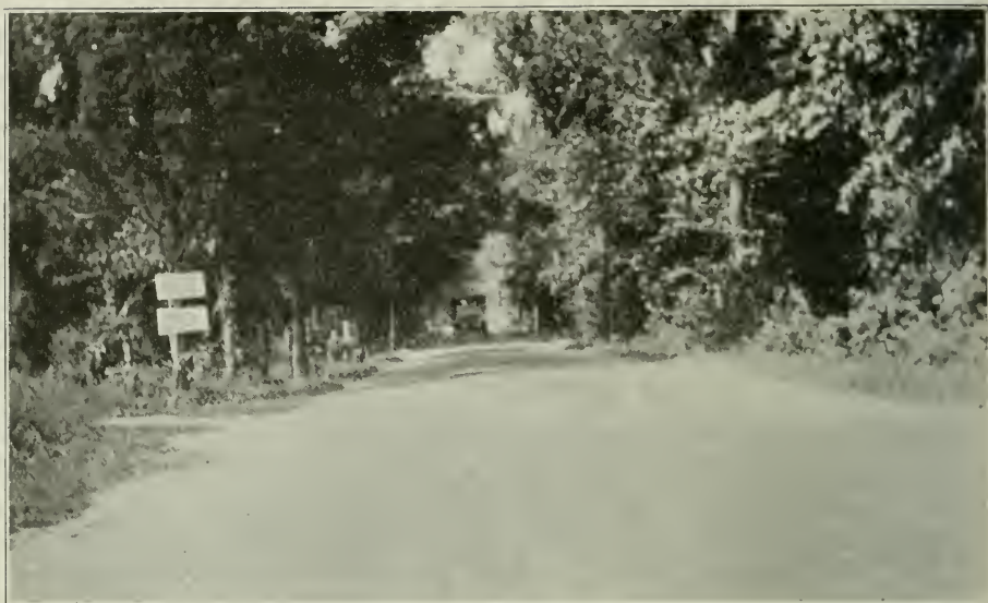
BARRINGTON, R. I., EXPERIMENTAL ROAD. V. Texaco Macadam Binder.
