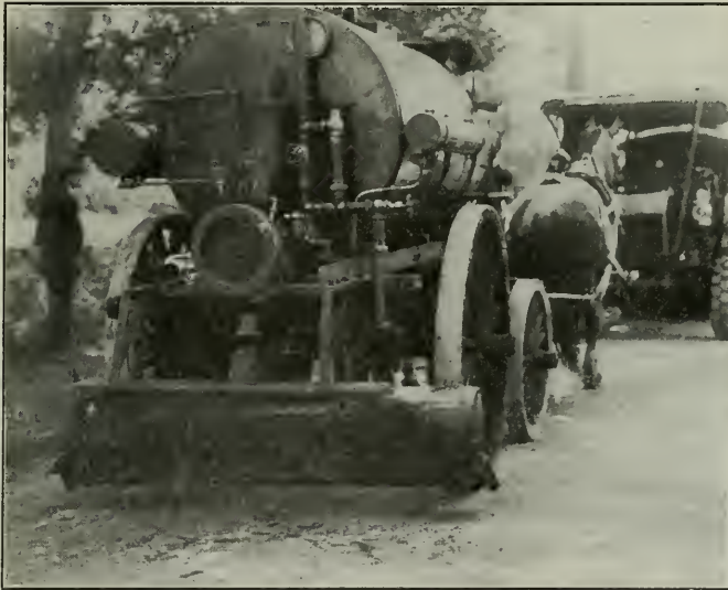
VII. BITUMINOUS ROAD CONSTRUCTION MACHINERY. Gasoline Engine Distributer of Standard Oil Co.
