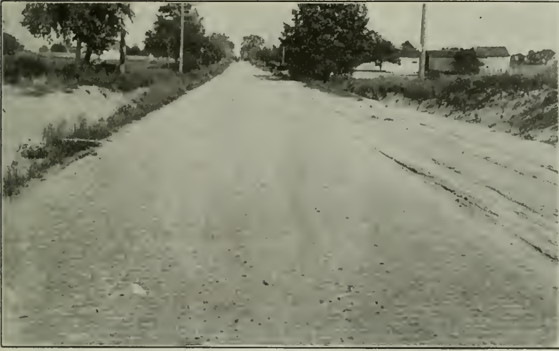
DURHAM ROAD, CUYAHOGA COUNTY, OHIO. Laid Five Years Ago on a Concrete Base.
