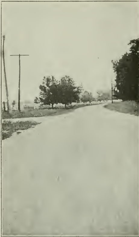
SECTION XII. CONCRETE MACADAM. Ohio State Experimental Road.
