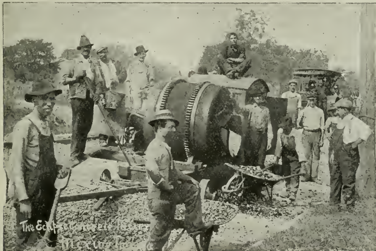
MIXING BITUMINOUS CONCRETE WITH AN "ECLIPSE" MIXER.
