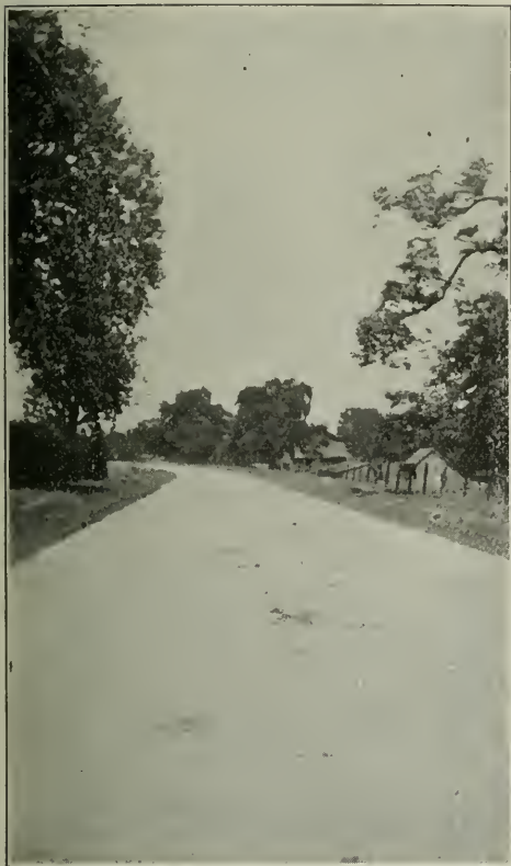
SECTION XVI. GRAVEL CONCRETE. Ohio State Experimental Road.
