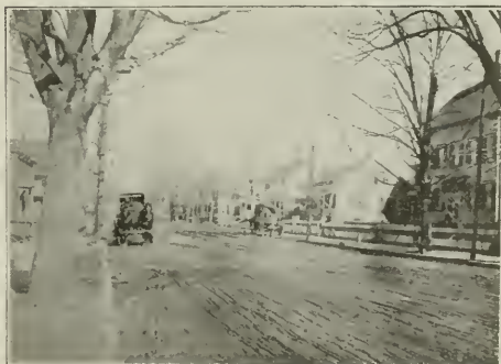
BROADWAY, PAWTUCKET R. I. Macadam Street with Short Section of Bitulithic.
