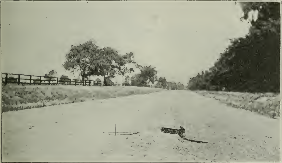
SECTION XIV. PETROLITHIC PAVEMENT. Ohio State Experimental Road.
