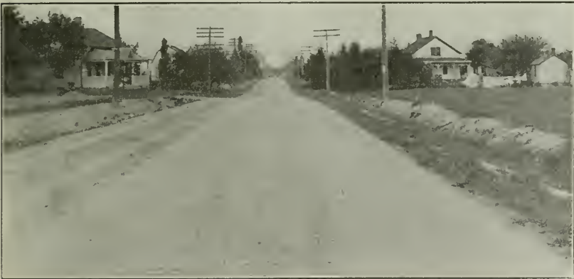
NORTH RIDGE ROAD, CUYAHOGA COUNTY, OHIO. Laid Five Years Ago on a Broken Stone Base.
