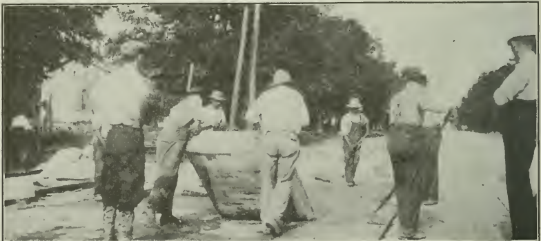
MAIN STREET ROAD, BUFFALO, N. Y. Applying Grout by the Incorrect Dumping Method.
