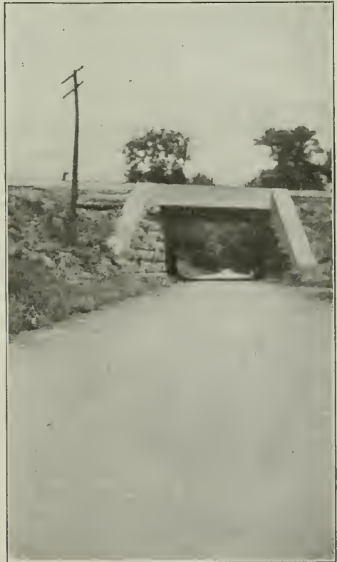
SECTION VIII. FAIRFIELD ASPHALTIC CEMENT Ohio State Experimental Road.
