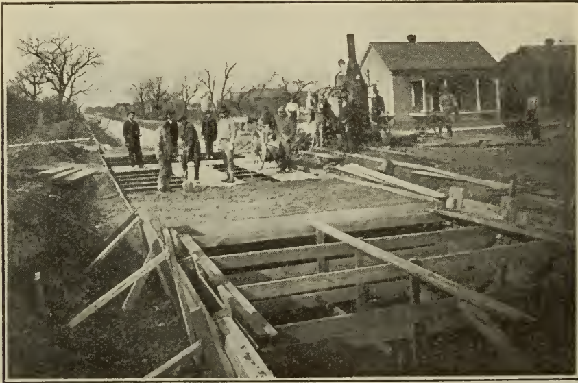
ROOFING PORTION OF STORM WATER CONDUIT, LAWTON, OKLA.
