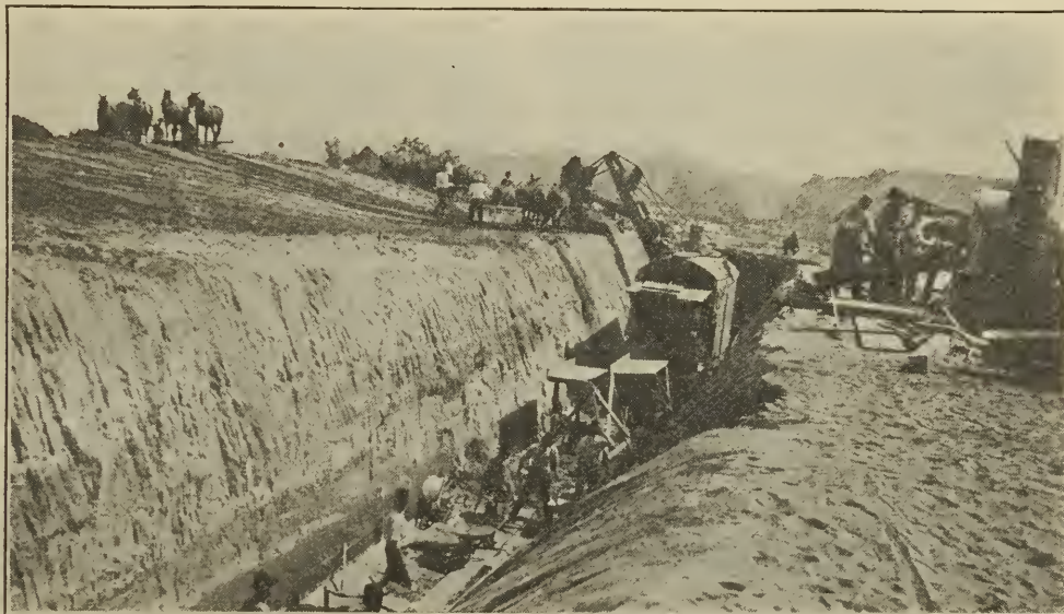
THE LOS ANGELES WATER WORKS. Trenching for the New Eight-Foot Conduit.
