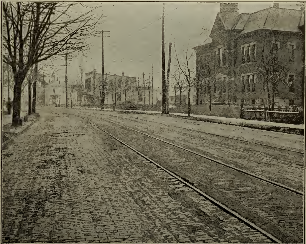
MAIN STREET, SOUTH OF THORNTON STREET, AKRON, O. Fifteen Years Old. Cement Filler
