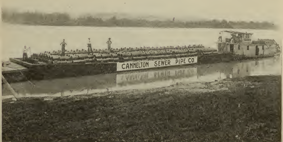
SHIPMENT OF CANNELTON SEWER PIPE ON THE OHIO RIVER.
