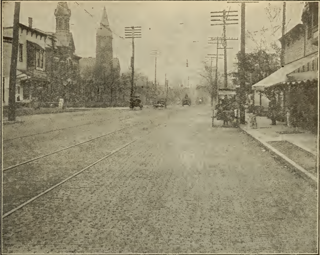
MAIN STREET, NORTH OF THORNTON STREET, AKRON. O. Twenty Years Old. Pitch Filler
