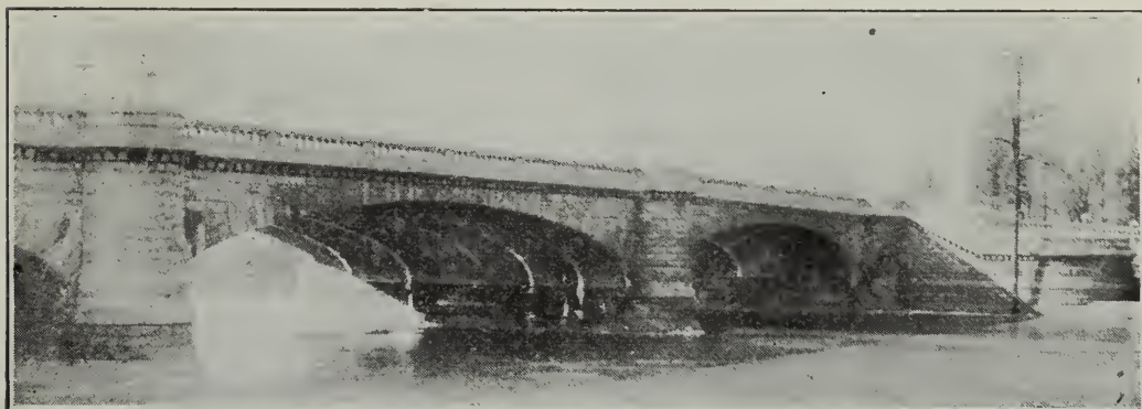
VI. THIRTIETH STREET BRIDGE, INDIANAPOLIS, IND.
