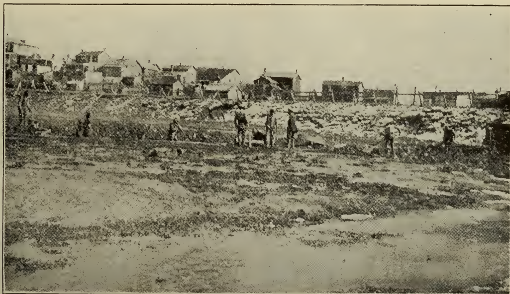
LAYING WATER TIGHT SEWER IN SWAMP AT HARRISBURG, PA. (See page 352).
