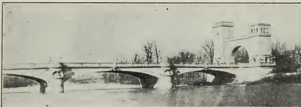
V. EMRICHSVILLE BRIDGE, INDIANAPOLIS, IND.
