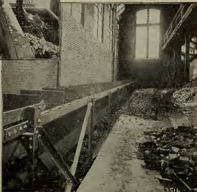
III. INTERIOR OF GREEN GAR- BAGE PLANT, WHERE THE GARBAGE IS SORTED AND SHOVELED INTO CON- VEYOR.
