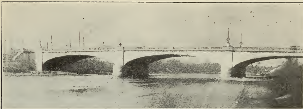
IV. WEST MICHIGAN STREET BRIDGE, INDIANAPOLIS, IND.
