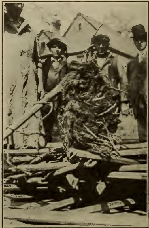
ROOTS REMOVED FROM CLEVELAND SEWERS BY SIEBEN MACHINE.
