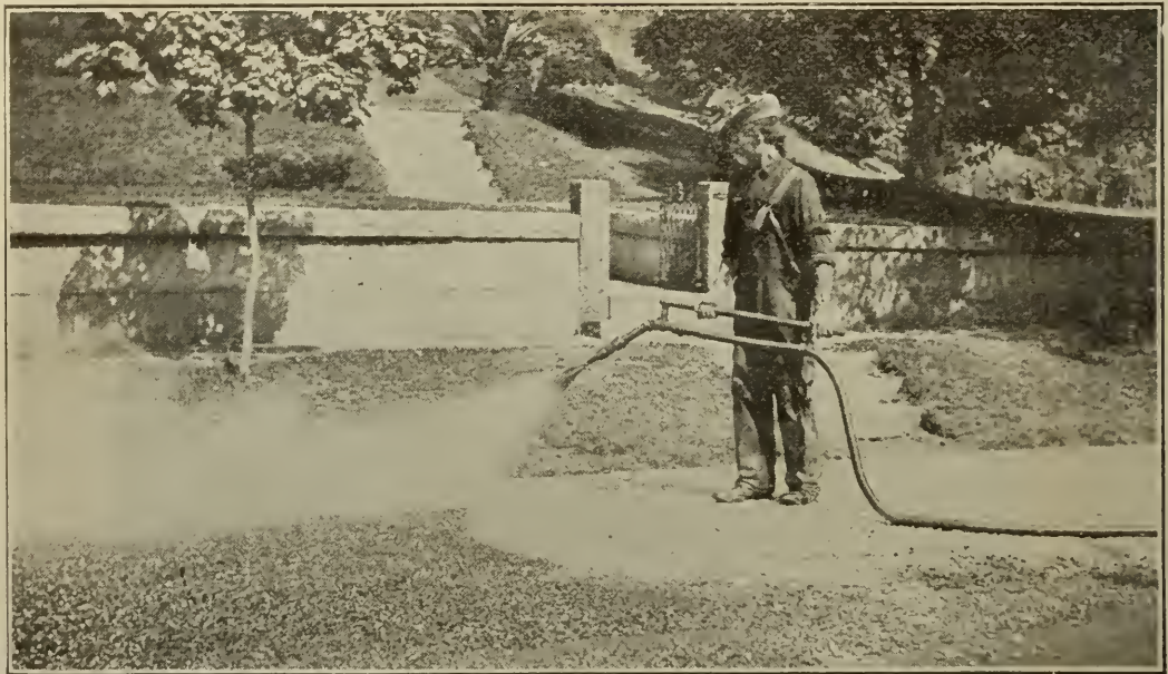
SPRAYING TARVIA X ON THE BROKEN STONE AS A BINDER.
