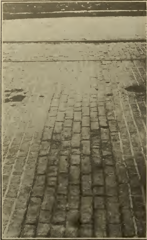
9. STATE STREET, CONNEAUT, O. Cement filled brick street laid in 1904 on gravel foundation, with six joints poured with pitch filler every 40 feet.
