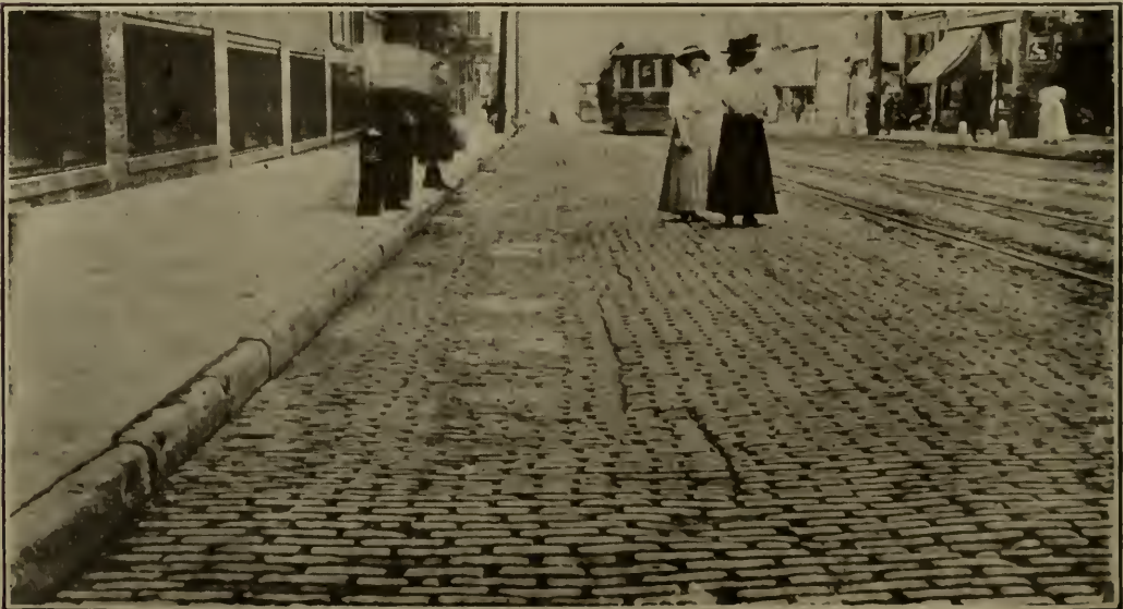
2. MAIN STREET, AKRON, O. Opposite No. 497. Breaks in Pitch Filled Pavement.
