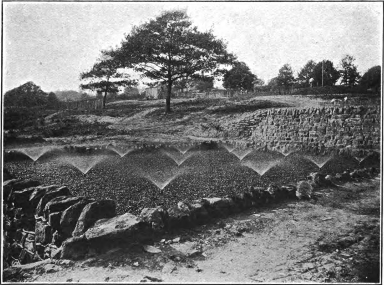
Fig. 49.—Fixed Sprinklers in Operation at Tunbridge Wells.
