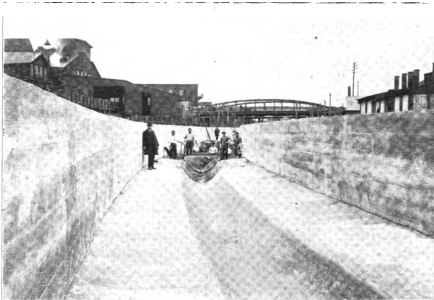
Large Concrete Sewer in Aramingo Canal.
